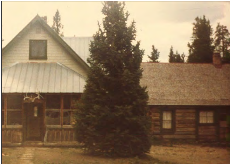
Figure 20. North-facing sides of Main House and Cabin (Buildings 2 and 3), 1980
