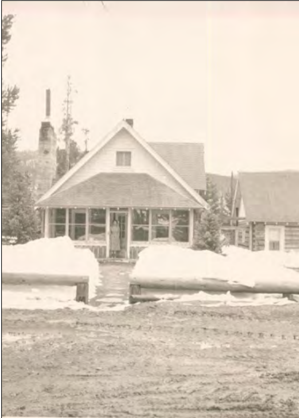
Figure 16. Henry Jones' wife on the north façade of Main House. April 1960
