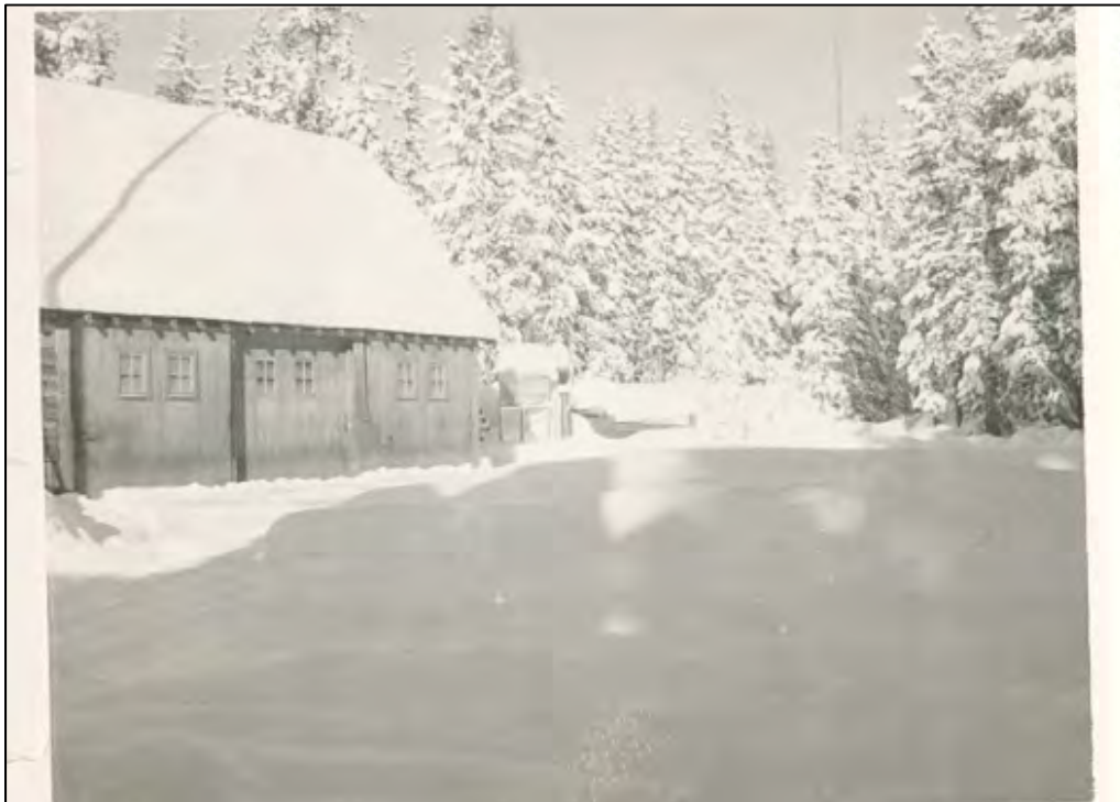
Figure 18. CCC Garage/Office (Building 1) – part of east (main) façade, camera facing northwest. January 1962
