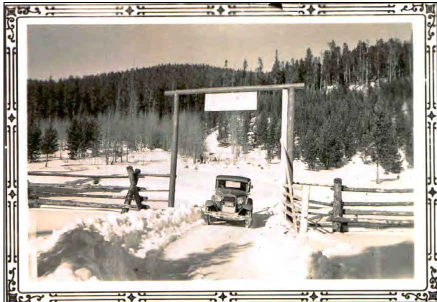
Figure 4. Original entrance to the Building Complex (Resource 10), camera facing southwest, ca. 1930s.
