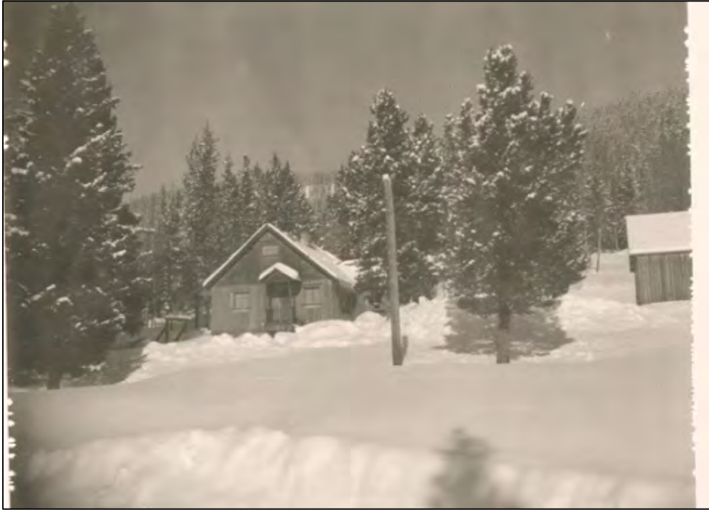
Figure 14. South façade Crew Cabin (Building 8) and Barn/Garage (Building 9), camera facing north, ca. 1940-50s
