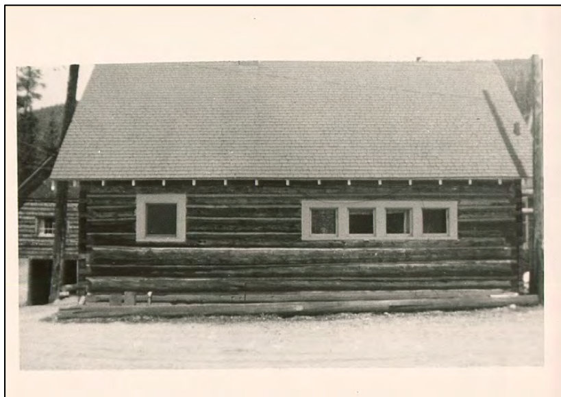
Figure 13. South Façade of Cabin (Building 2), camera facing north, ca. 1940-50s
