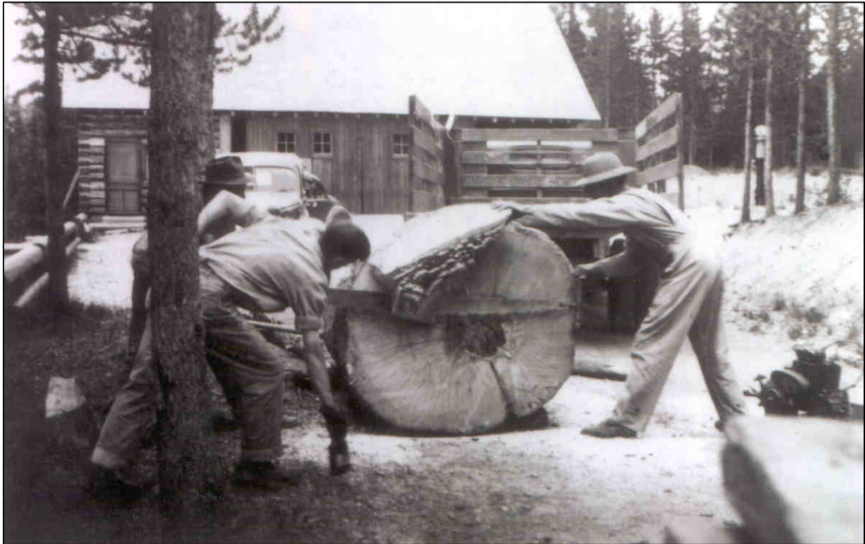
Figure 11. POWs working at the Building Complex, in front (east) of Office/ (Building 1), making picnic tables, camera facing west, ca. 1944.
