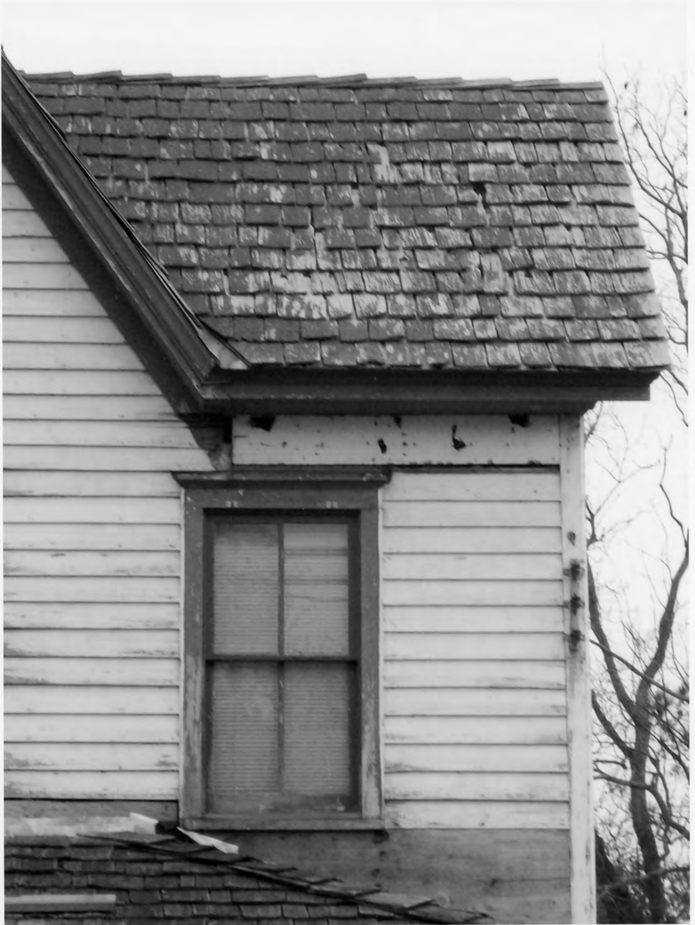
Tunnell - West House_Sussex County_DE detailed view of second story west facade window, clapboards, cornice, and plain frieze
