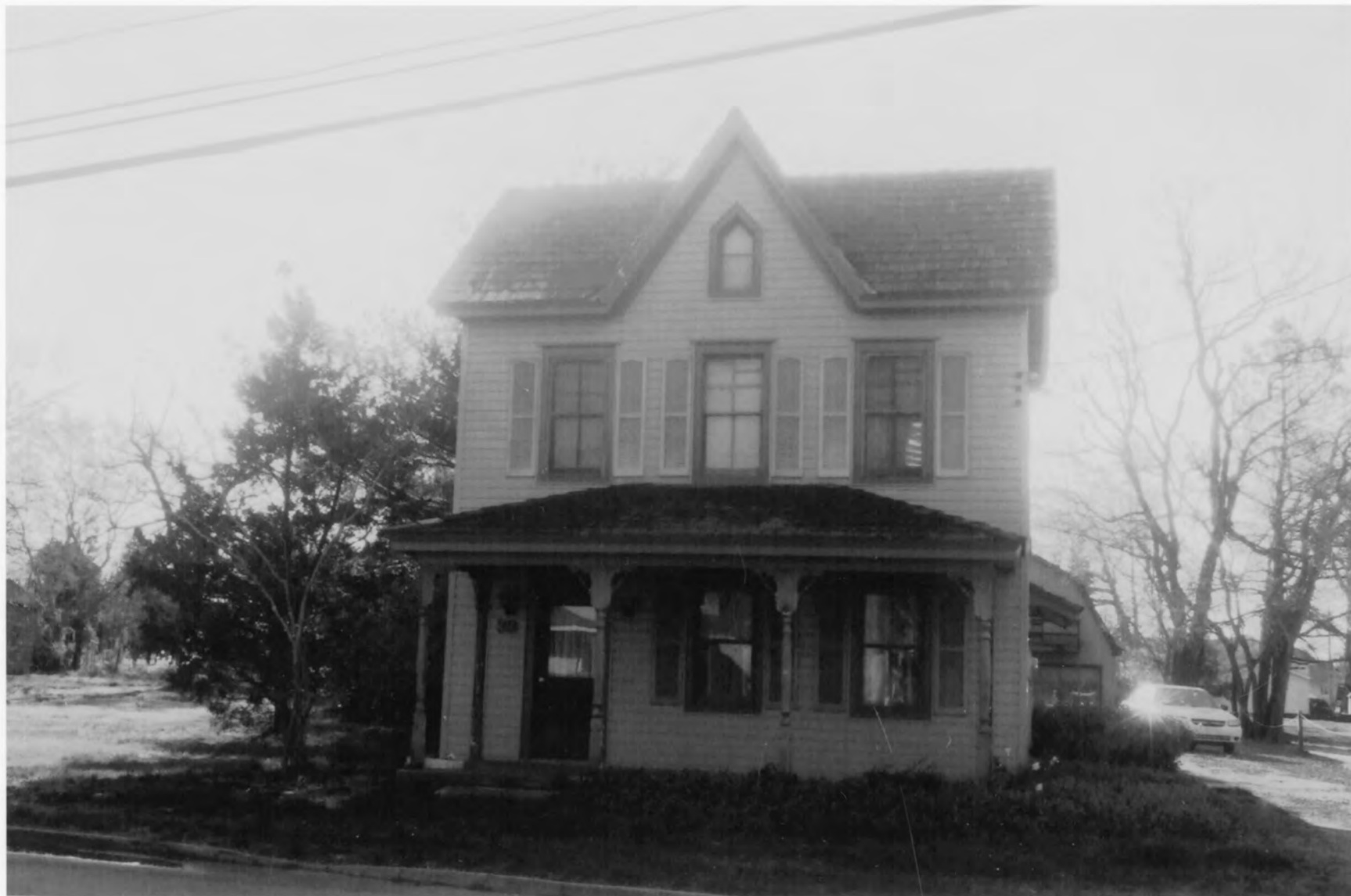
Tunnell - West House_Sussex County_DE west facade fronting Central Avenue
