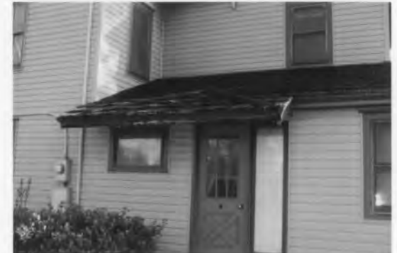
South side of house with enclosed side porch
