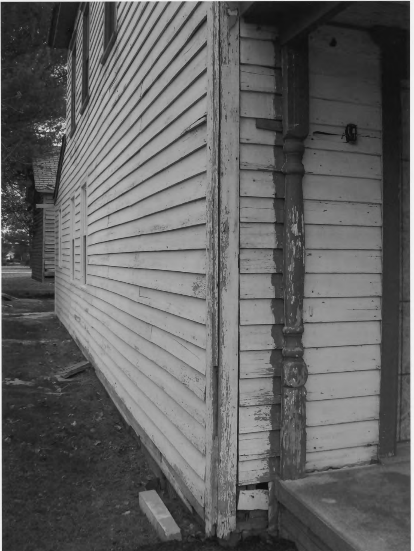
Tunnell - West House_Sussex County_DE detail of northwest corner of house showing original clapboards, beaded corner trim, and the attached turned, split-column on clapboards
