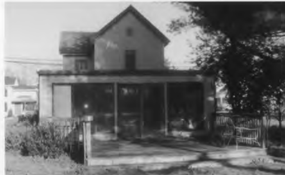
East side of house before the recently constructed addition was removed
