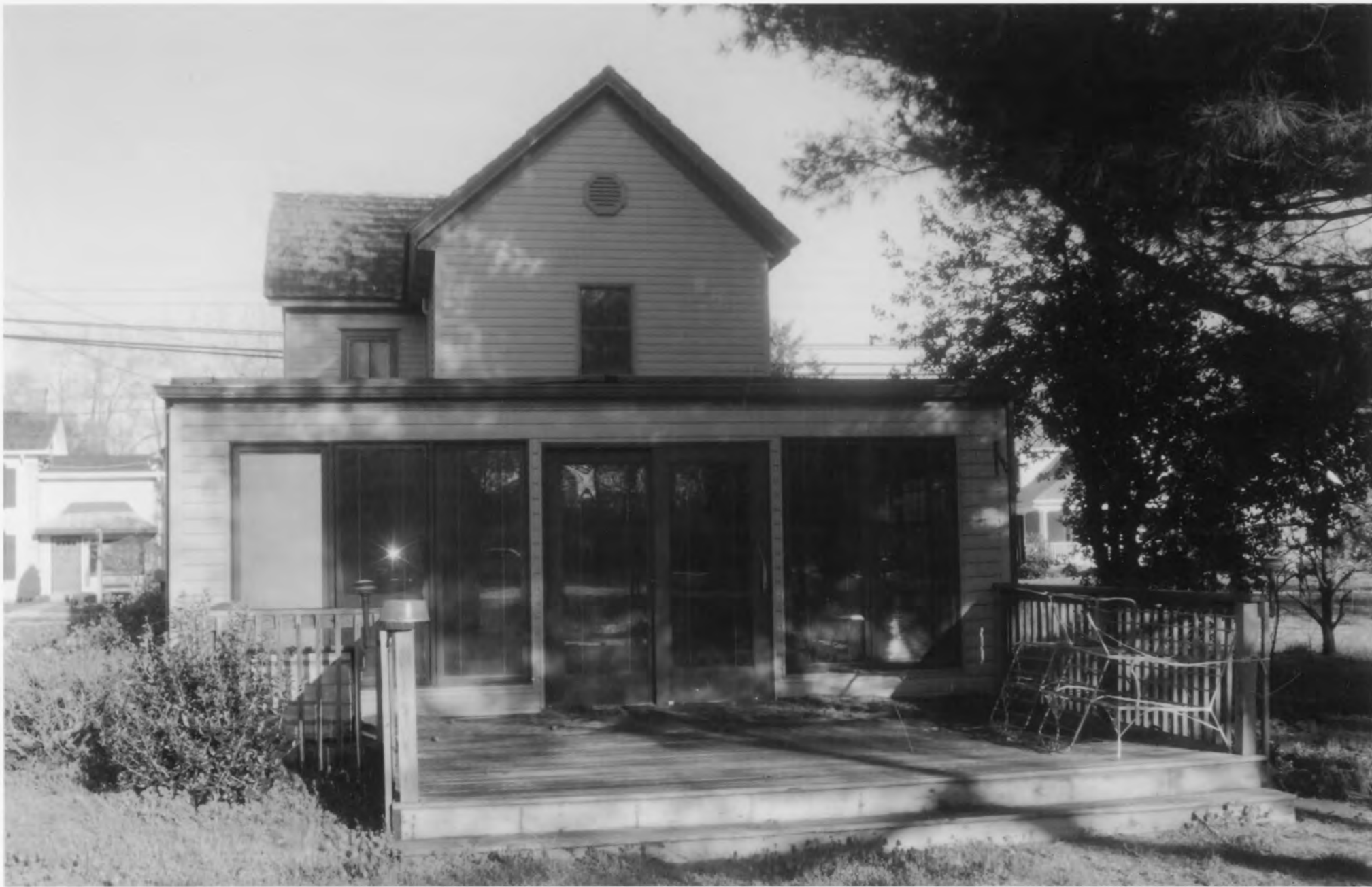
Tunnell - West House_Sussex County_DE east elevation with recently constructed deck and one-story addition
