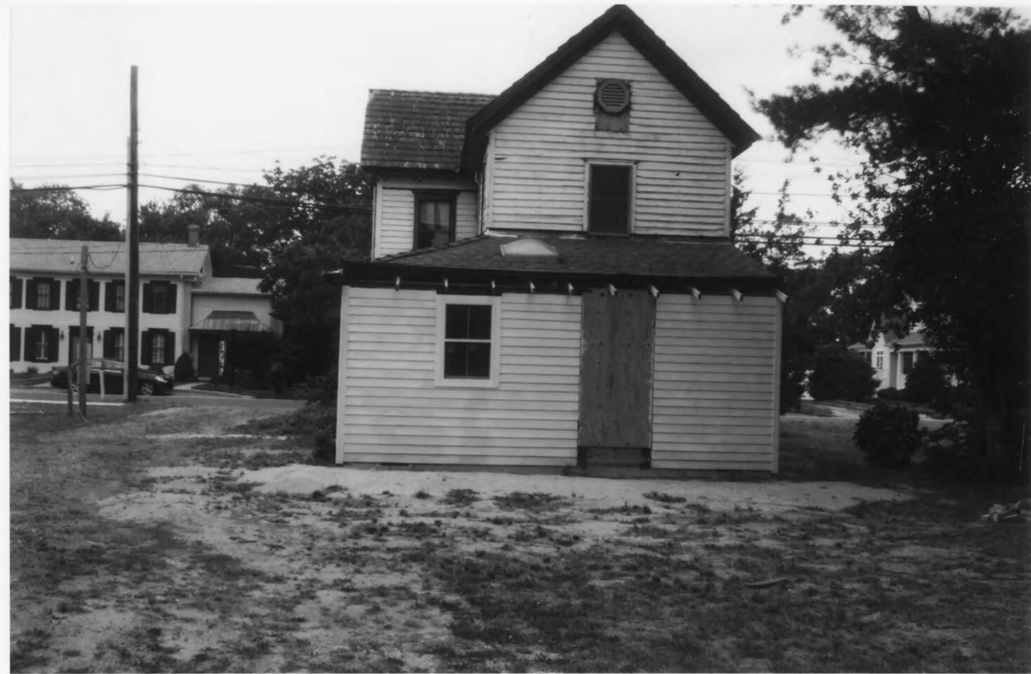
Tunnell - West House_Sussex County_DE east elevation showing restored wall of late-nineteenth century wrap-around addition
