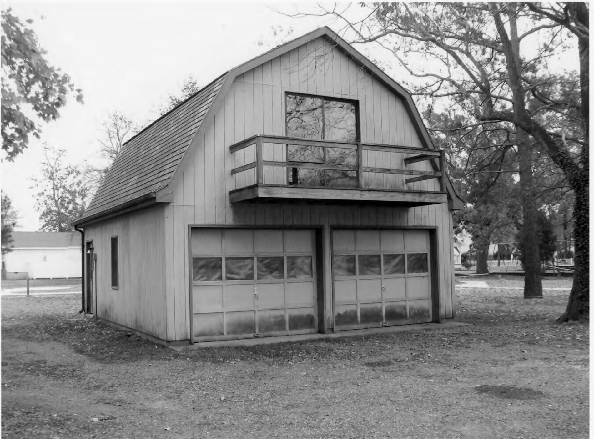
Tunnell - West House_Sussex County_DE recently constructed two-story, two-bay, frame, garage with gambrel roof
