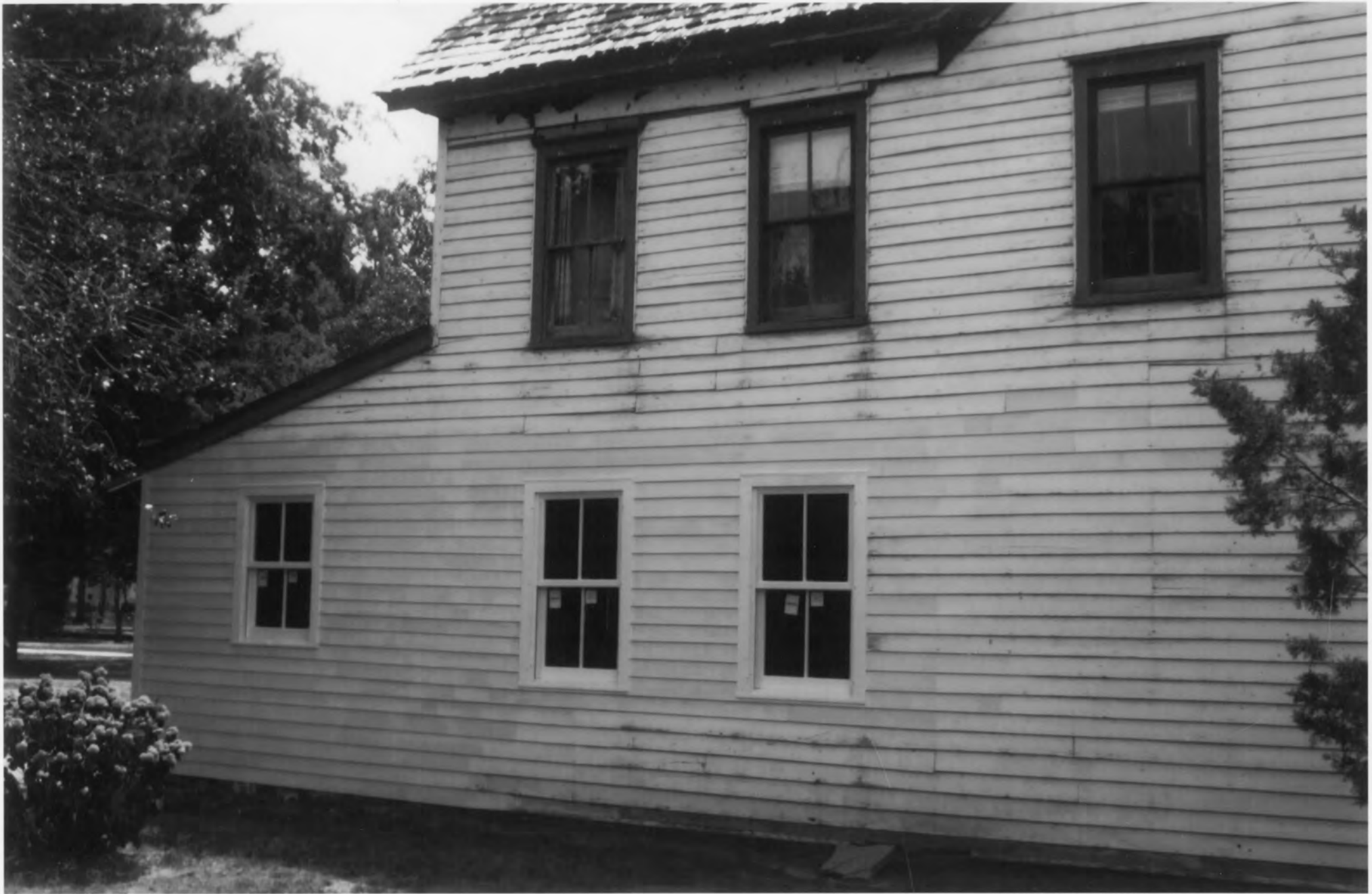
Tunnell - West House_Sussex County_DE north elevation with restored two-over-two, double-hung windows
