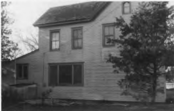
North side of residence with modern first floor windows
