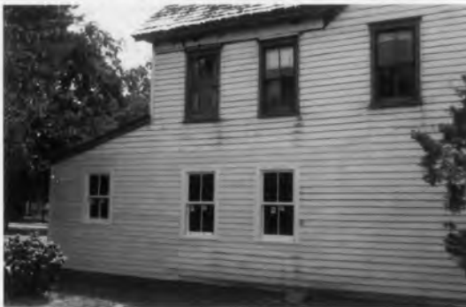
North side of house with restored windows and clapboards
