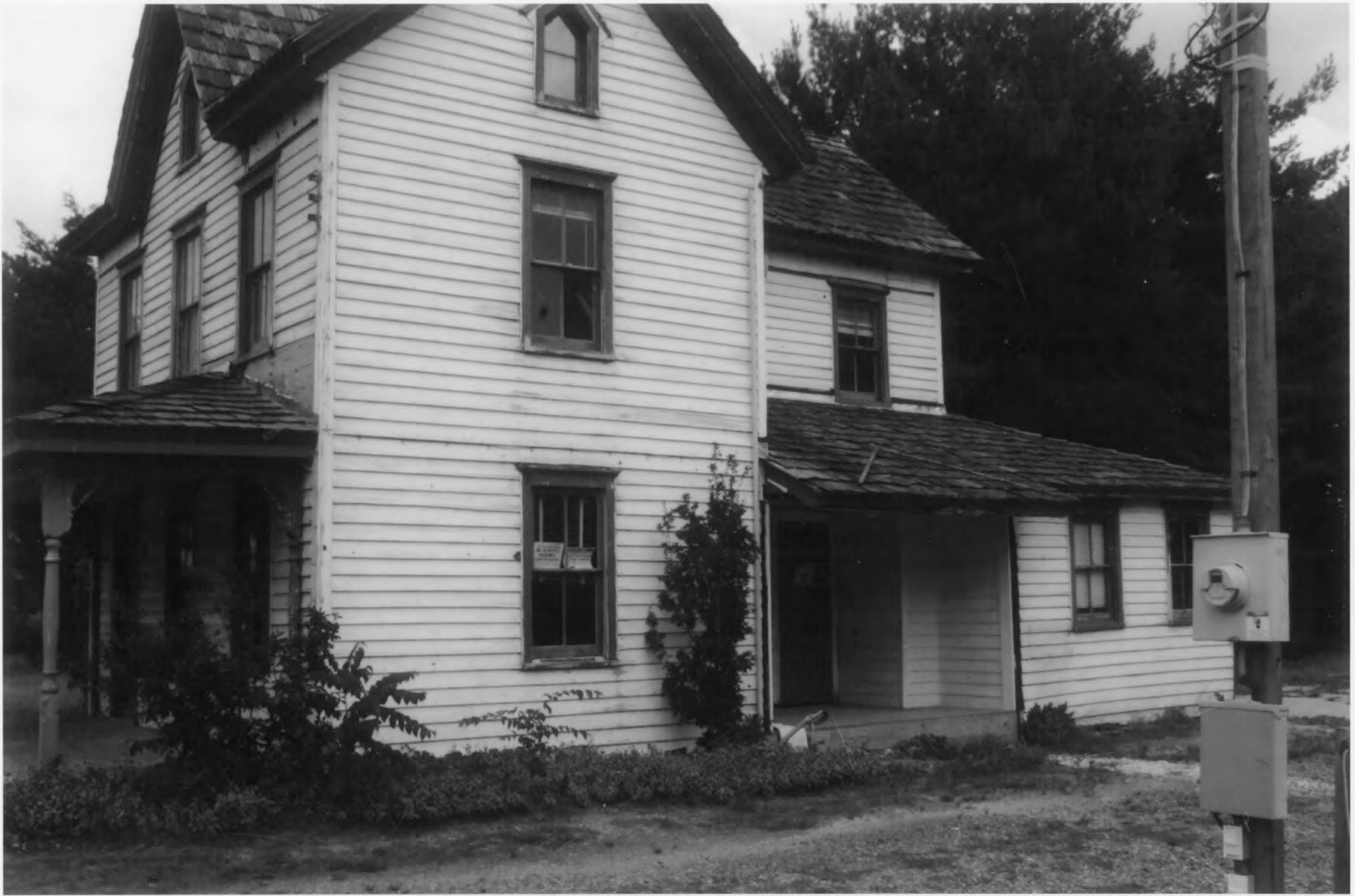
Tunnell - West House_Sussex County_DE south elevation showing opened side porch area
