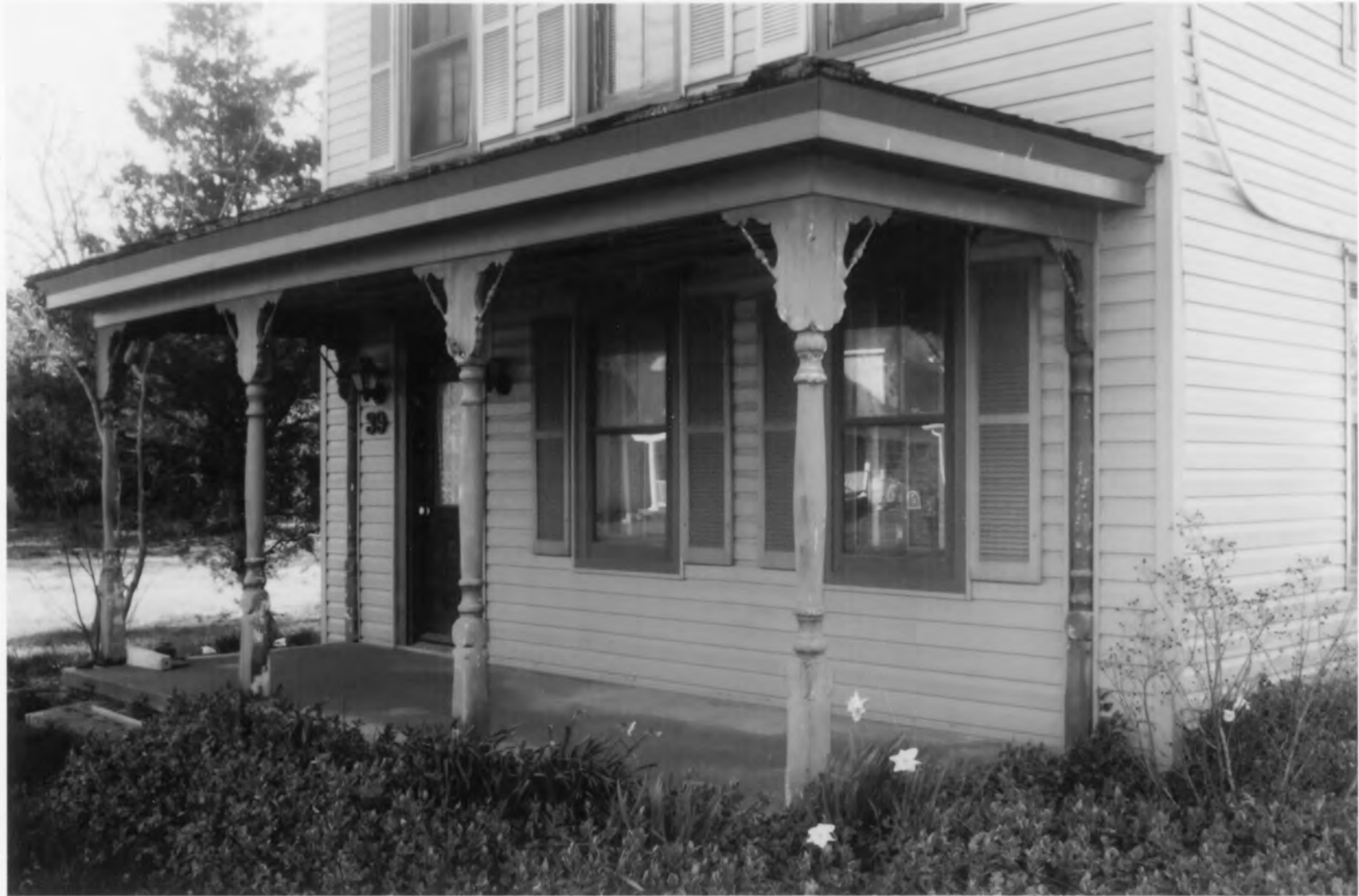
Tunnell - West House_Sussex County_DE three-quarter view of west facade, original porch columns with decorative capitals and corner braces
