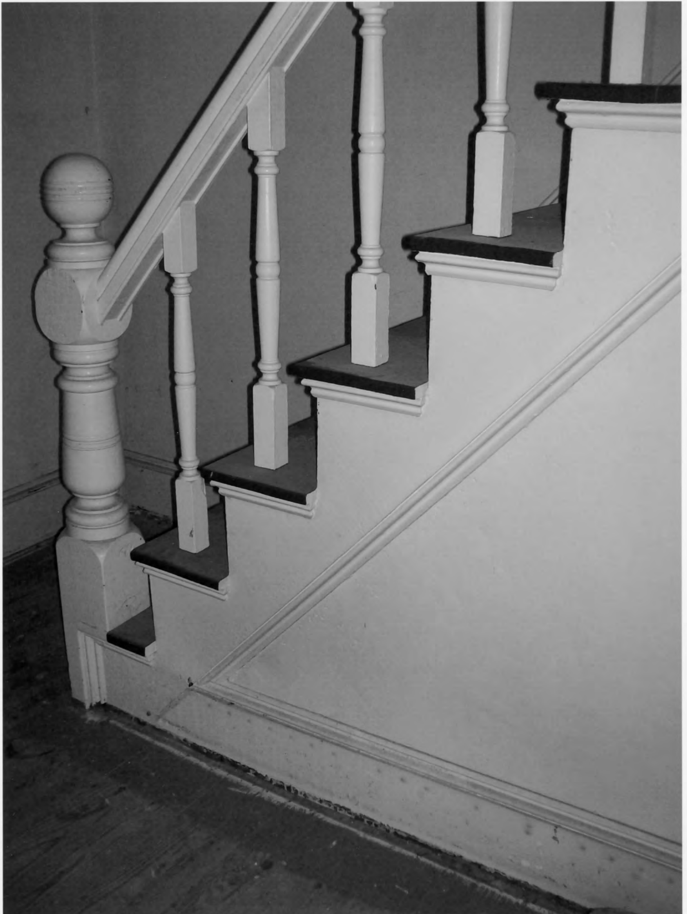
Tunnell - West House_Sussex County_DE side hall open-string staircase with original turned newel post, turned balusters, moulded handrail, baseboard trim, and pine flooring
