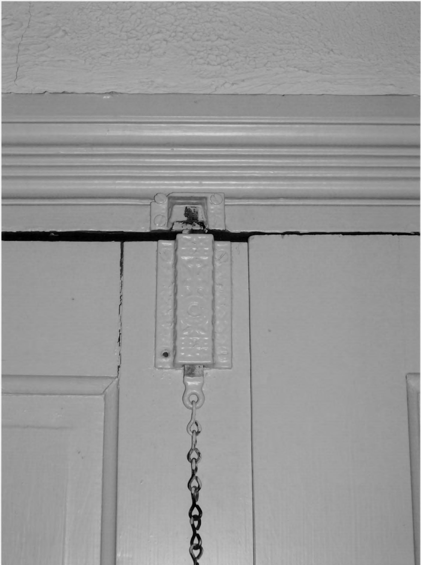
Tunnell - West House_Sussex County_DE parlor door detail of electroplated door lock with pull chain
