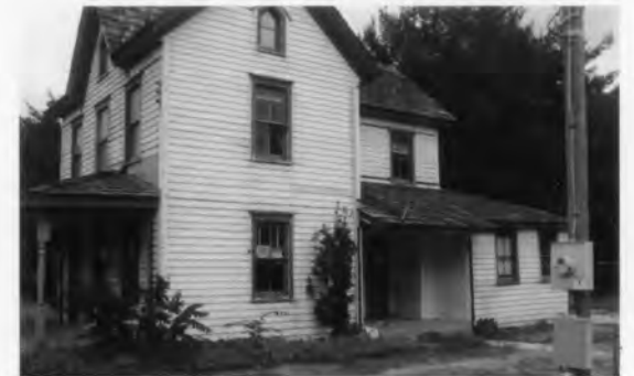
South side of house with porch enclosure removed
