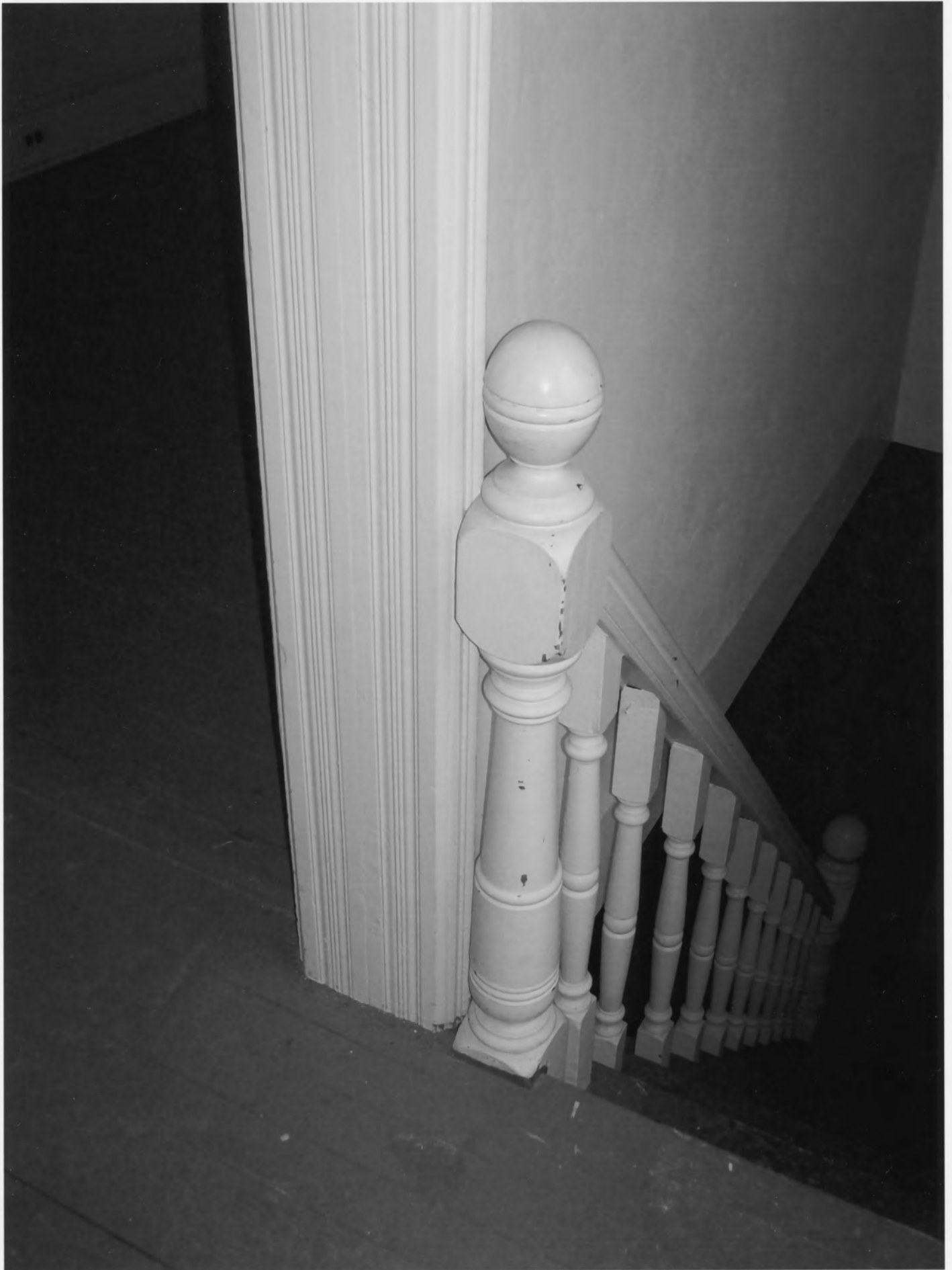
Tunnell - West House_Sussex County_DE second floor view of staircase showing large turned newel post, turned balusters, original flooring, and moulded door surround trim
