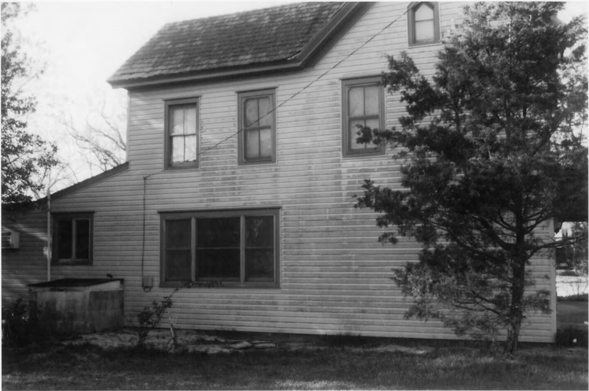
Tunnell - West House_Sussex County_DE north elevation with modern, three-section window and vinyl siding
