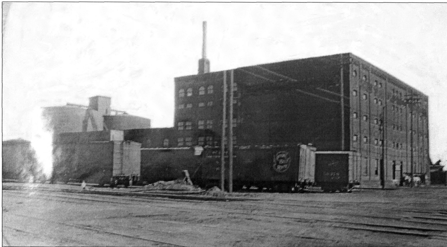
Figure 46: The former (?) oil mill as home for Chapman Transfer and Storage, 1923, note how the linseed oil company signage has been covered over, note also the metal chimney extension ( Three Quarters of a Century of Progress )
