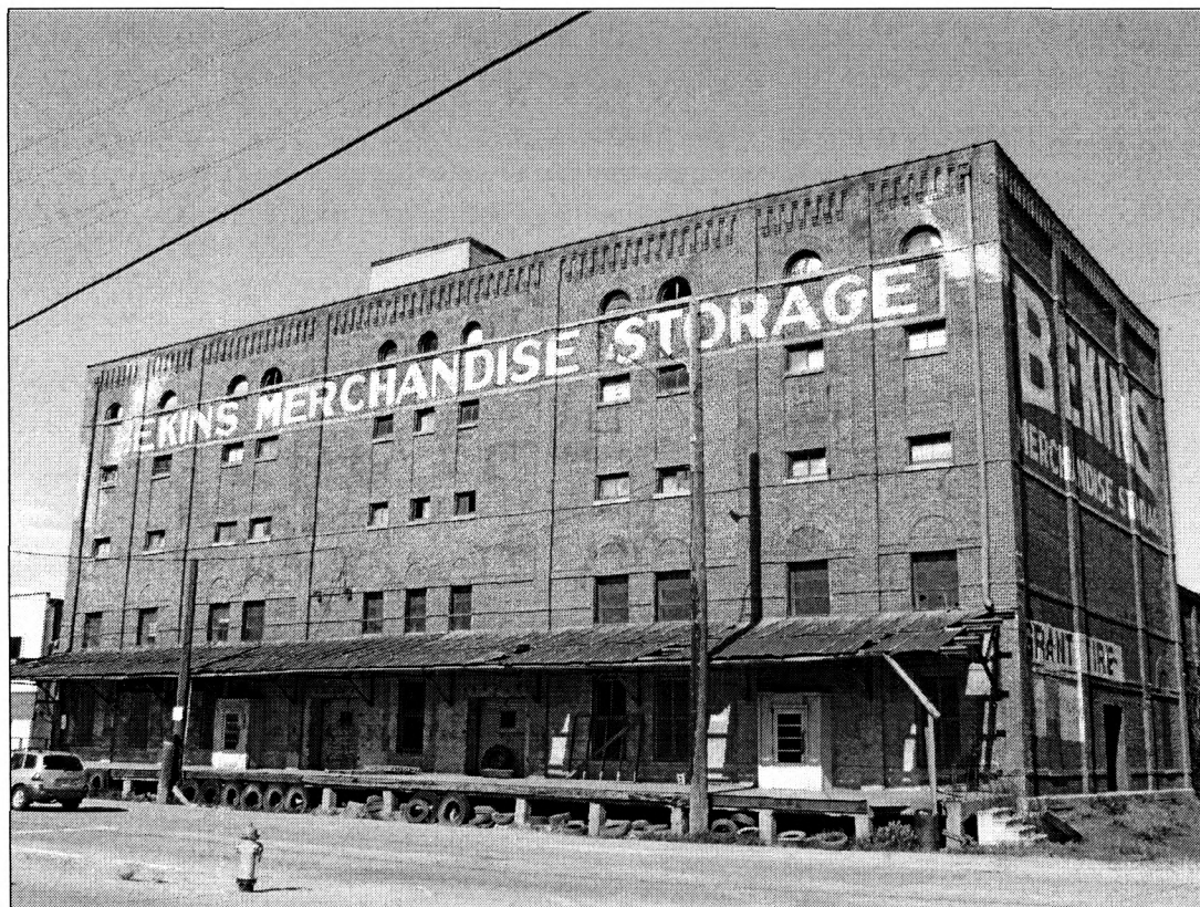
Figure 2: Façade overview, view northeast (photo by J. Jacobsen, 2007)
