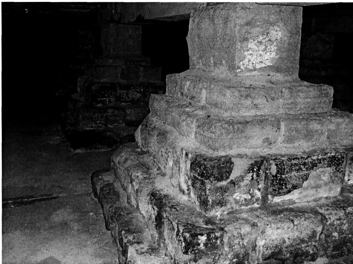
Figure 3: above-grade spread-stone footings, view southwest (photo by J. Jacobsen, May 2007)
