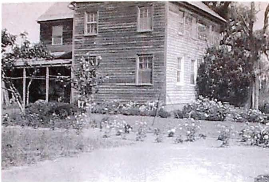
Figure 6: ca. 1950 photograph of the house before the asbestos siding was added and showing the south side of the house with the ca. 1920 open air porch. [photo courtesy of Isabelle Foster Sakewicz]
