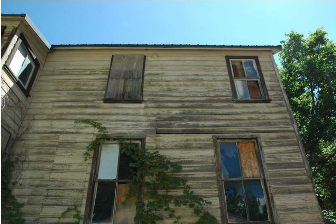
Photograph 5 West elevation of Reddick Hotel, south half. Camera facing east.
