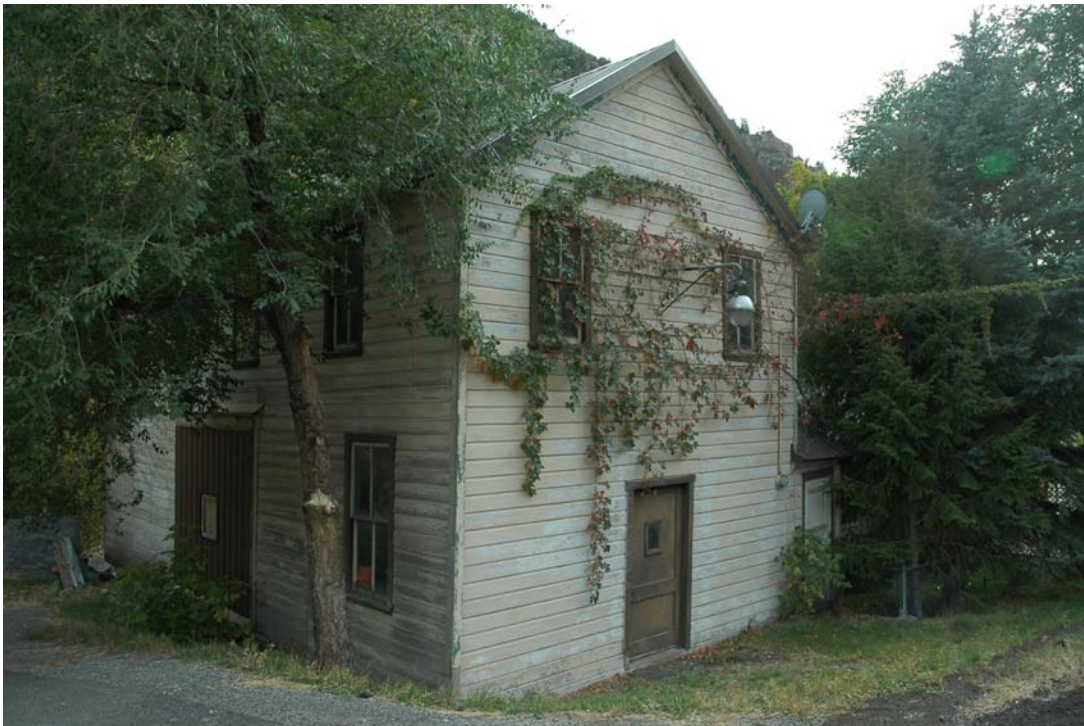
Photograph 2 North and east elevations of Reddick Hotel. Camera facing southwest.
