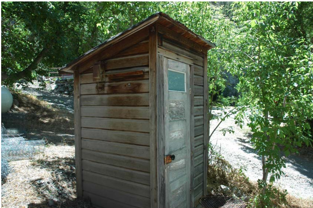
Photograph 12 Outhouse/shed for television equipment. Camera facing southeast.
