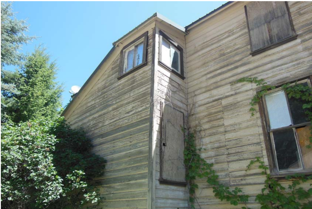
Photograph 6 West elevation of Reddick Hotel, stairwell structure. Camera facing northeast.
