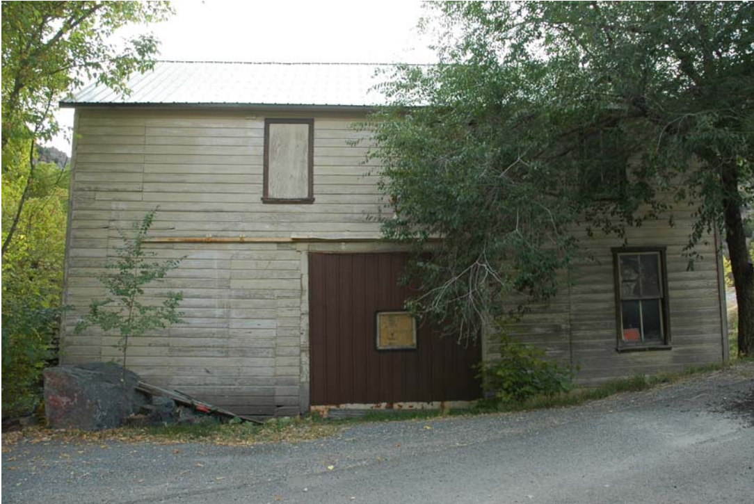
Photograph 3 East elevation of Reddick Hotel. Camera facing west.
