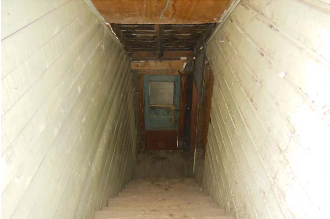
Photograph 11 Interior, stairwell. Camera facing north toward entrance.
