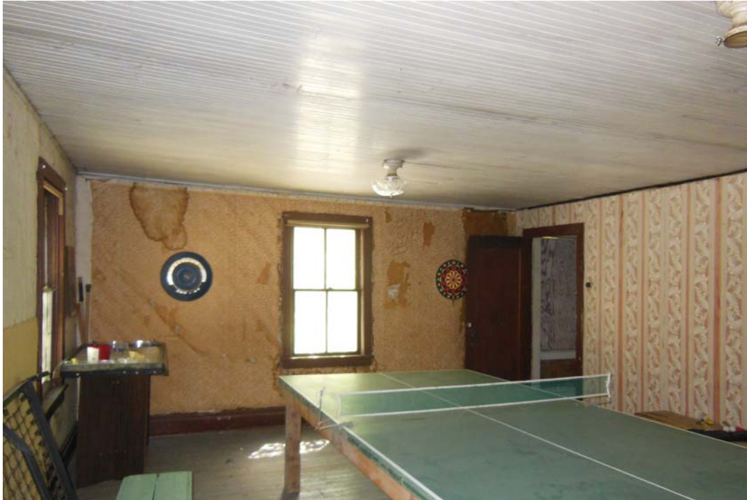
Photograph 9 Interior, second floor north room. Camera facing east.
