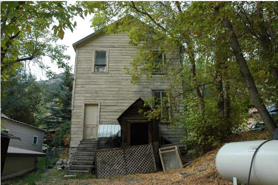
Photograph 4 South elevation of Reddick Hotel. Camera facing north.
