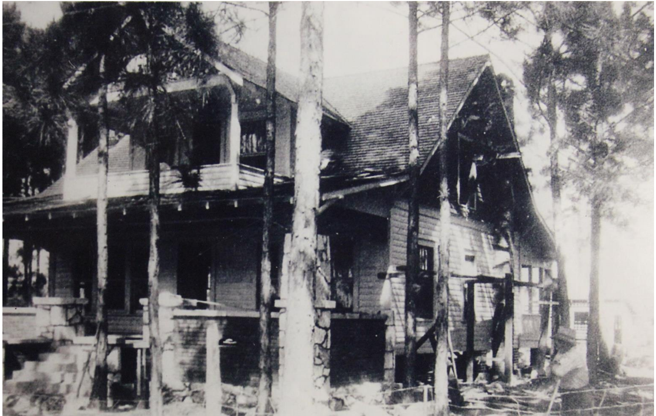
Figure 4: Construction Photo, c. 1917. The original lot, like much of Bunnell, was wooded with pine trees. (Flagler County Historical Society)
