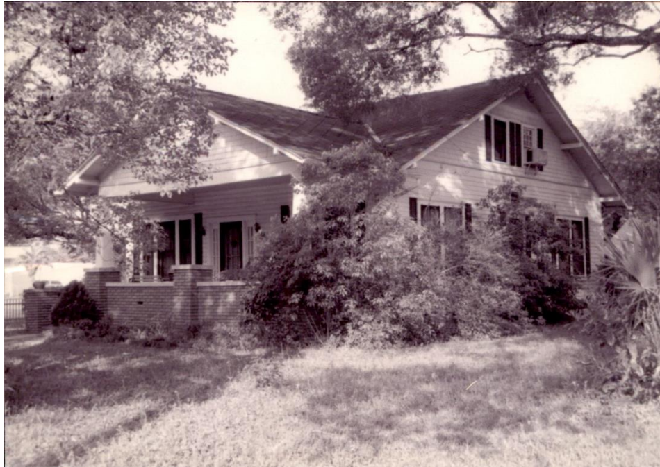
Figure 9: 1998 Survey photo of 400 E Moody Boulevard. The house retains much of its original details, but now has a new red, standing seam metal roof. (Florida Master Site File, FL00107)
