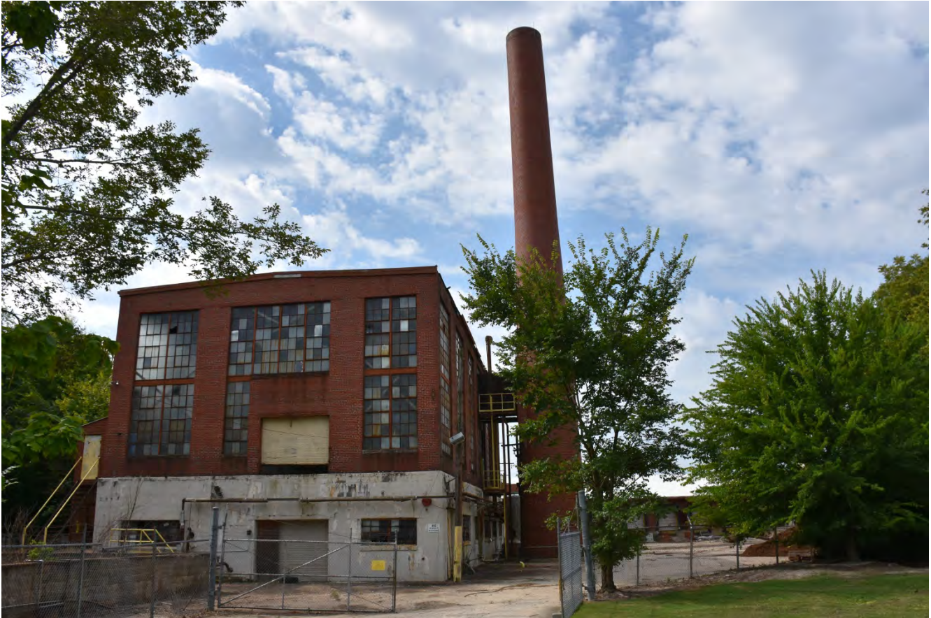
11. 1940/1952 boiler house and 1940 smokestack, north elevation; oil storage tank at left
