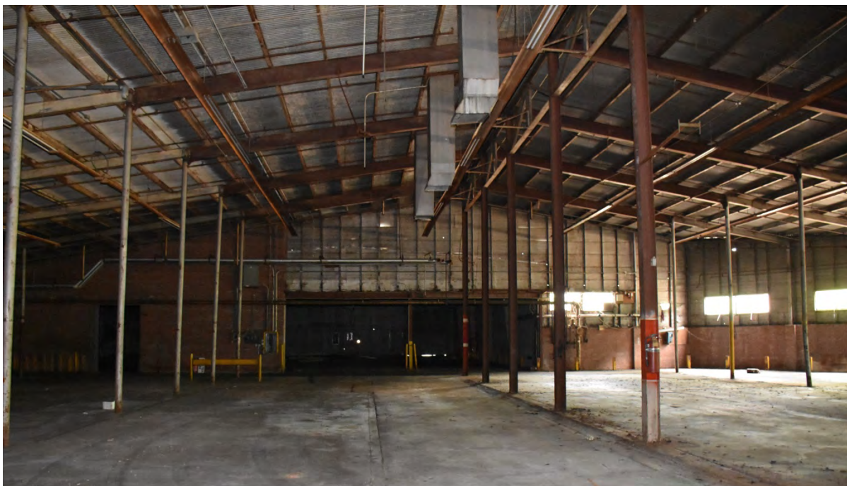
8. 1955 finished product warehouse, west end, looking west into 1977 warehouse (below)
