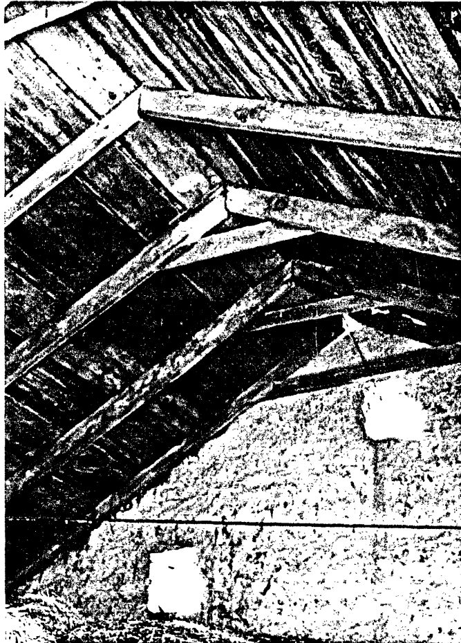
Fig. 2. Interior view of Kass Barn. St. Donatus, Iowa ( Site 44b ) Note lack of Ridge Pole at roof peak
