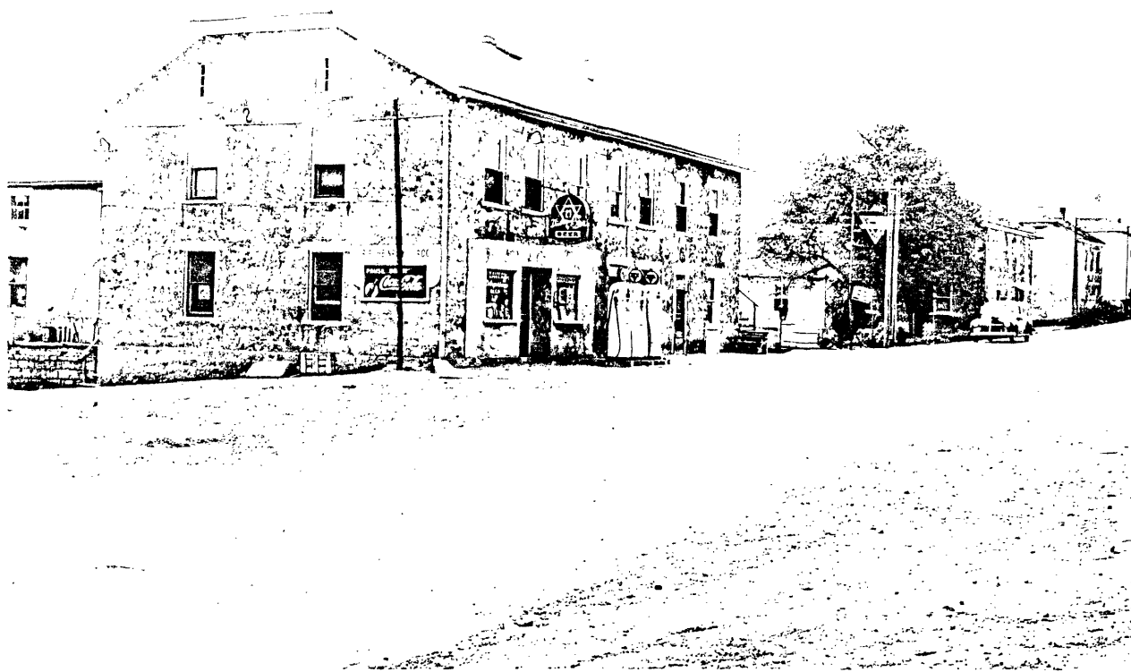
Fig. 9. Intersection of the Dubuque to Bellevue and the Gear's Ferry Roads. Looking North. Sites 13a and 14. ( Date Unknown. )
