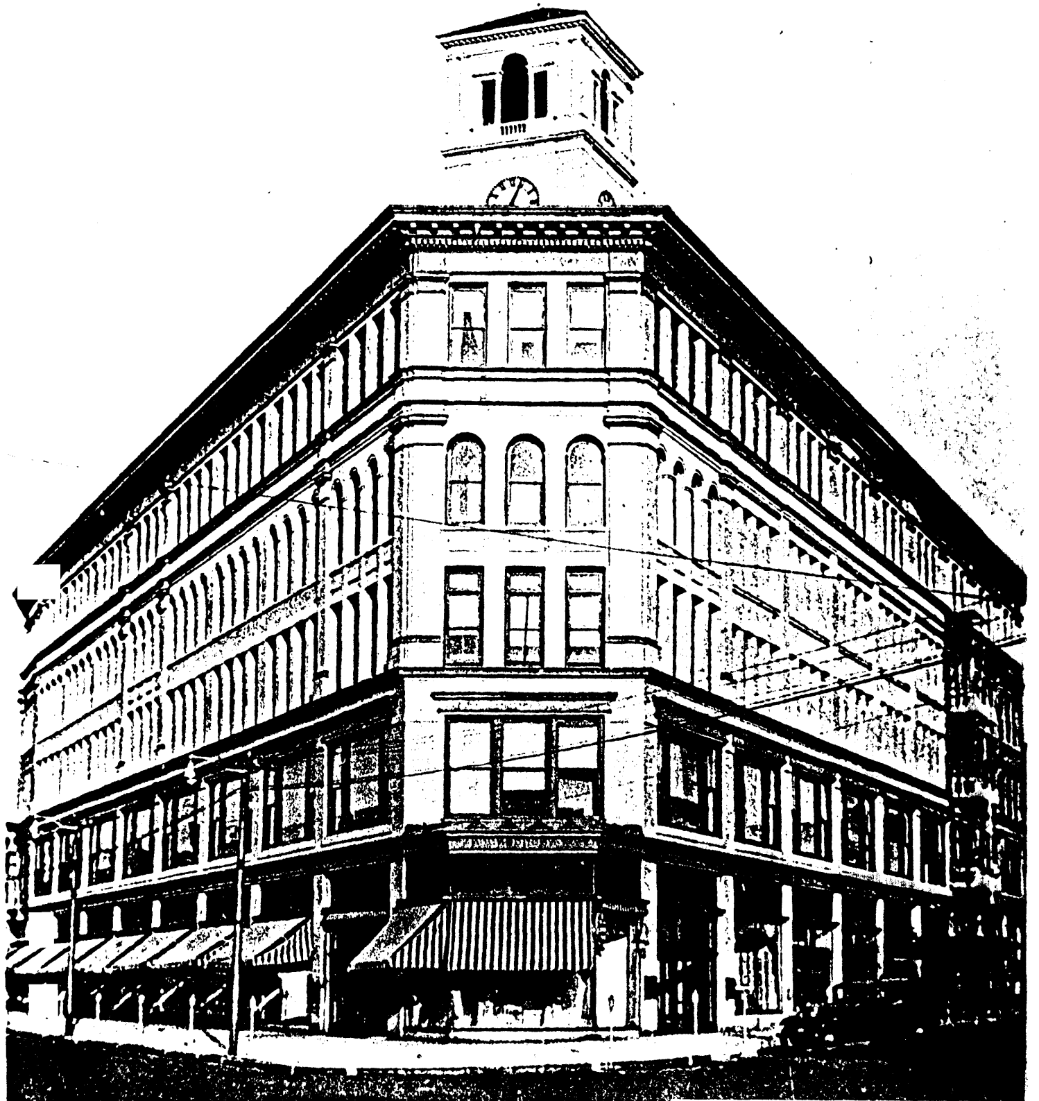
Steinbach/Cookman Building Asbury Park, Monmouth County, NJ c.1938 view of fifth floor added in 1920
