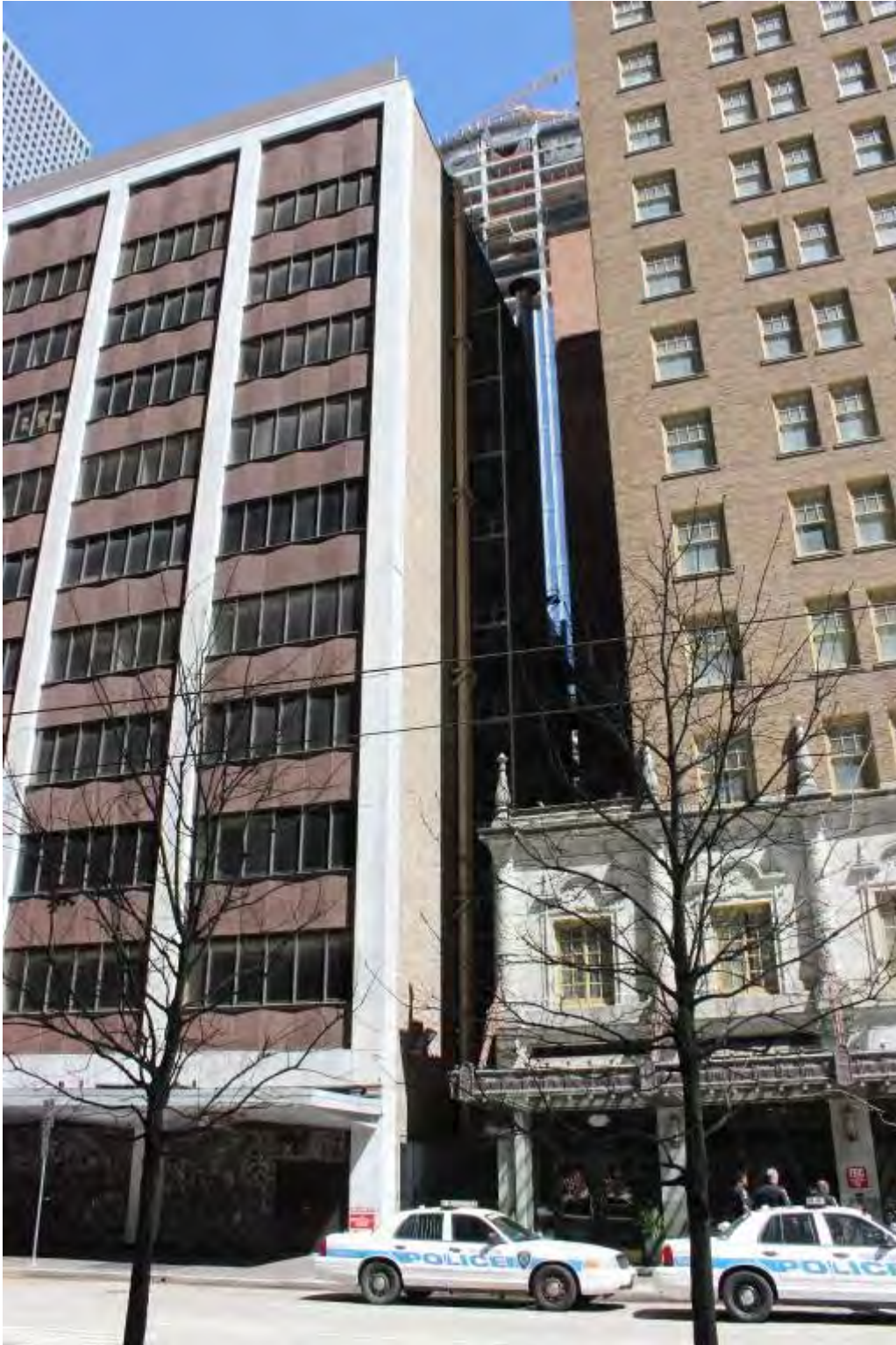
Photo 2 – Houston Bar Center Building, southwest and southeast elevations, view north.
