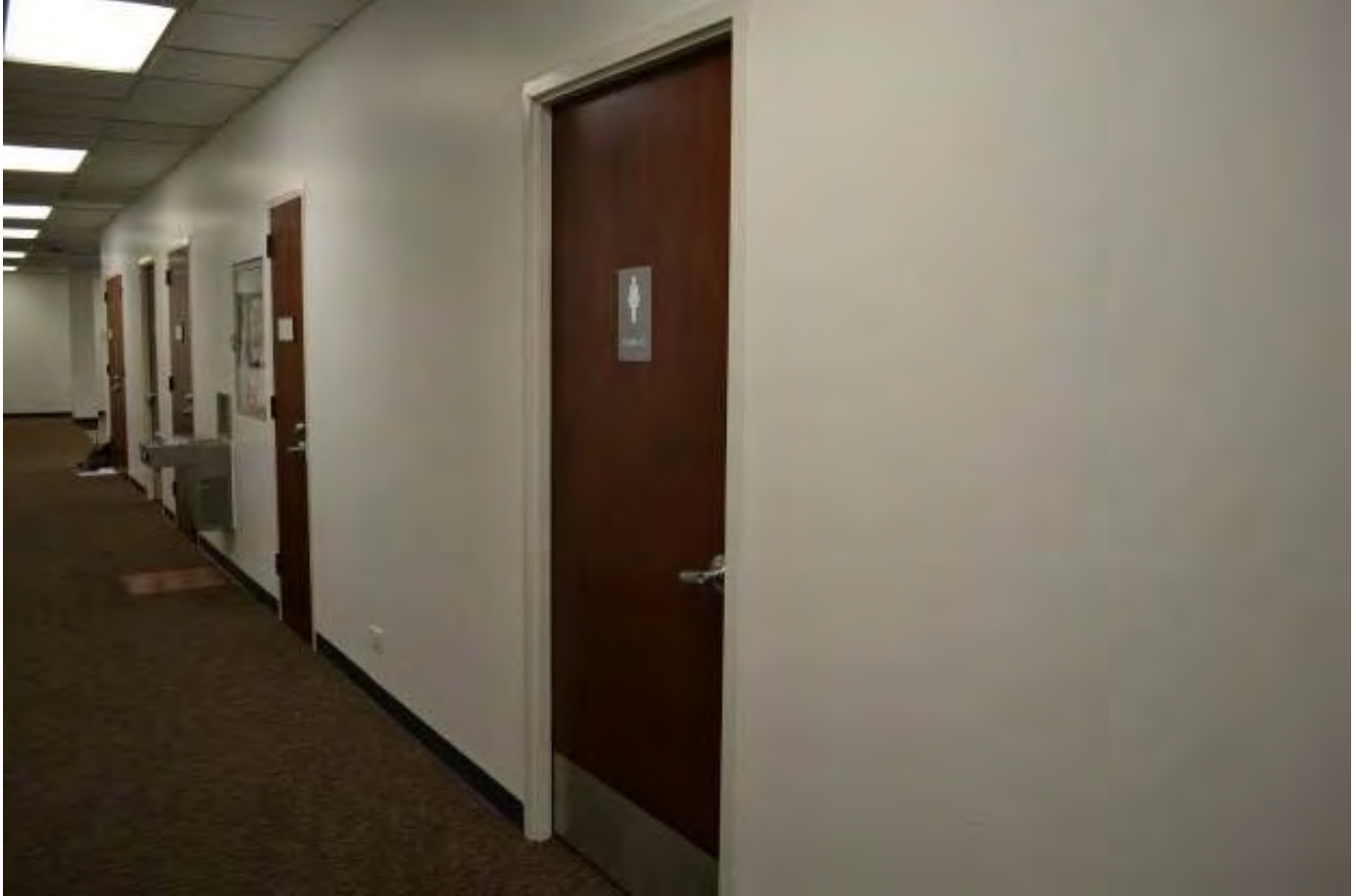
Photo 7 – Houston Bar Center Building, typical upper level corridor, view west.
