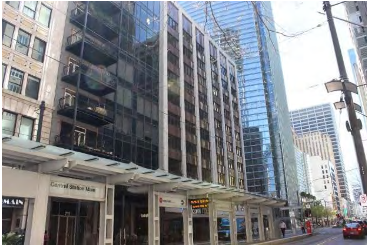
Photo 4 – Houston Bar Center Building, northwest elevation, view south. New light-rail station awning in foreground is not connected to the adjacent buildings.
