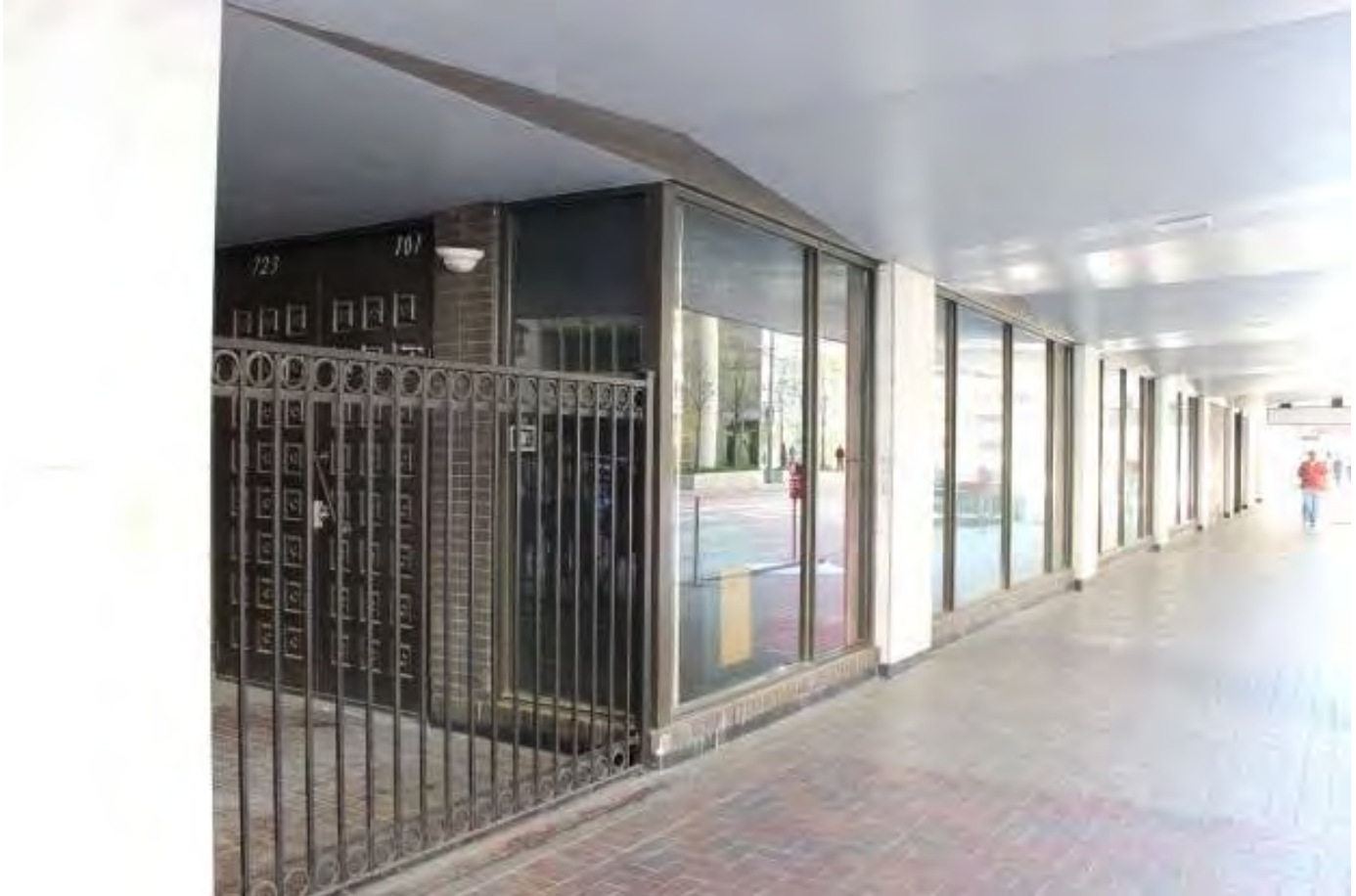
Photo 8 – Houston Bar Center Building, exterior walkway along south elevation, view east.
