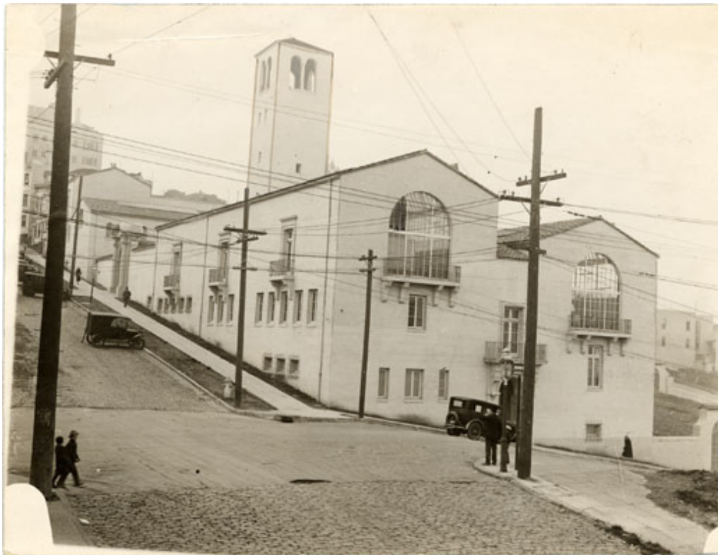
Figure 2: California School of Fine Arts, ca. 1927 Source: San Francisco Historical Photograph Collection.
