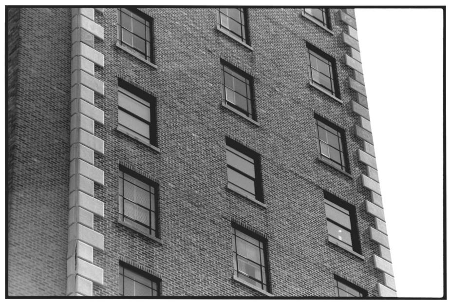
B- Closeup of windows, including unmatching windows; and deteriorating quoins.
