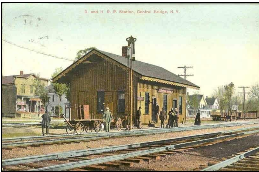
Figure 5: D & H Railroad Station (no longer extant), Central Bridge, NY.
