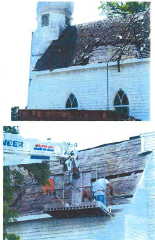
Fig. 20 (top left), 21 (top right), 22 (bottom left), & 23 (bottom right) Photos during roof restoration – Note structure and cedar shingles, ca. 2008 (courtesy of Fort Pembina Historical Society)
