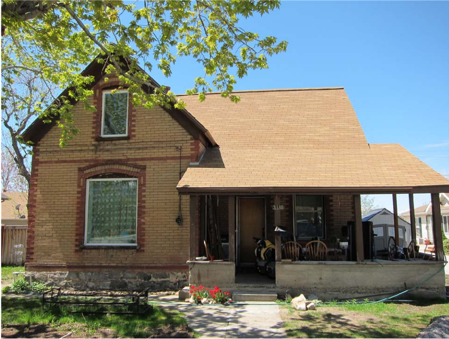
Photo No. 1 East Elevation. Camera facing west.
