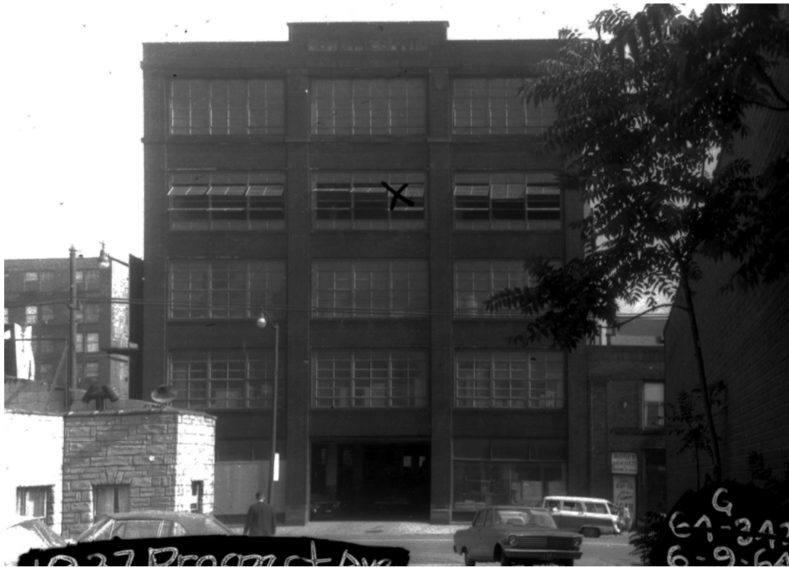
Fig. 2. Stuyvesant Motor Company Building, 1937 Prospect Avenue, Cleveland, Ohio Cleveland Landmarks Commission Photo dated June 9, 1964
