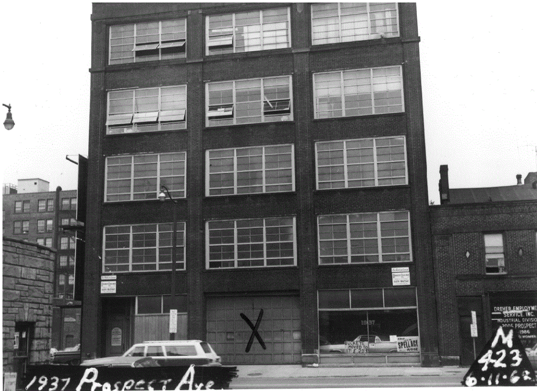
Fig. 1. Stuyvesant Motor Company Building, 1937 Prospect Avenue, Cleveland, Ohio Cleveland Landmarks Commission Photo dated June 11, 1962 (?)
