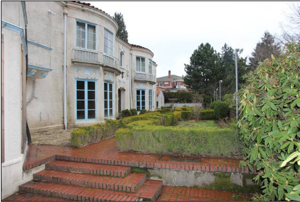
Photo 5 of 32: South façade from southwest corner patio.
