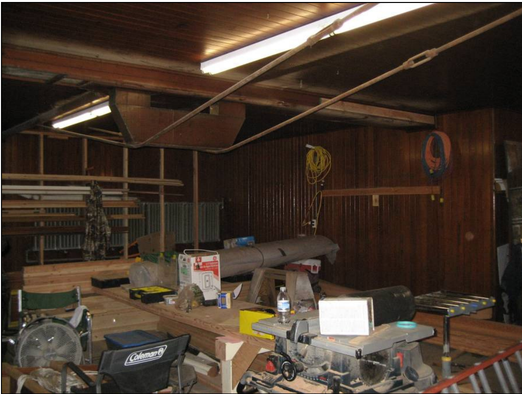
Photo 32 of 32: Unique structural spanning system in garage.
