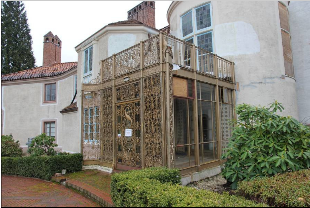
Photo 9 of 32: Wrought-iron and bronze glazed entry porch on north elevation.
