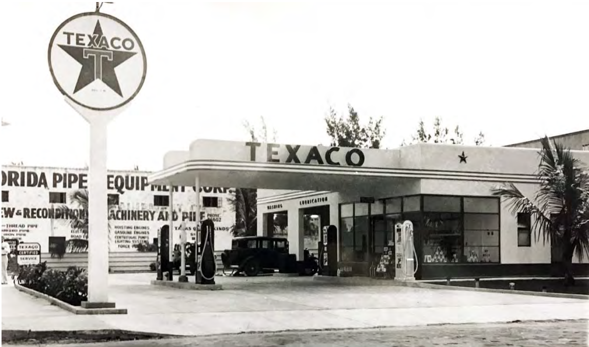
Texaco station in Miami, Florida, c.1937
