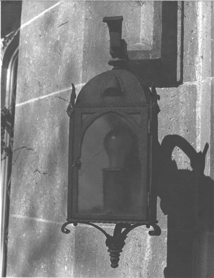
Detail of lighting fixture at Main Entrance: 1 of a pair of bracket landerns, triangular as per special design, rusty iron and brass.
