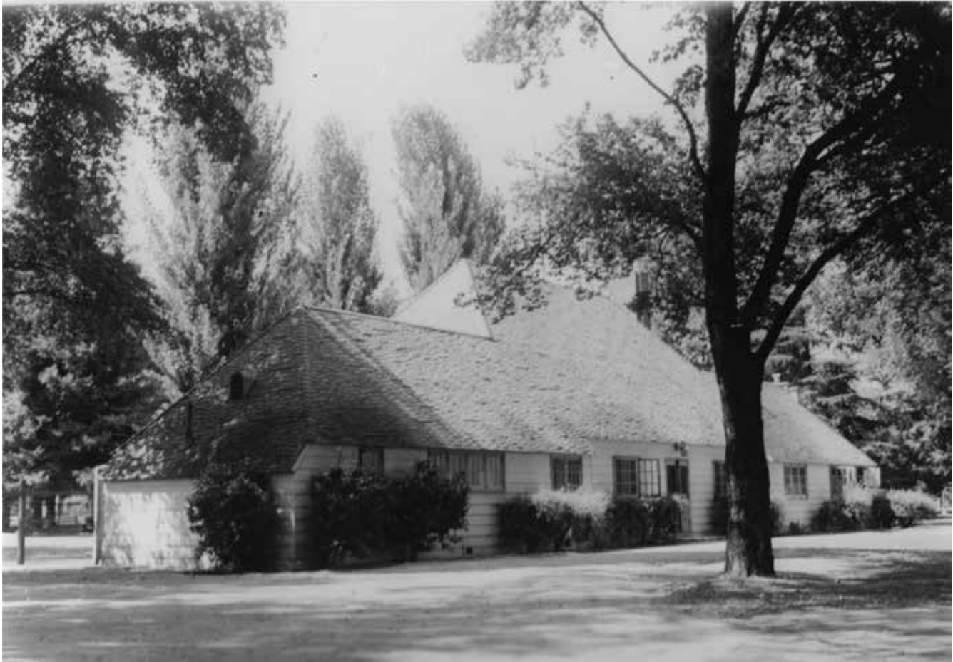
Figure 11, Southside Park clubhouse, no longer extant. Sacramento Public Library photo
