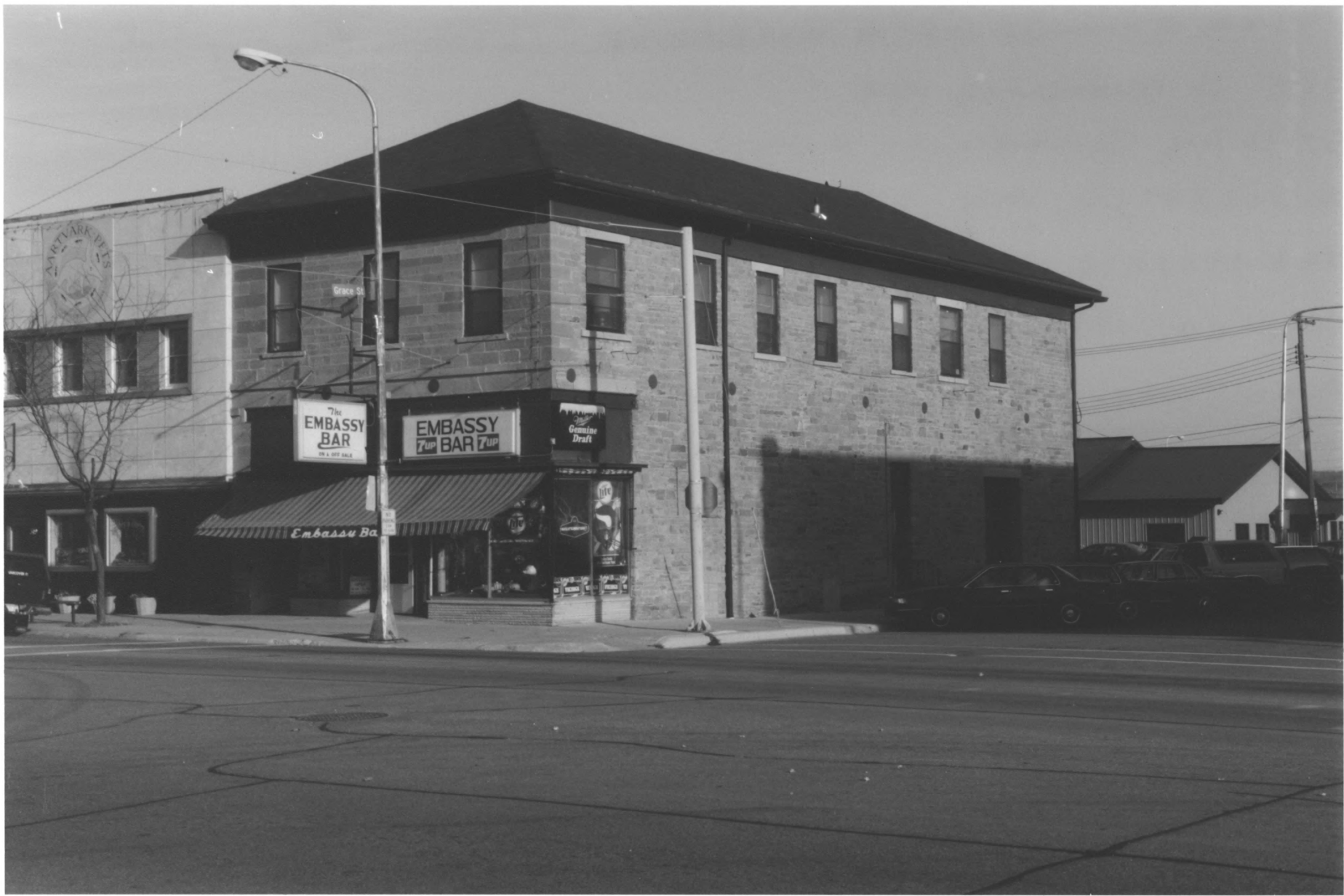
WILLIAM SCHIMMEL GRAIN WAREHOUSE ST PETER COMMERCIAL HISTORIC DISTRICT NICOLLET CO., MN 013613-4A
