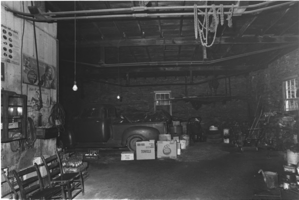
47. Ellis Garage Nashville, Davidson County, TN.
