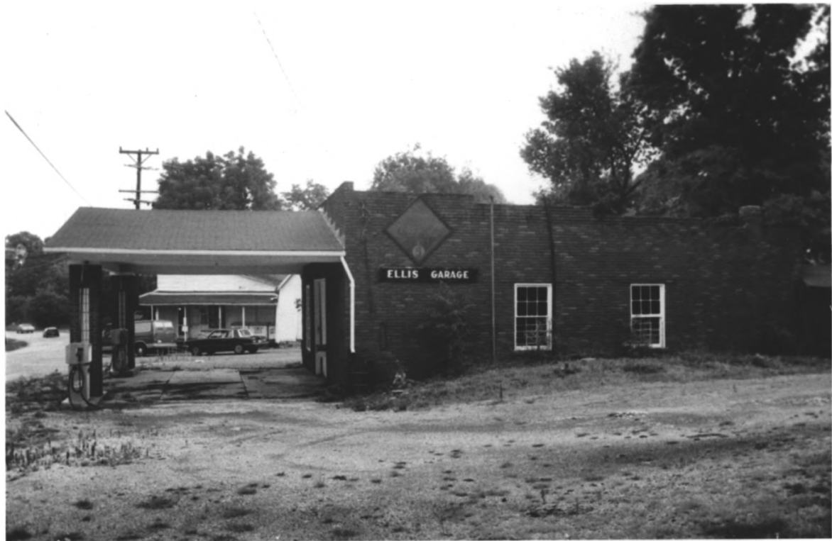
#4 Ellis Garage Nashville, Davidson County, TN.
