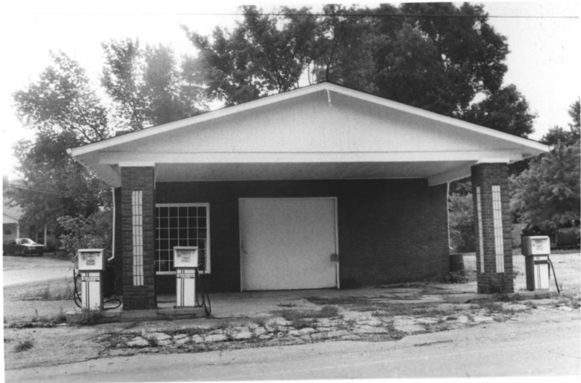
#2 Ellis Garage Nashville, Davidson County, TN.
