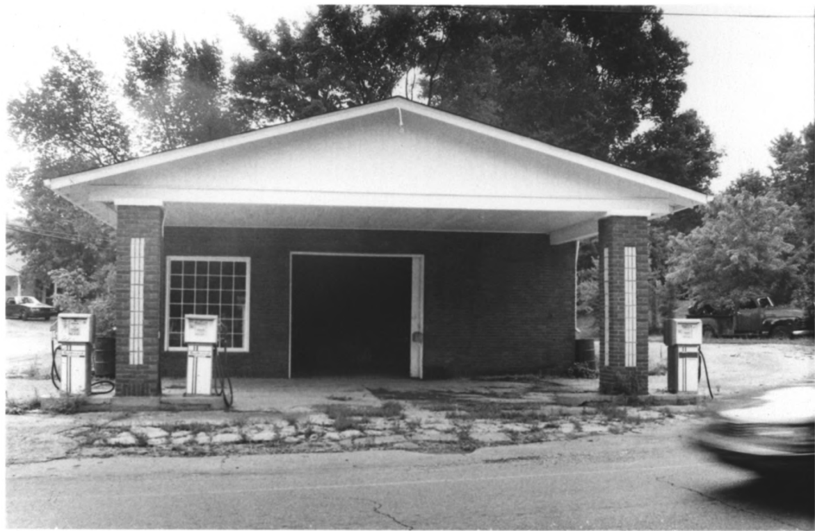
#1 Ellis Garage Nashville, Davidson County, TN.
