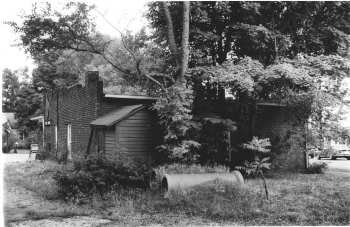
#5 Ellis Garage Nashville, Davidson County, TN.
