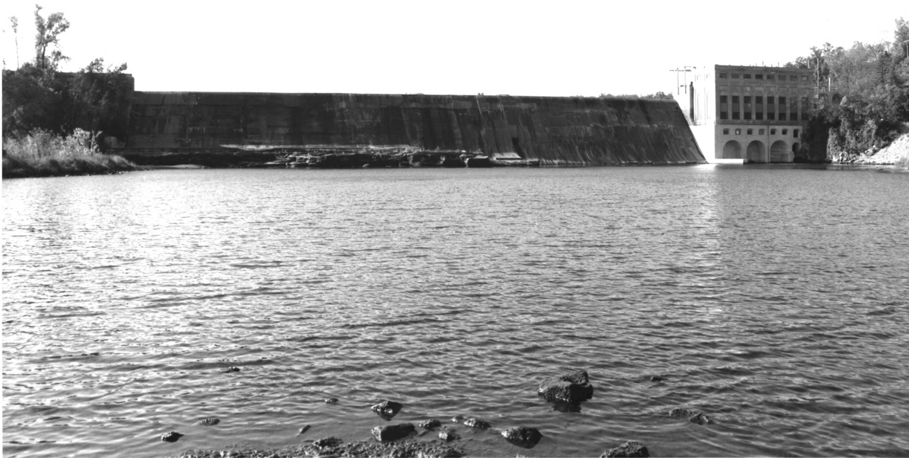
Lake Zumbro Hydroelectric Generating Plant Mazeppa Twp., vicinity of Mazeppa, Wabasha Co., MN 010526-21
