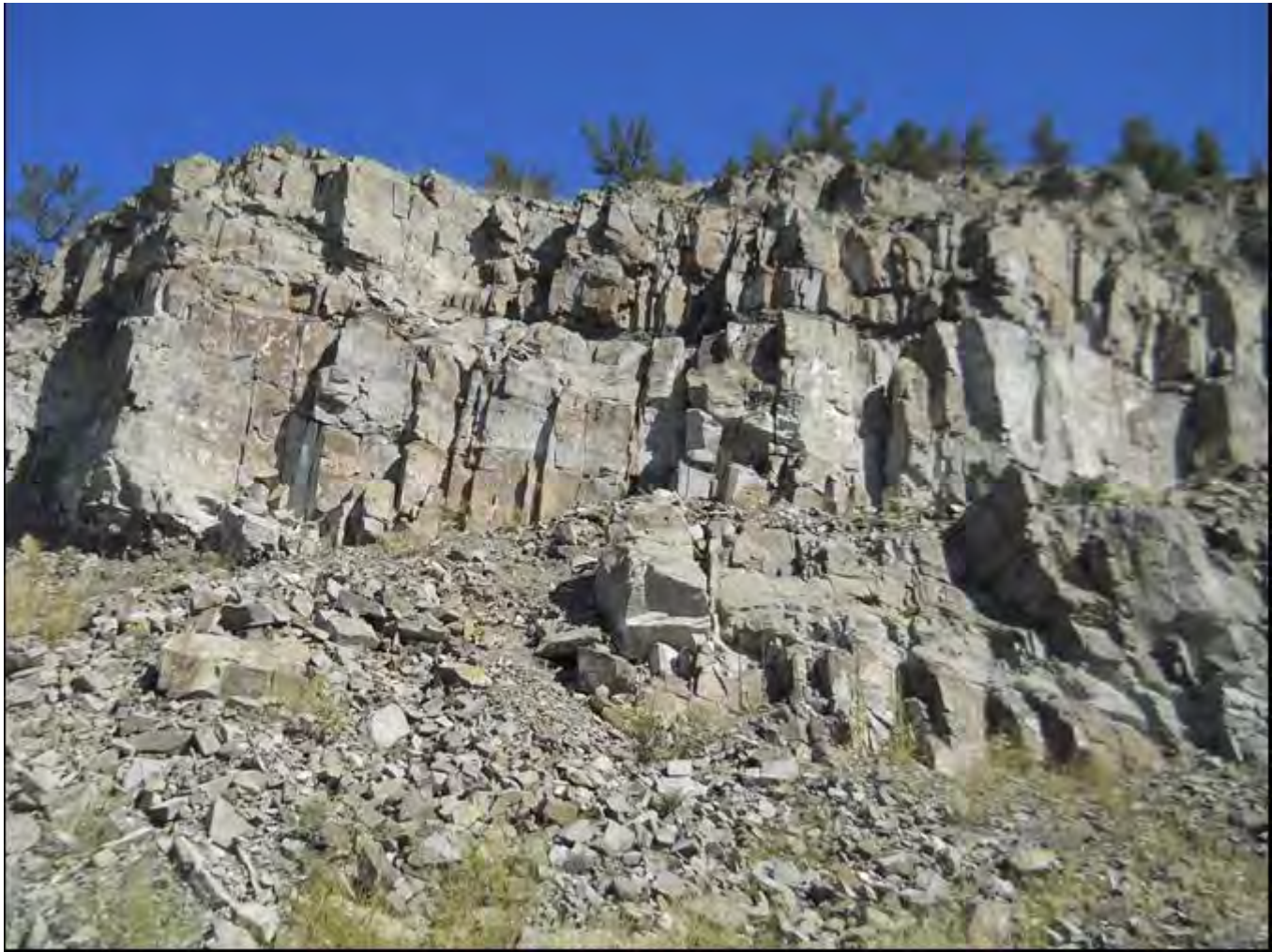
Photo 0008. Detail of scaled rock, MP 0.8. View to the north.
