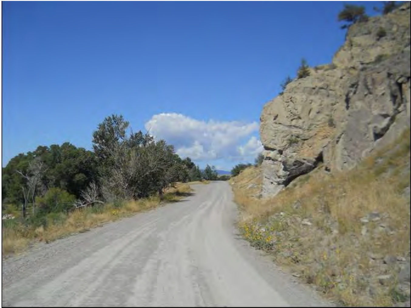
Photo 0021. Convict Grade, MP 1.7. View to the west.
