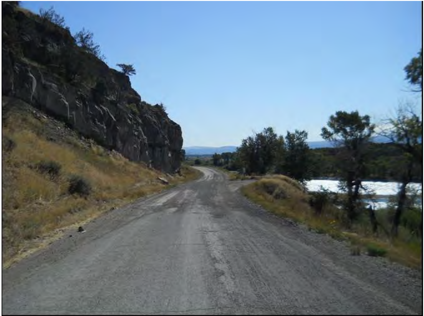
Photo 0003. Convict Grade, MP 0.6. View to the east.
