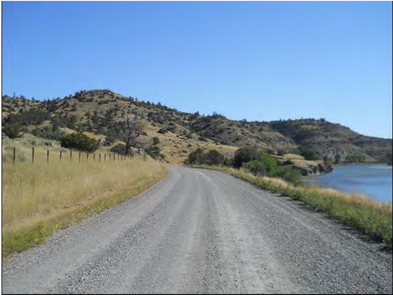
Photo 0011. Convict Grade, MP 0.9. View to the east.
