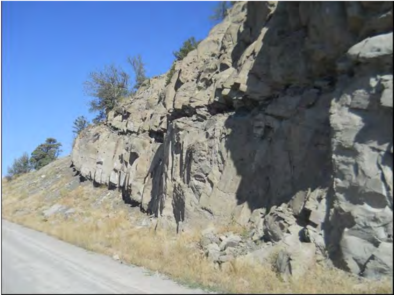
Photo 0006. Detail of rock scaling, MP 0.7. View to the northwest.
