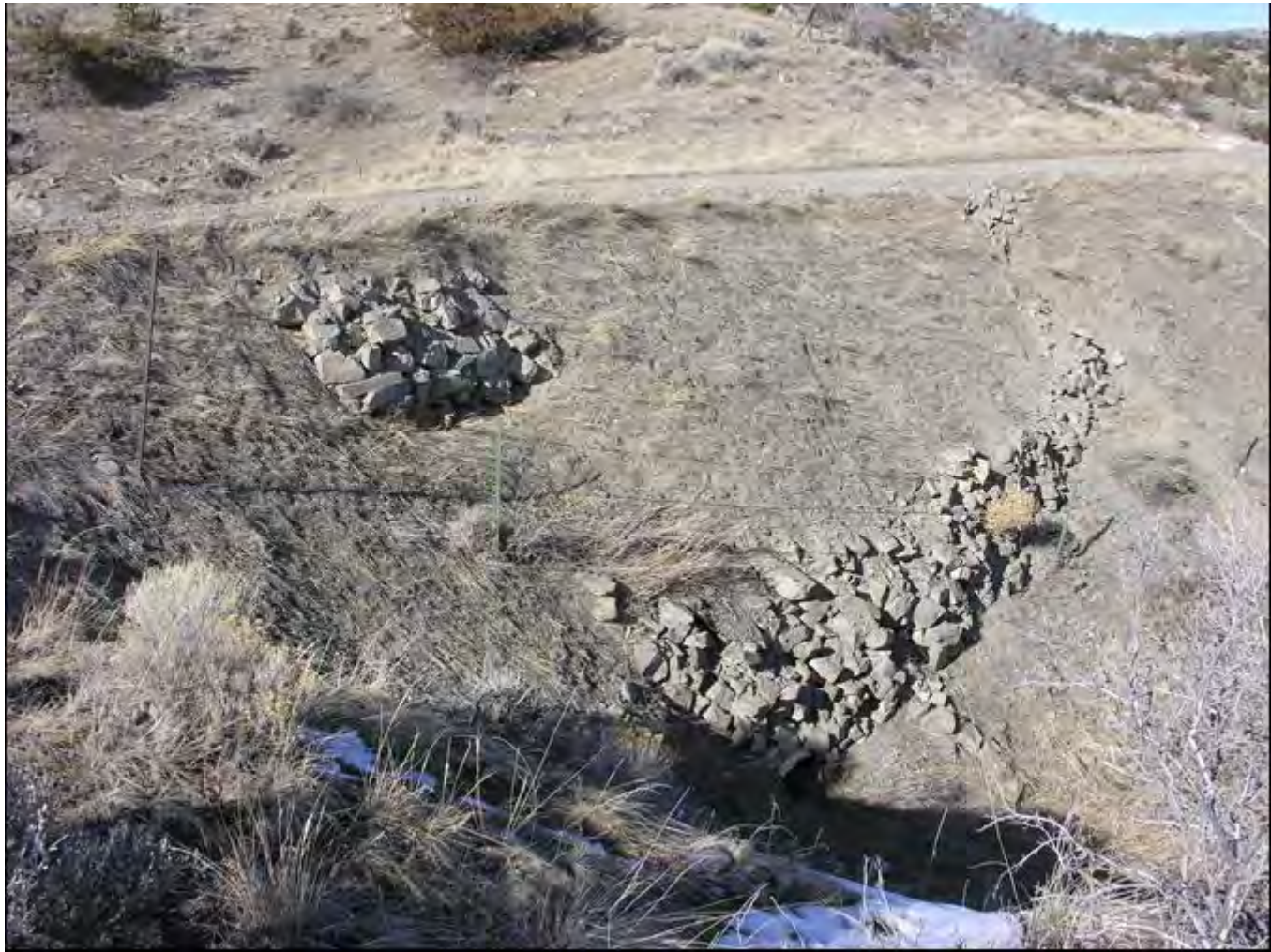
Photo 0029. Rock Retaining Wall, MP 2.65. View to the north.
