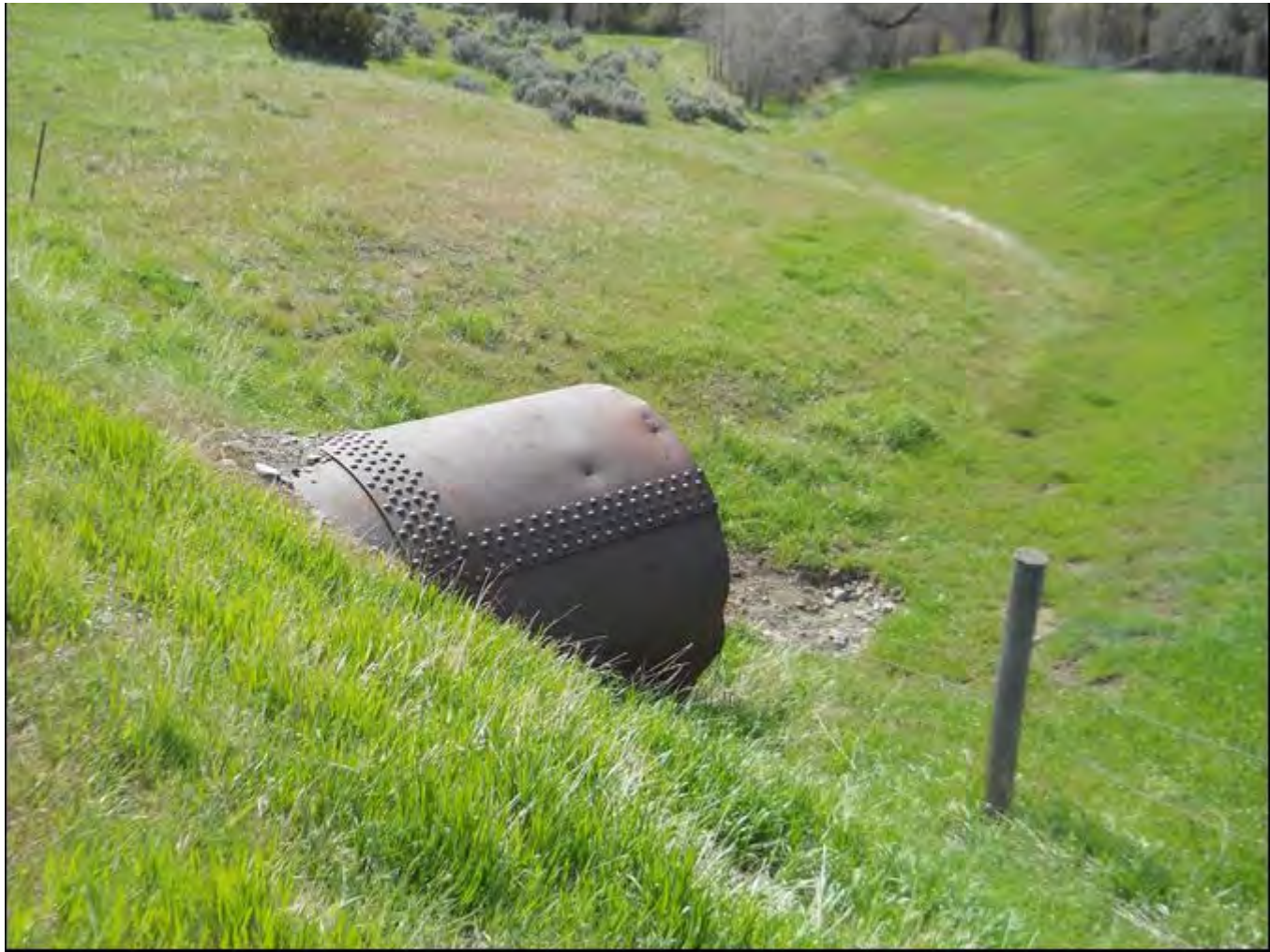
Photo 0002. Riveted Steel Culvert, MP 0.5. View to east-southeast.
