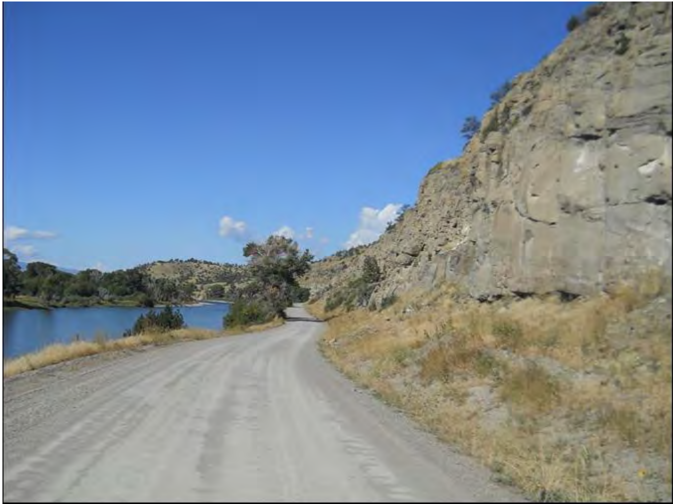
Photo 0025. Convict Grade, MP 2.0. View to the west.
