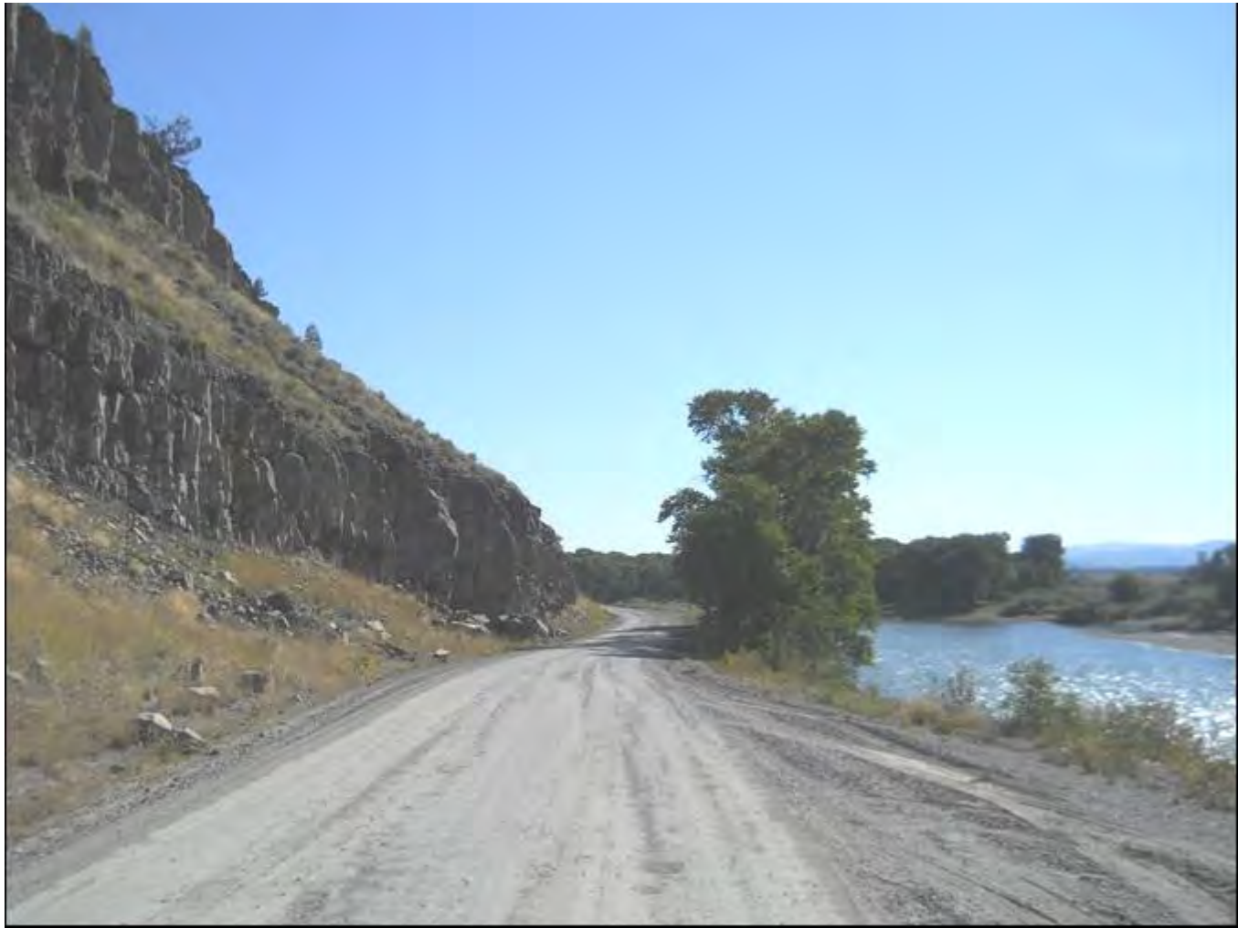
Photo 0007. Convict Grade, MP 0.7. View to the east.
