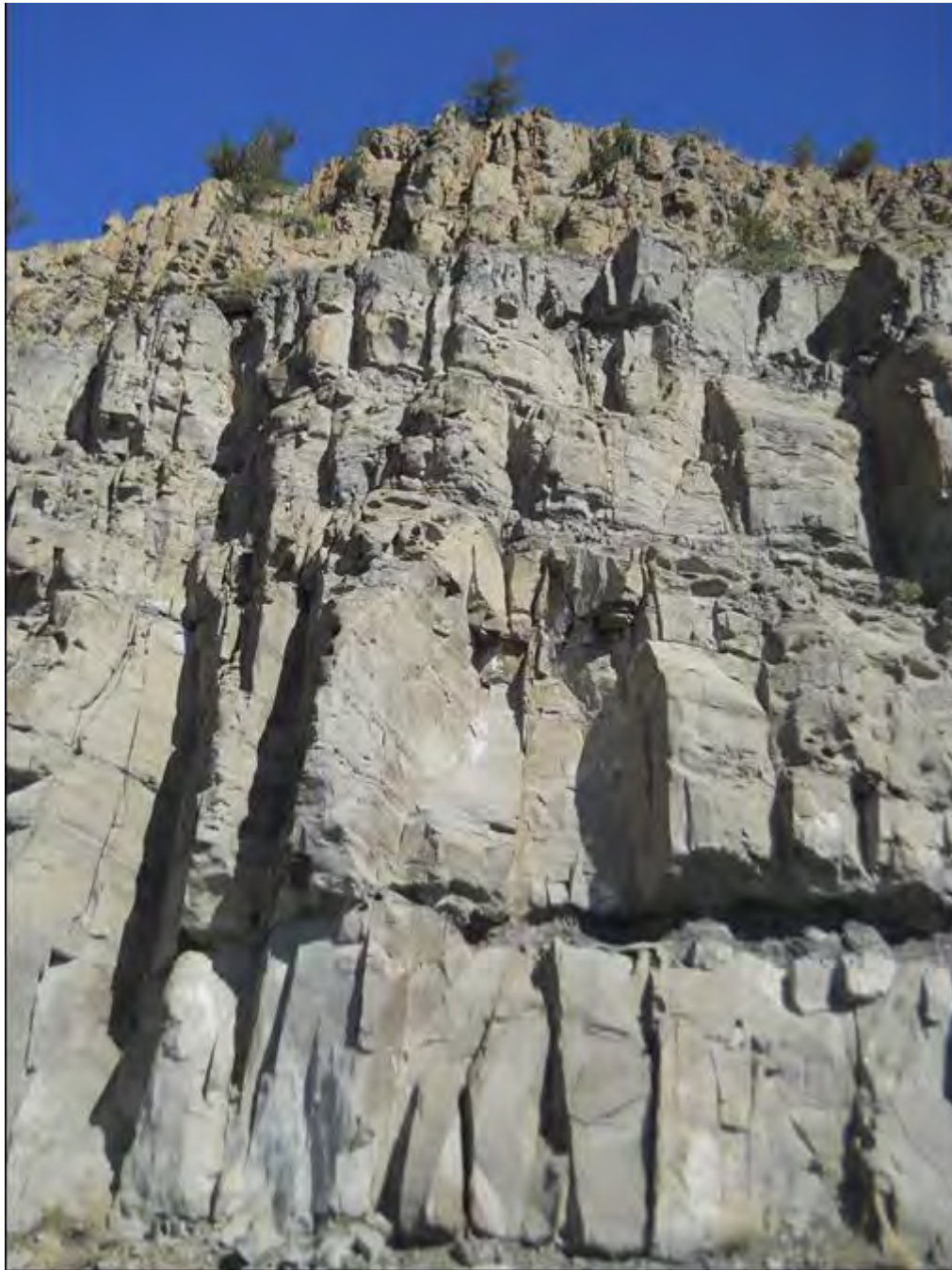
Photo 0026. Detail of rock scaling, MP 2.0. View to the north.
