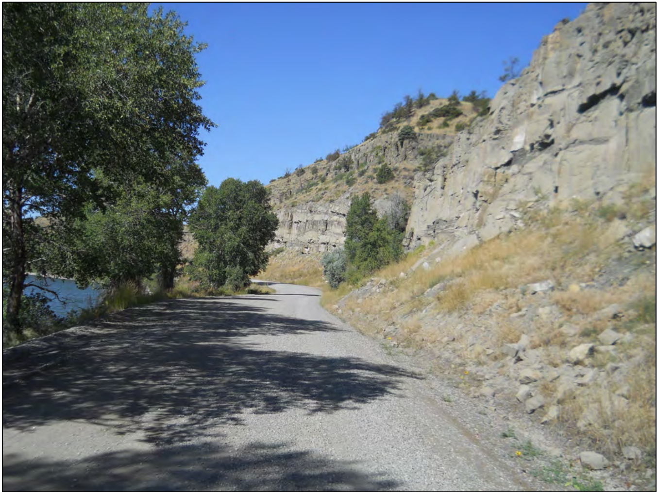
Photo 0016. Convict Grade, MP 1.58±. View to the west.
