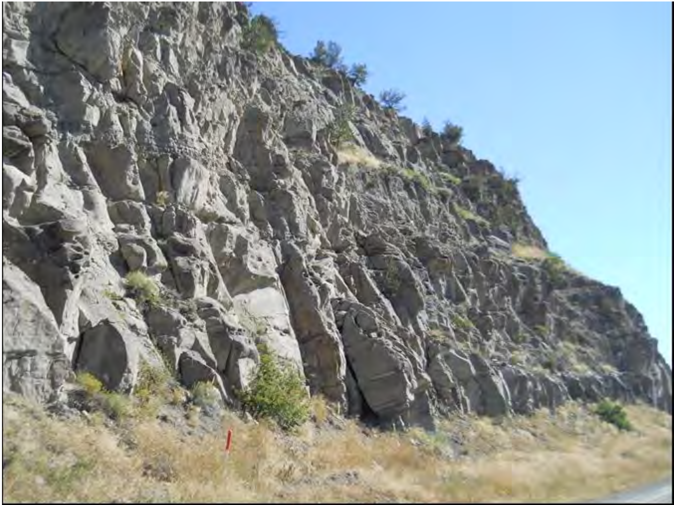
Photo 0023. Detail of rock scaling, MP 1.85. View to the northeast.
