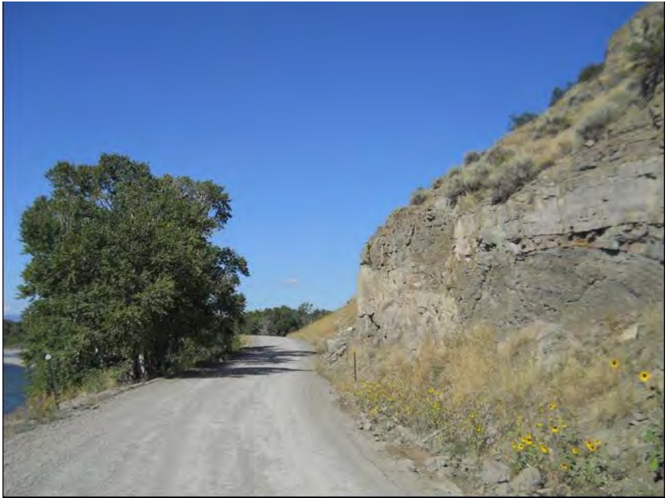
Photo 0010. Convict Grade, MP 0.9. View to the west.
