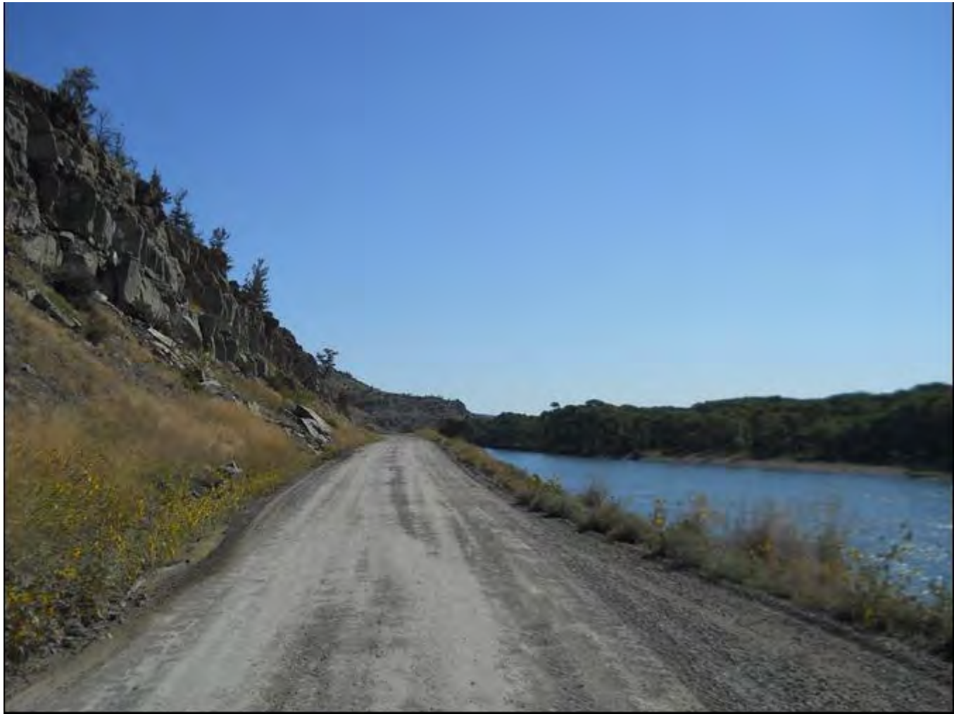
Photo 0009. Convict Grade, MP 0.8. View to the east.
