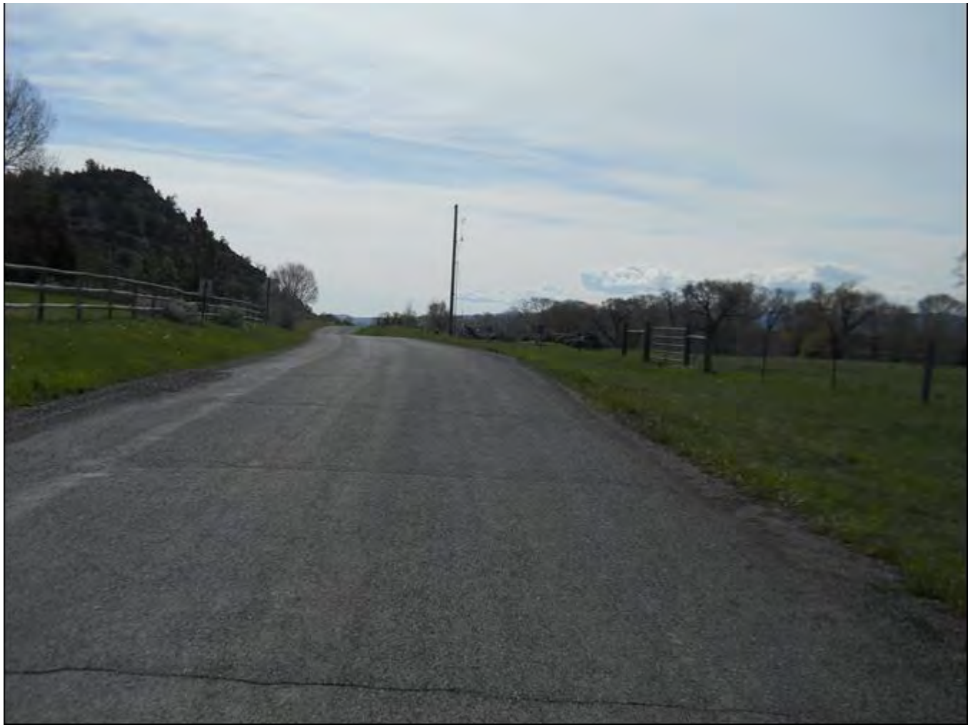
Photo 0001. West end of Convict Grade Segment, MP 0.45. View looking east.
