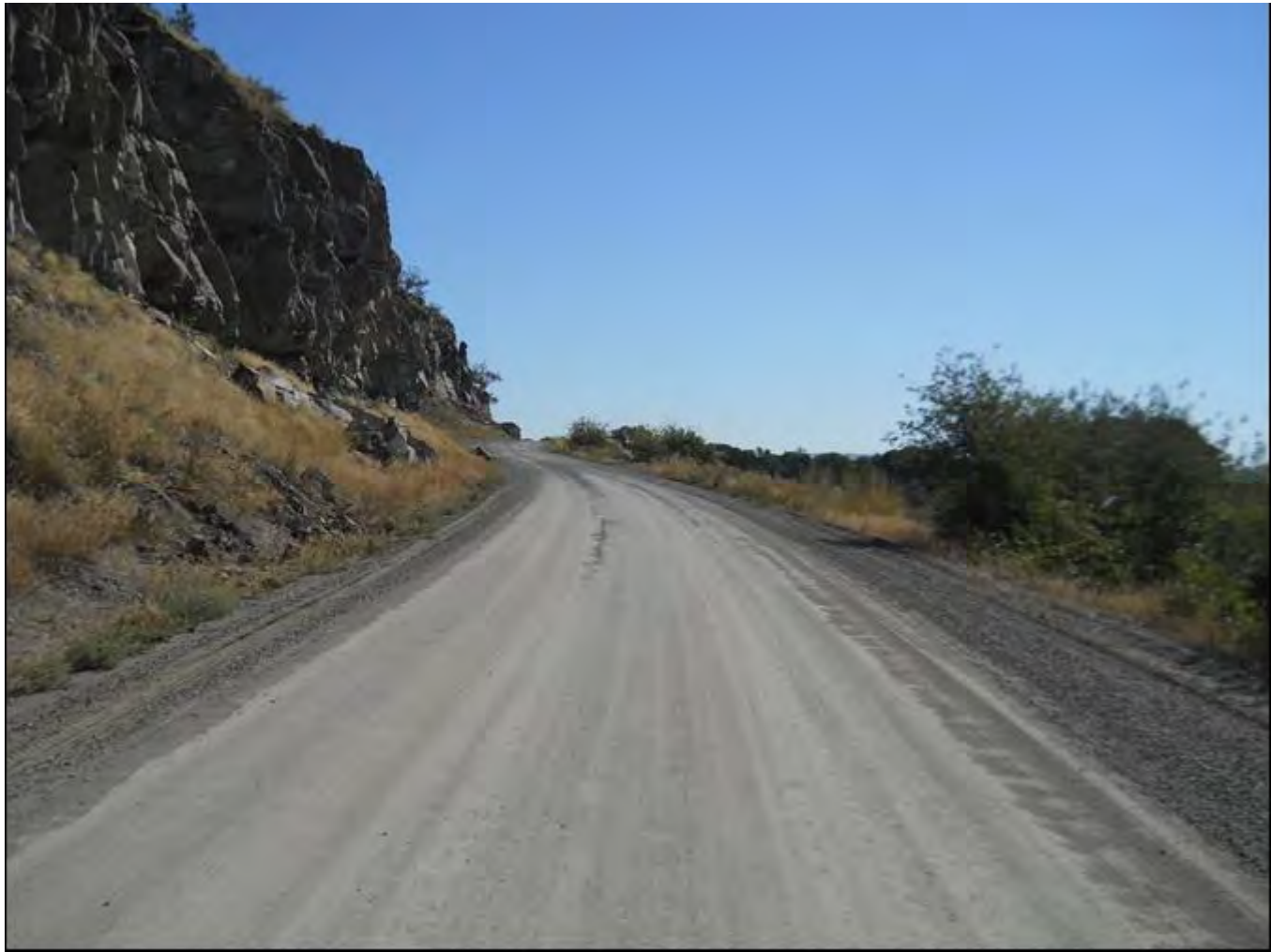
Photo 0024. Convict Grade, MP 1.85. View to the east.
