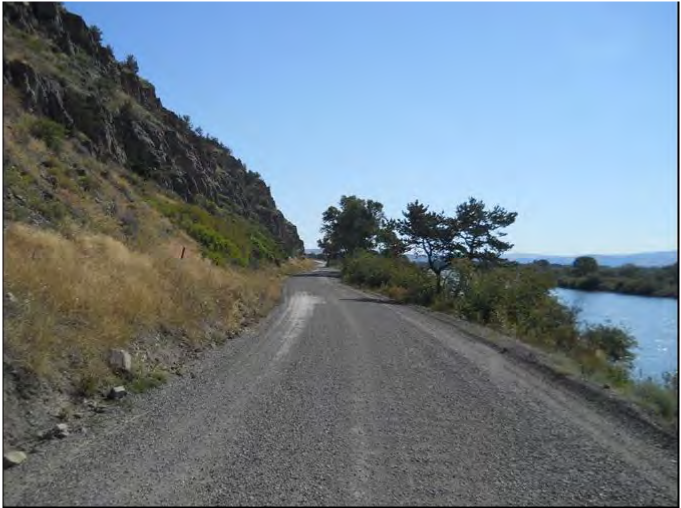
Photo 0019. Convict Grade, MP 1.65±. View to the east.
