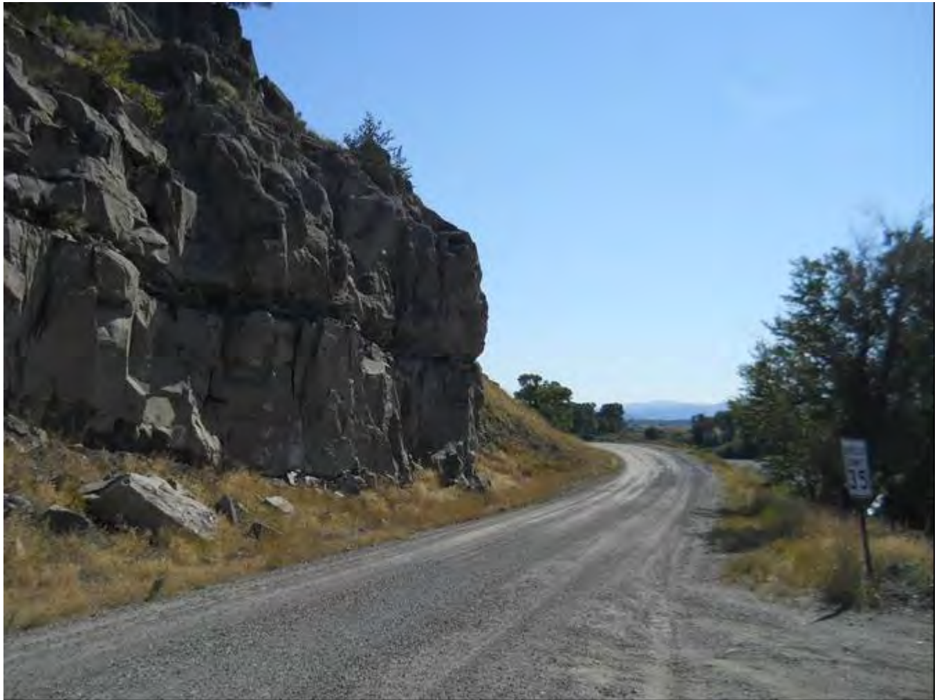
Photo 0004. Convict Grade, MP 0.7. View to the east.
