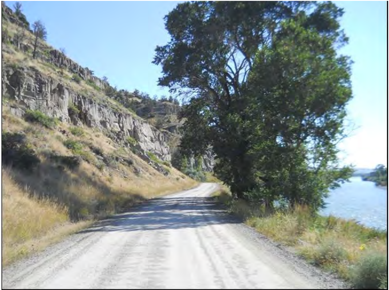
Photo 0012. Convict Grade, MP 1.3. View to the east.
