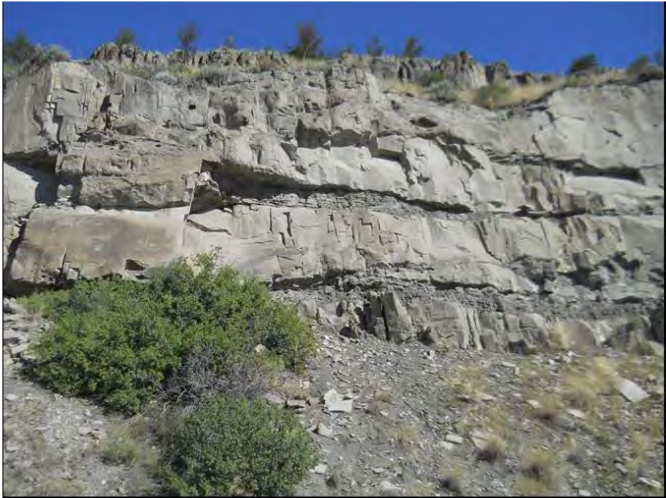
Photo 0013. Detail of scaled rock, MP 1.5. View to the north.
