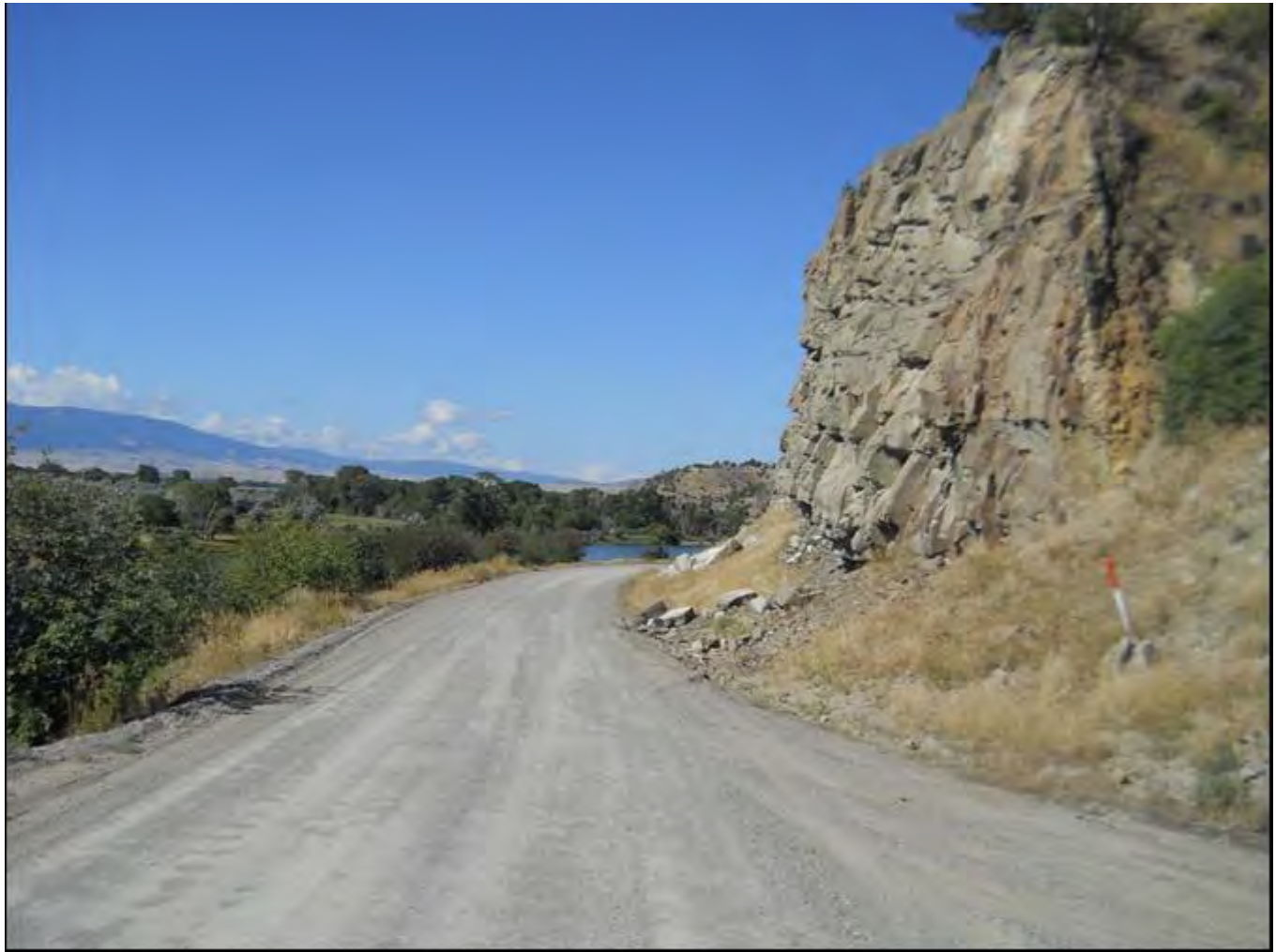
Photo 0027. Convict Grade, MP 2.05. View to the west.
