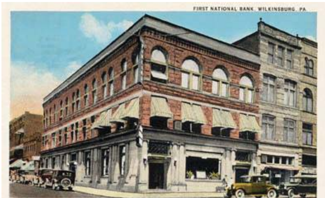
Figure 11. Circa 1943 postcard of the National Bank of Wilkesburg (#27) at the northeast corner of Penn Avenue and Wood Street, looking northeast. Wilkesburg Historical Society.
