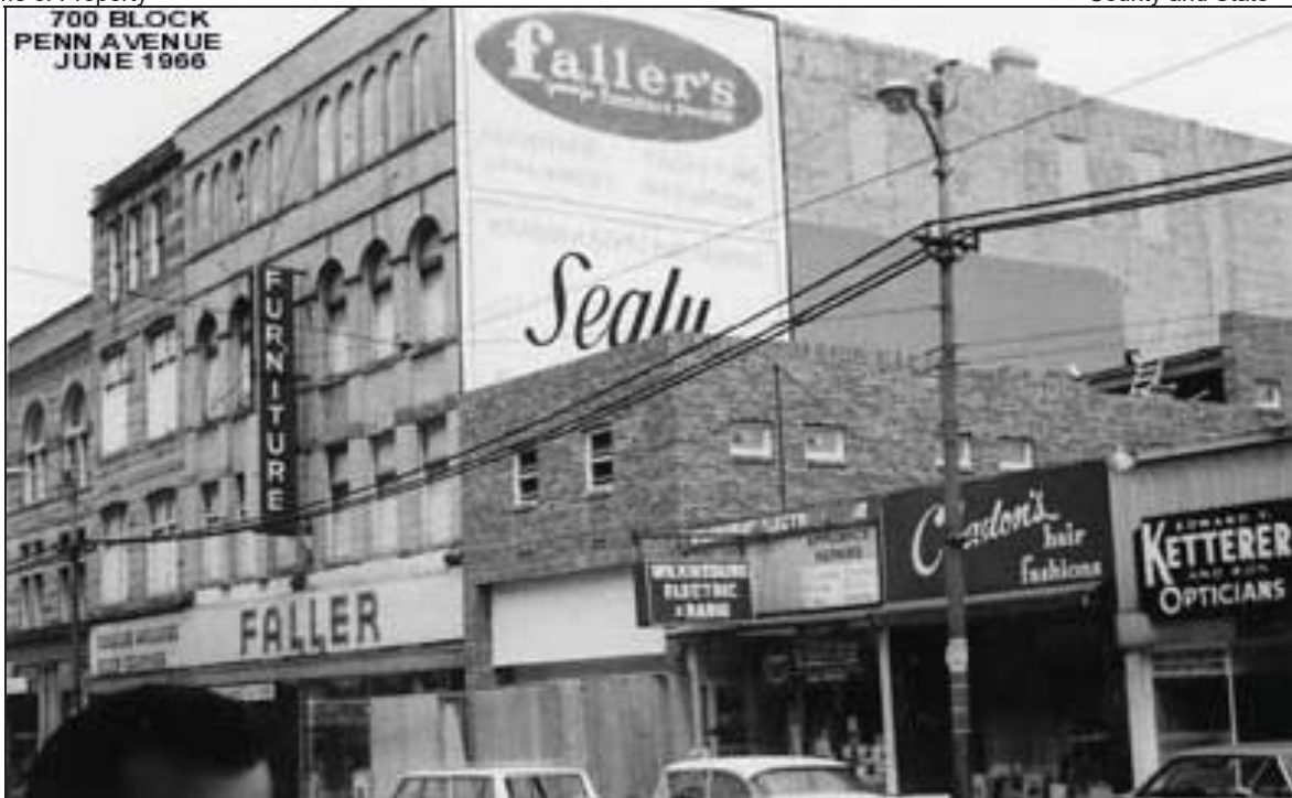
Figure 14. 1966 view of 700 Block Penn Avenue looking northwest. The National Bank of Wilkesburg and Walmer's Hardware (#27 and #28; far left), Puffinburg Furniture Company Building (#29; left), and several non-contributing buildings (#30, 31, and #32) are visible. Wilkesburg Historical Society.
