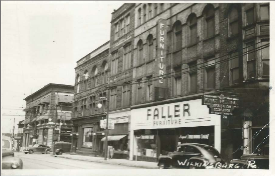
Figure 12. Penn Avenue looking northwest toward Wood Street, circa 1930. The Hunter Building (#26; left), National Bank of Wilkesburg (#27; center left), Walmer's Hardware Building (#28; center right), and Puffinburg Furniture Company Building (#29; right) are visible. Wilkesburg Historical Society.
