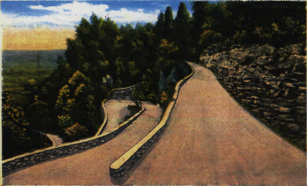
THE "W" WALDEN'S RIDGE, ALONG THE DIXIE HIGHWAY, 7 MILES FROM CHATTANOOGA, TENN.—4
