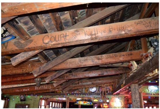
Photo 25. Detail of original roof truss system of Riley's Tavern (Resource #1), located in ca. 1935 addition of saloon.
