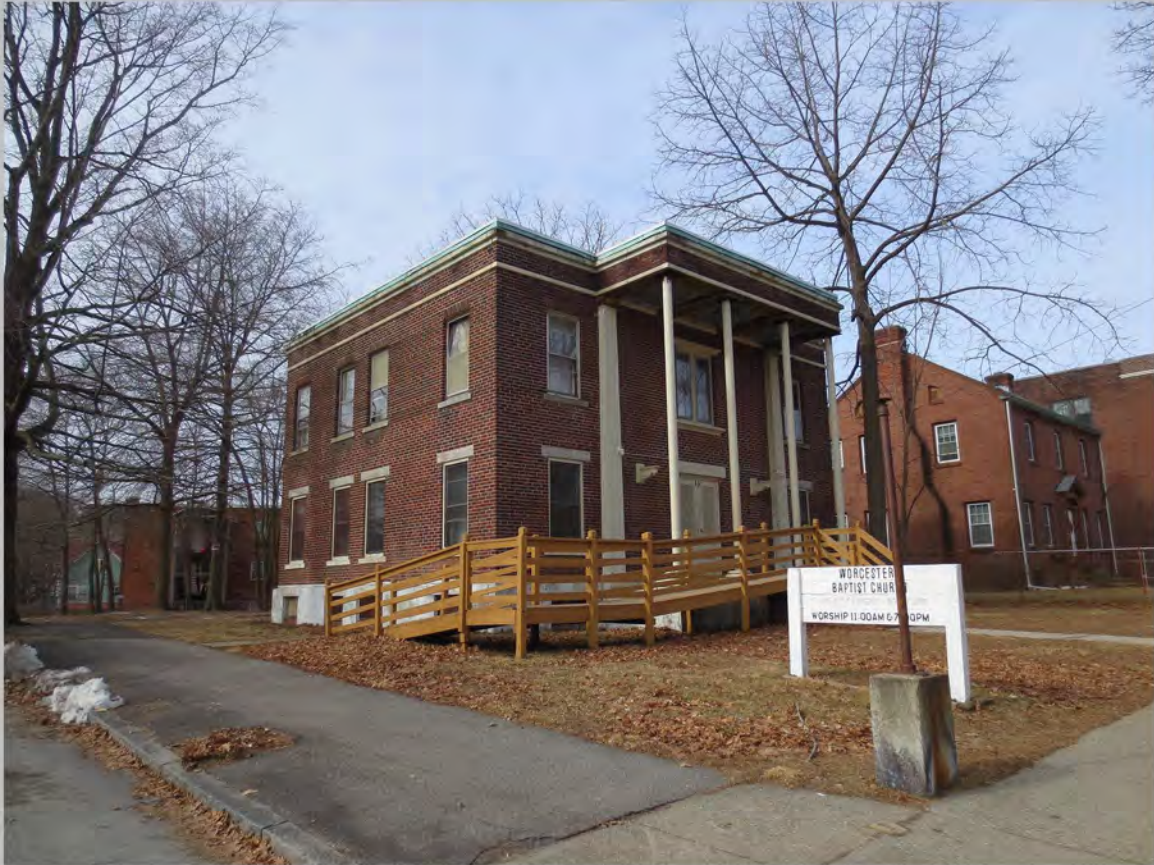
11. 15 and 17 Ethan Allen Street, south and east elevations, view northwest
