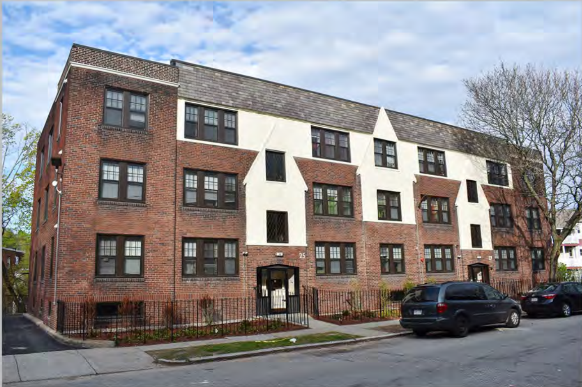
9. 25–27 Ethan Allen Street, front (east); view west
