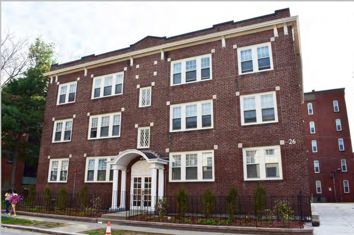
8. 26 Ethan Allen Street, front (west) elevation; view northeast
