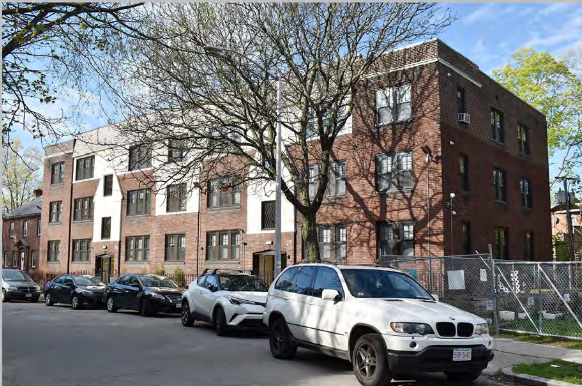
10. 25–27 Ethan Allen Street, front (east) and north elevations; view southwest
