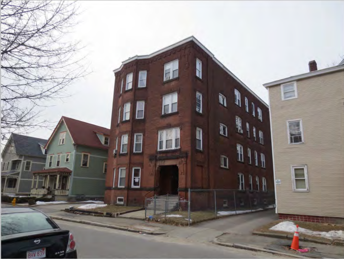
1. 18 Dale Street, east and north elevations; view southwest
