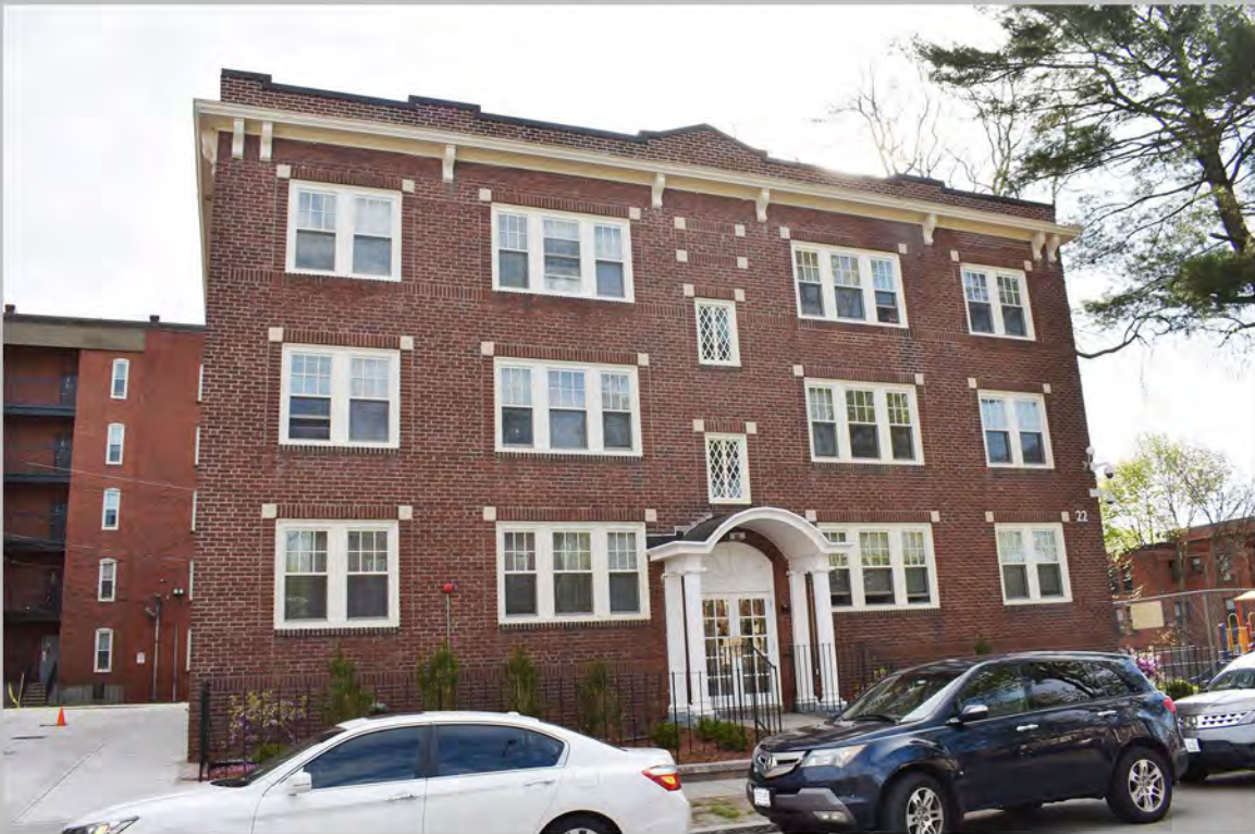
6. 22 Ethan Allen Street, north and west elevations; view southeast (May 2019)
