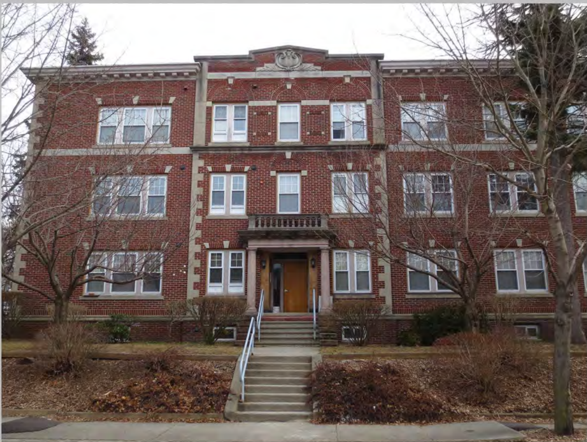
4. 11–15 Dale Street/1 Allendale Street, west elevation; view east
