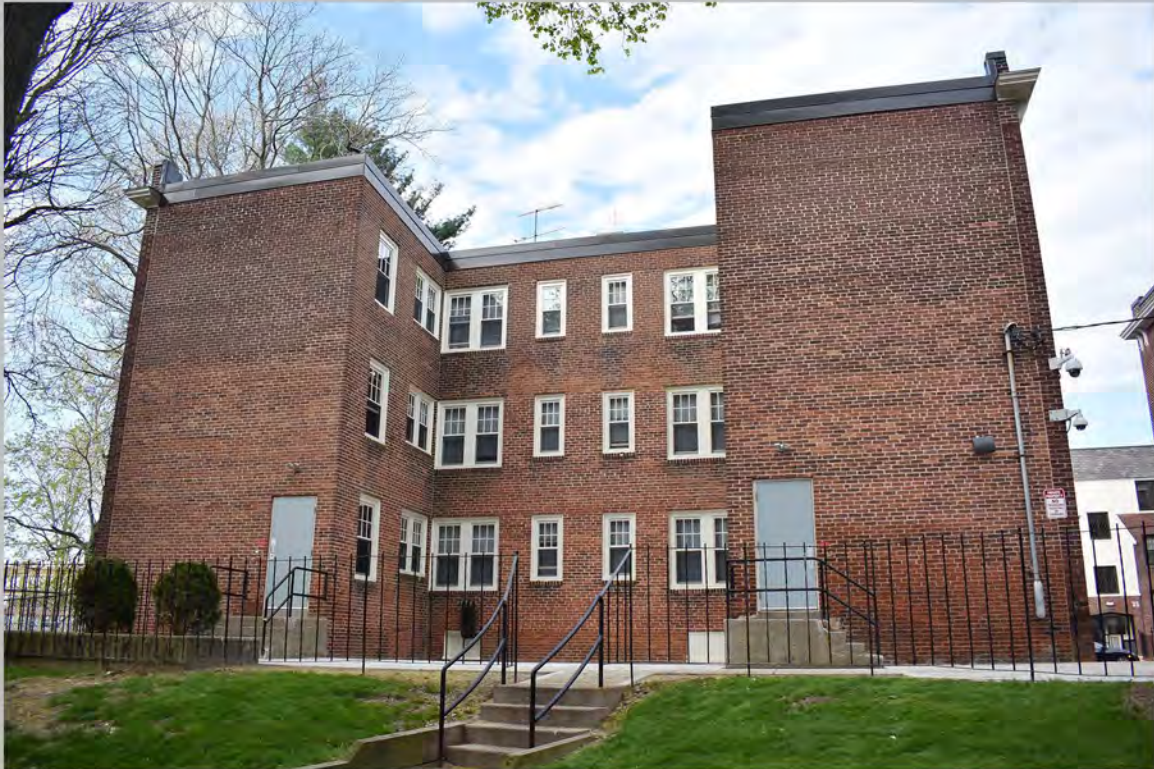
7. 22 Ethan Allen Street, north and east elevations; view southwest
