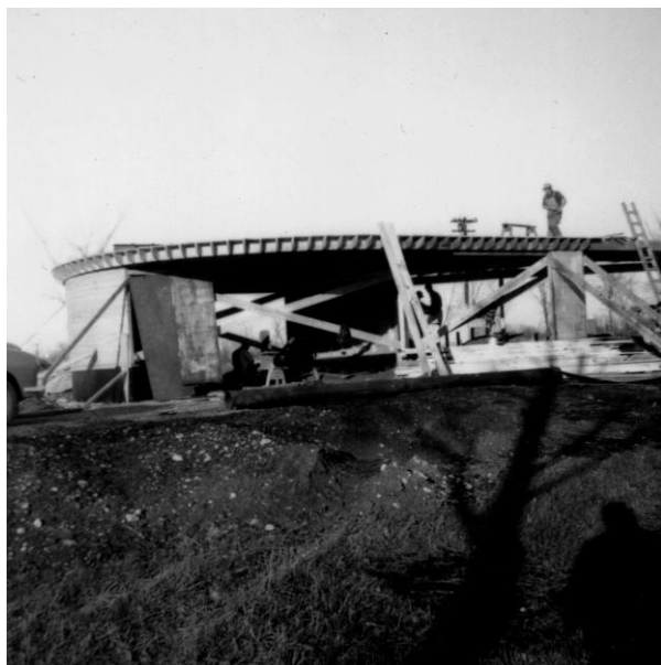
Photograph of construction of porte cochere from southwest, November 1949.
