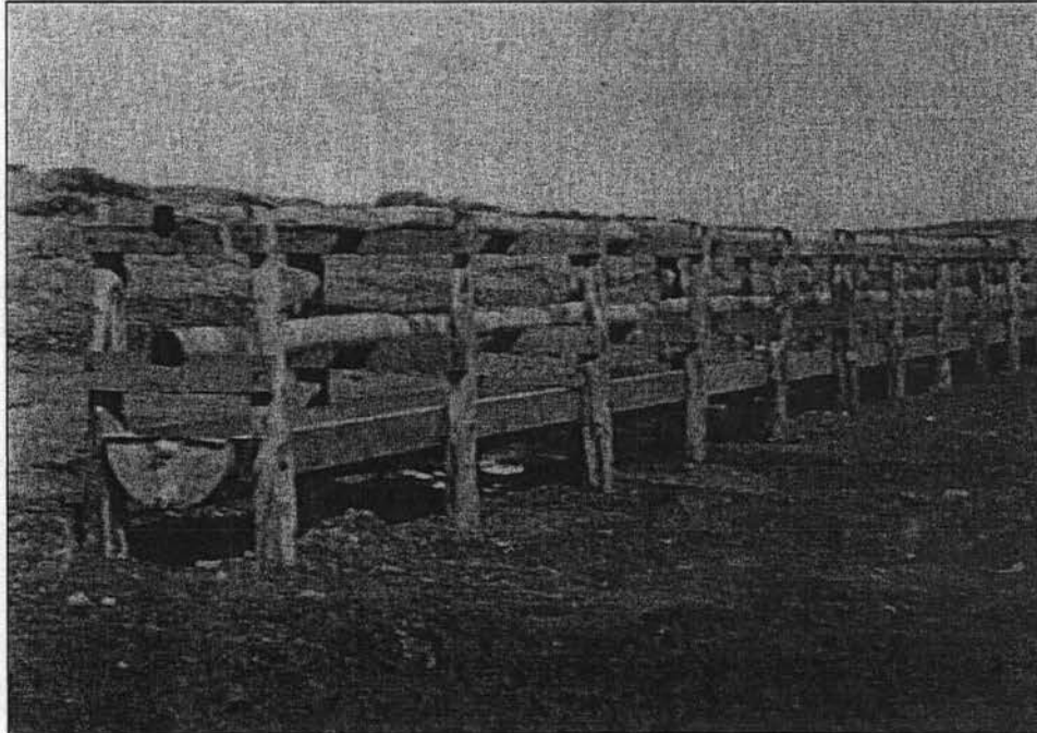
Figure 2. Civilian Conservation Corps workers from the Dalton Wells camp (DG-32) initially hewed logs by hand to produce livestock watering troughs, but soon turned to this design that used upright posts, a wood framework, and galvanized, sectional metal troughs. This 100' trough at Dubinky Well displays the same design as those in the nominated area. SOURCE: Allred, "Eighth Period Report," 31 March 1937.
