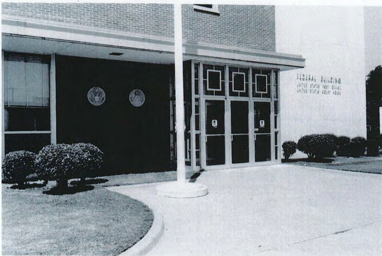
View of main entry, U.S. Post Office and Courthouse, Helena, Arkansas (GSA EDOCs Photo 3958; unknown date).
