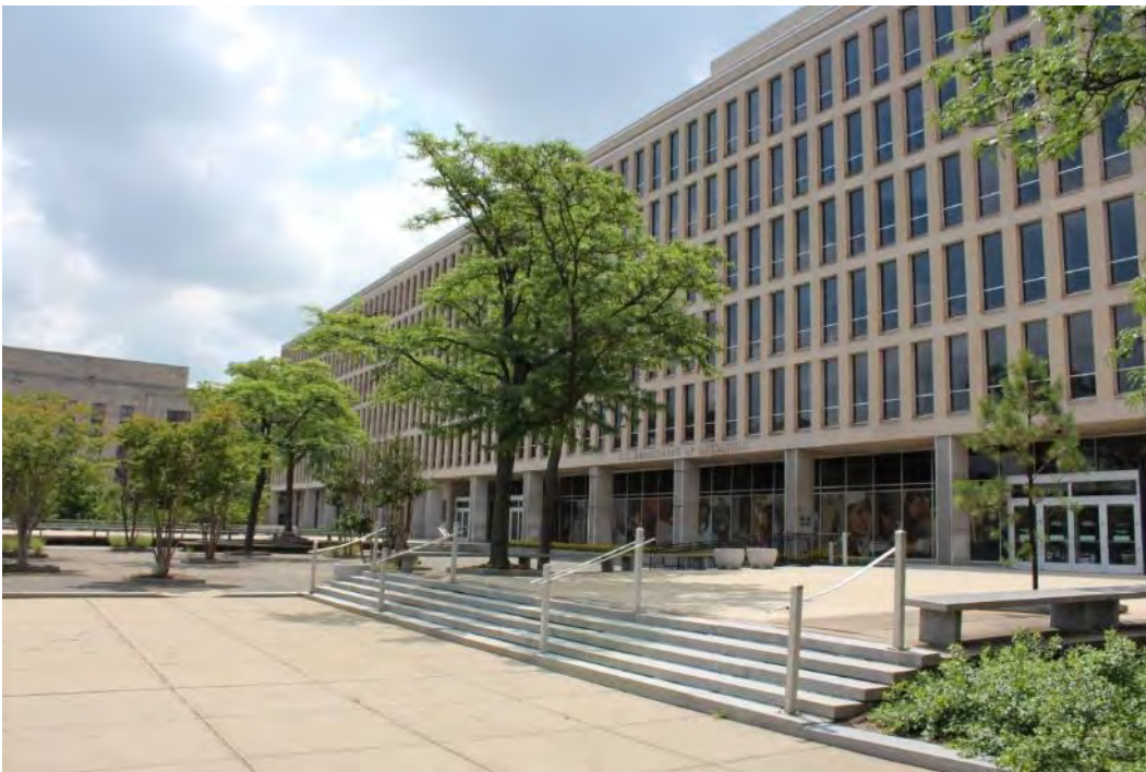
Photo #0003: DC_Federal Office Building No. 6_0003.tif Façade, western walkway and central terrace, facing southeast.
