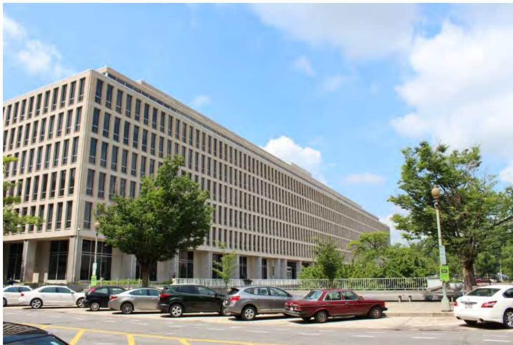
Photo #0001: DC_Federal Office Building No. 6_0001.tif Façade and east elevation, facing southwest.
