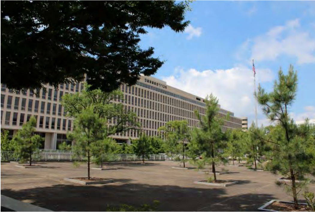
Photo #0006: DC_Federal Office Building No. 6_0006.tif East terrace and office building, facing southwest.
