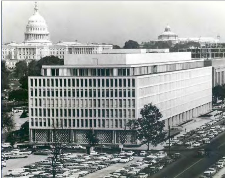
Figure 9: Historic Photograph, FOB 6, ca. 1961. Source: Suckow, Elizabeth and Chris Jedrey. NASA Hidden Headquarters , http://hqoperations.hq.nasa.gov/docs/Hidden_Headquarters_March_24_2009.pdf . Presentation given March 24, 2009.
