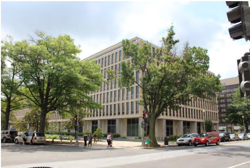
Photo #0012: DC_Federal Office Building No. 6_0012.tif Façade and triangular plaza along Maryland Avenue, S.W., facing southeast.
