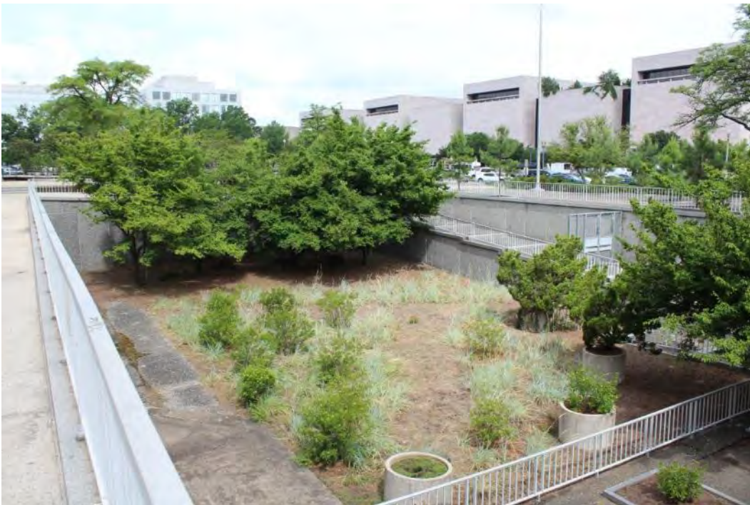
Photo #0007: DC_Federal Office Building No. 6_0007.tif Sunken courtyard, facing northwest.
