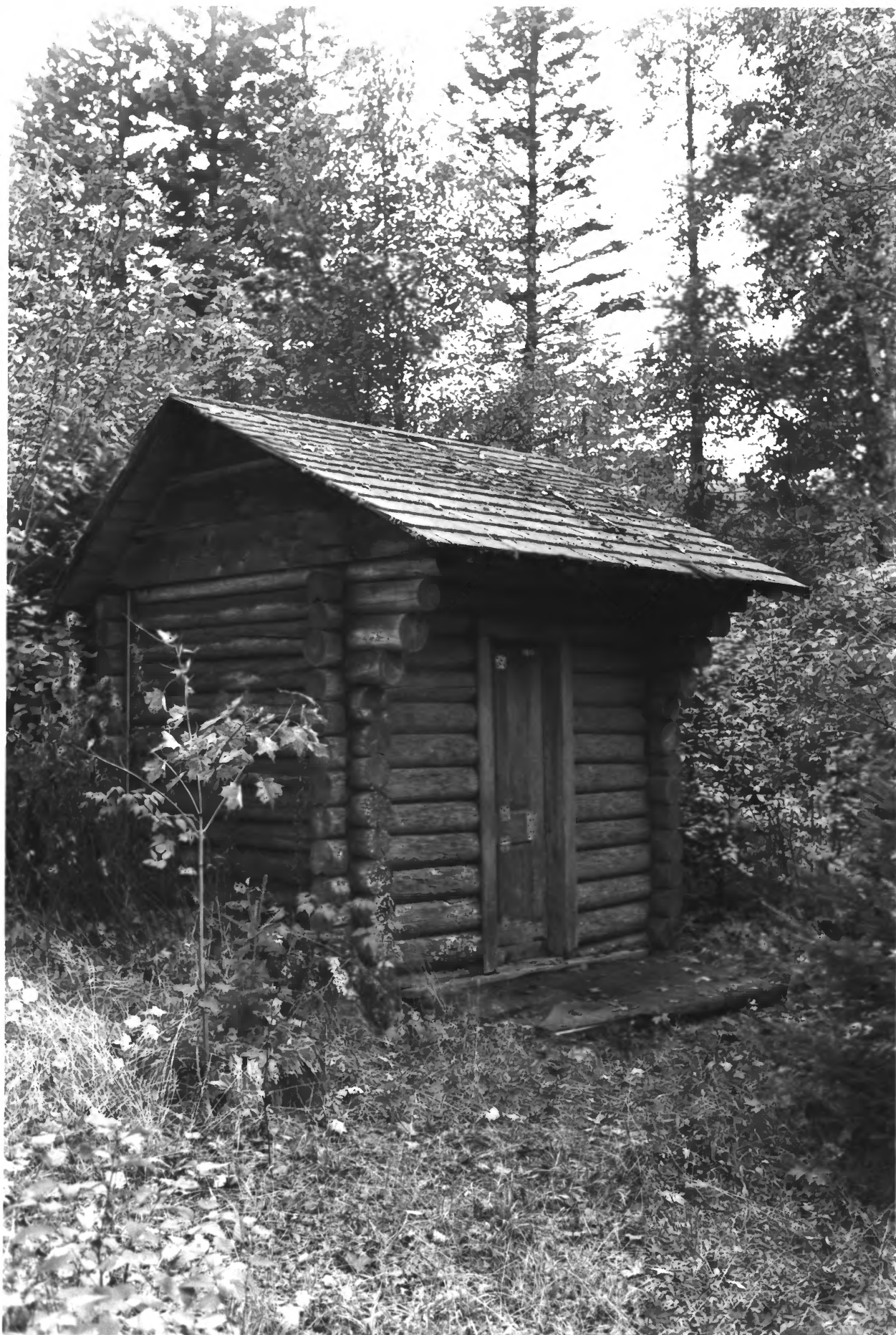
Outhouse, Teleguiche Camp Historic District (09331, 4A - photo #) Vicinity of Silver Bay, Lake Co., MN
