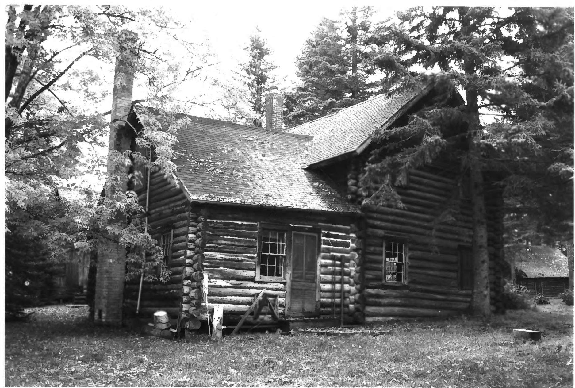
Tettegouche Camp Historic District Kitchen/Dining Hall, 1, (09331, # 0A-photo #) Vicinity of Silver Bay, Lake Co., MN
