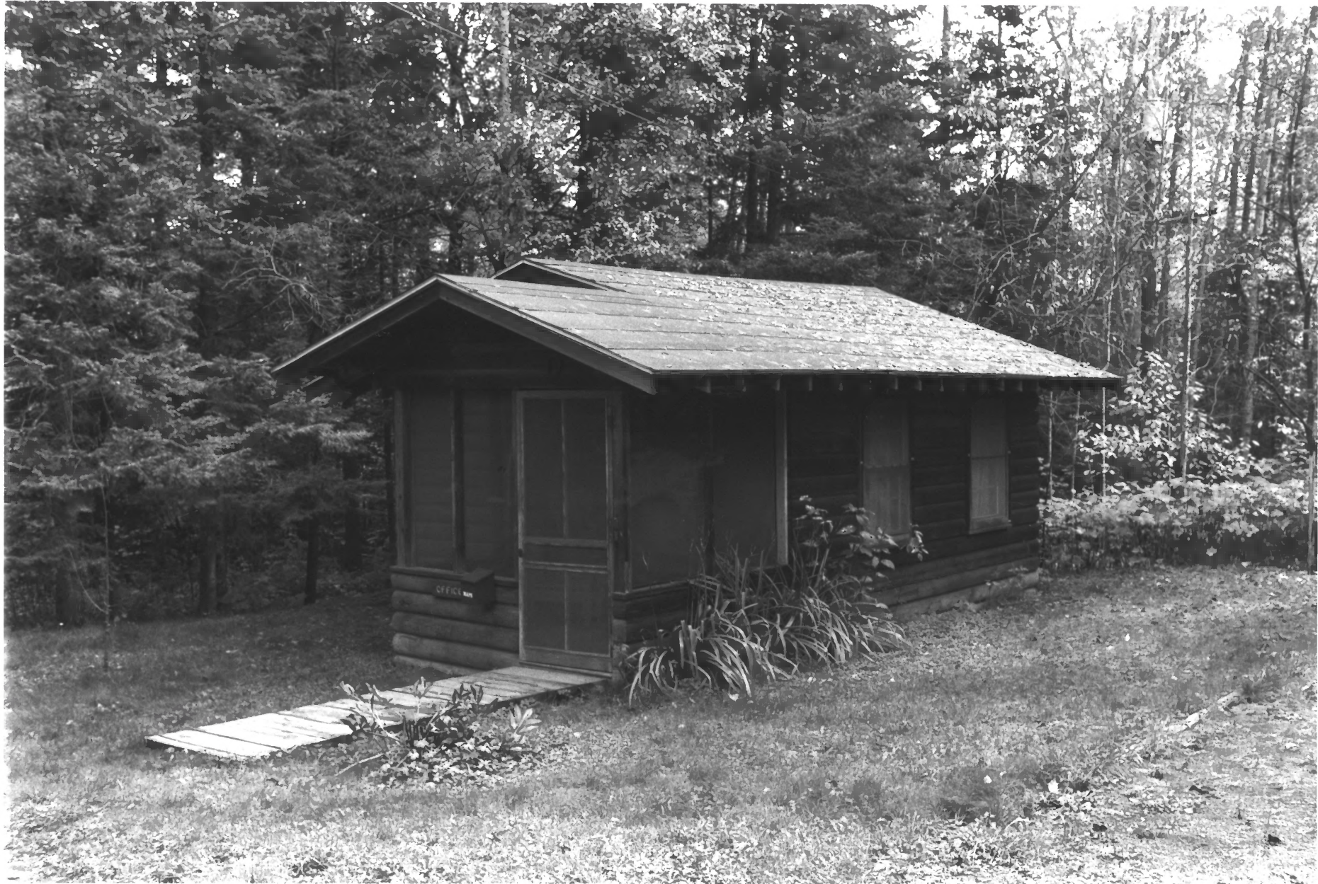
Cabin D, Tettegouche Camp Historic District (02391, #9 - photo #1) Vicinity of Silver Bay, Lake Co., MN
