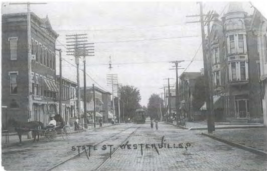
Figure 5: State Street, looking south from Main Street, c. 1907
