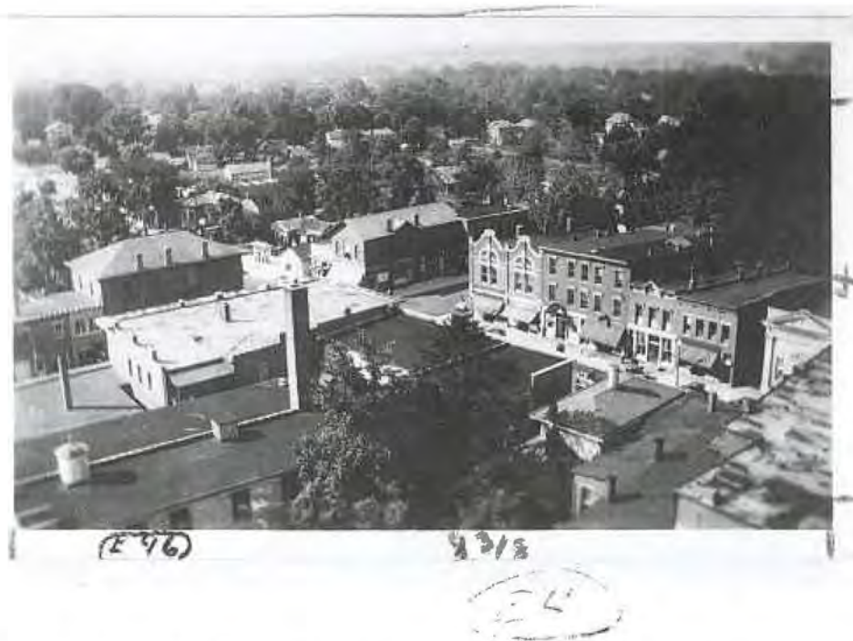
Figure 9: Bird's eye view of State Street, intersection with College Avenue, Looking southwest, 1930s
