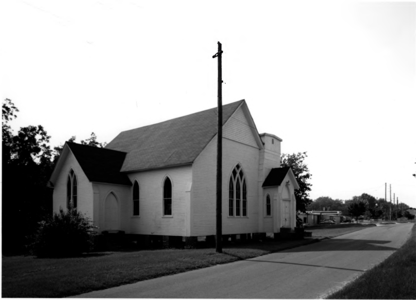
Haven Memorial Methodist Episcopal Church, Burke County, Georgia
