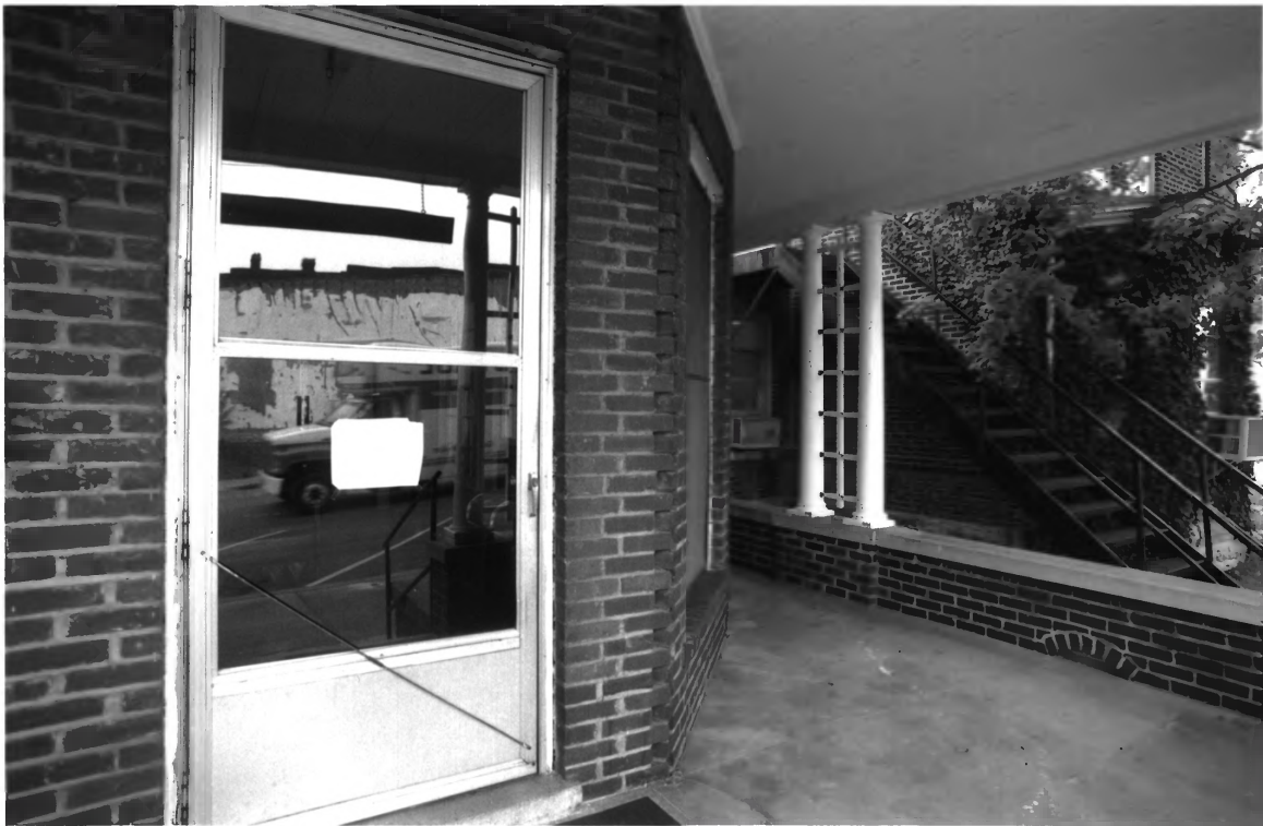
LADIES REST ROOM MARSHALL CO., TN # 2 of 15
