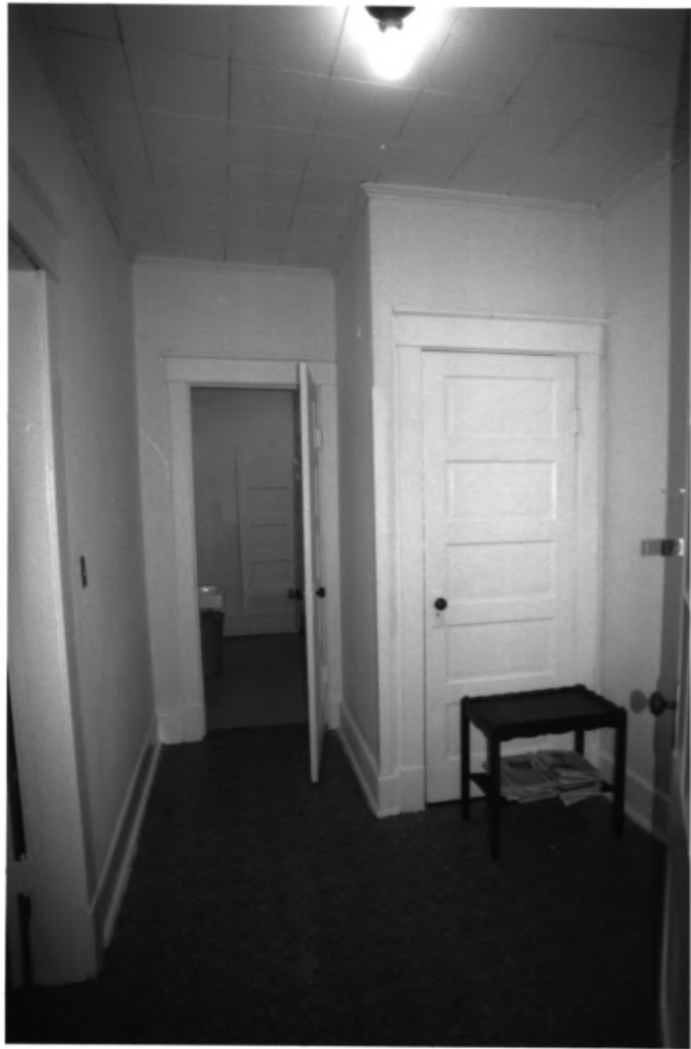
LADIES REST ROOM MARSHALL Co. TN #10 of 15
