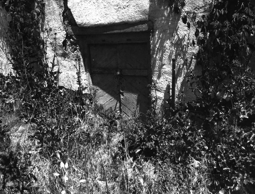
Malaguerra Winery Santa Clara County. Ca. Picture of a portion of the lower portion northerly end wall showing the access double doors. The picture shows the original stone and door beam. The plaster coat including the whitewash will be repaired in the rehabing to a Wine Museum. Picture taken 5/19/78 13 of 14
