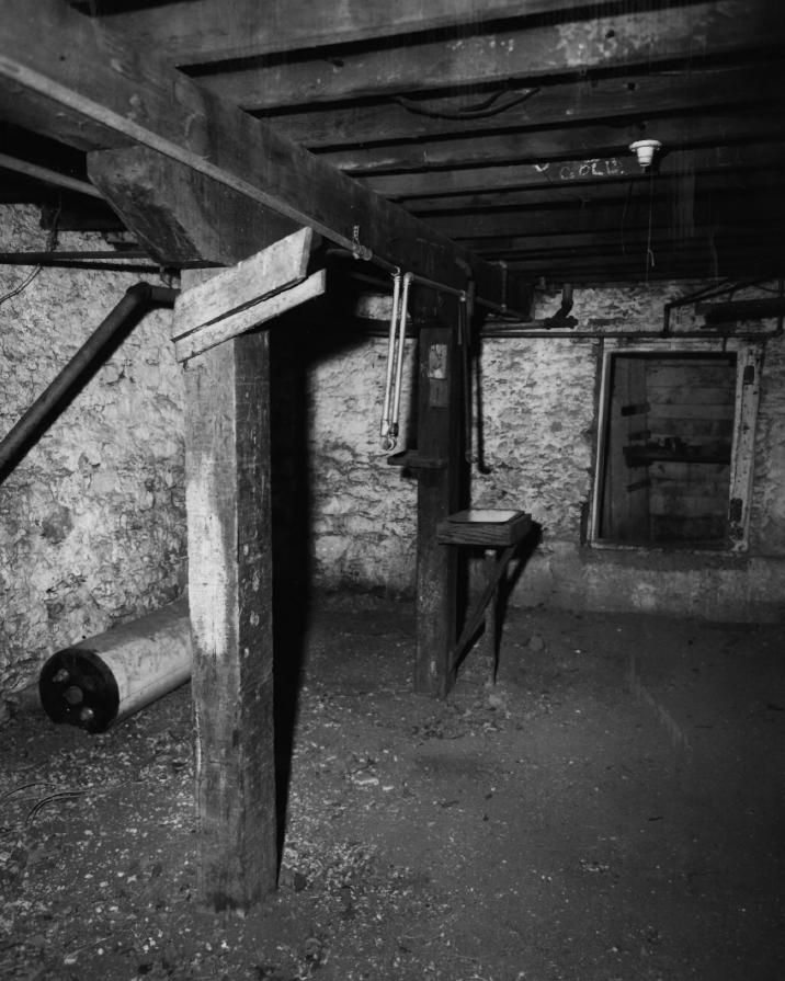
Malaguerra Winery UEC 7 Santa Clara County, Ca. Interior view of the basement or 1st floor, 1869 structure showing part of the easterly and southerly stone walls. It shows the heavy redwood posts, beams and joists. In rehabing the Winery, the exposed piping and wiring of added circa 1922 will be removed. Picture taken 5/19/78 10 of 14
