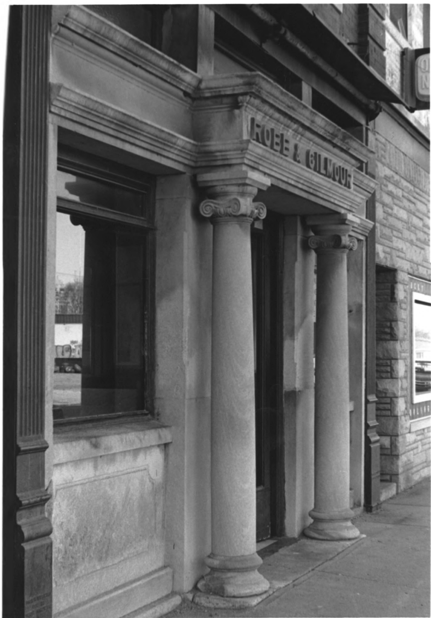
141 S. MAIN ST., CLINTON DOWNTOWN HIST. DIST., VERMILLION CO., IN PHOTO NO. 7
