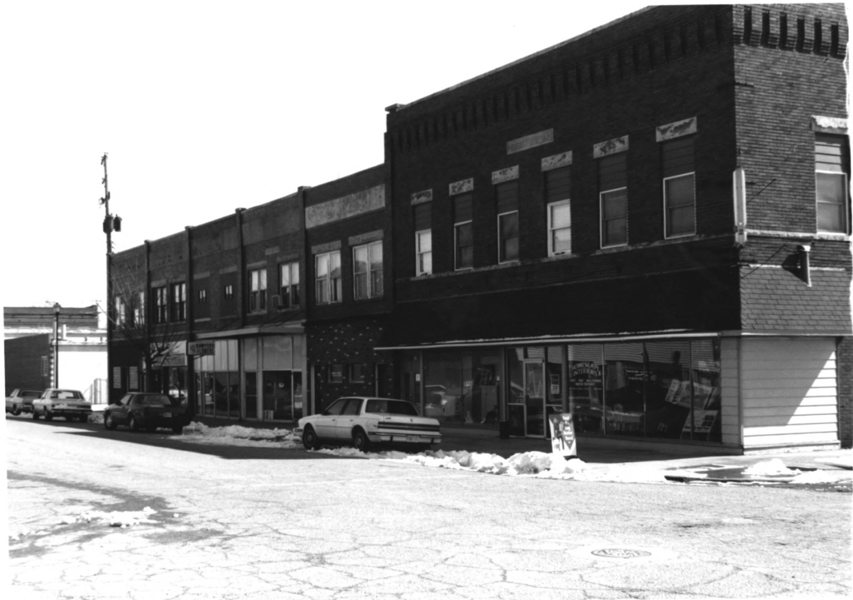
258-239 BLACKMAN ST., CLINTON DOWNTOWN HIST DIST., VERMILLION CO, IN, PHOTO No. 15
