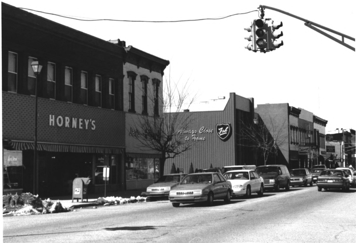
249-219 S. MAIN ST., CLINTON DOWNTOWN HIST. DIST., VERMILION CO., IN PHOTO No. 12
