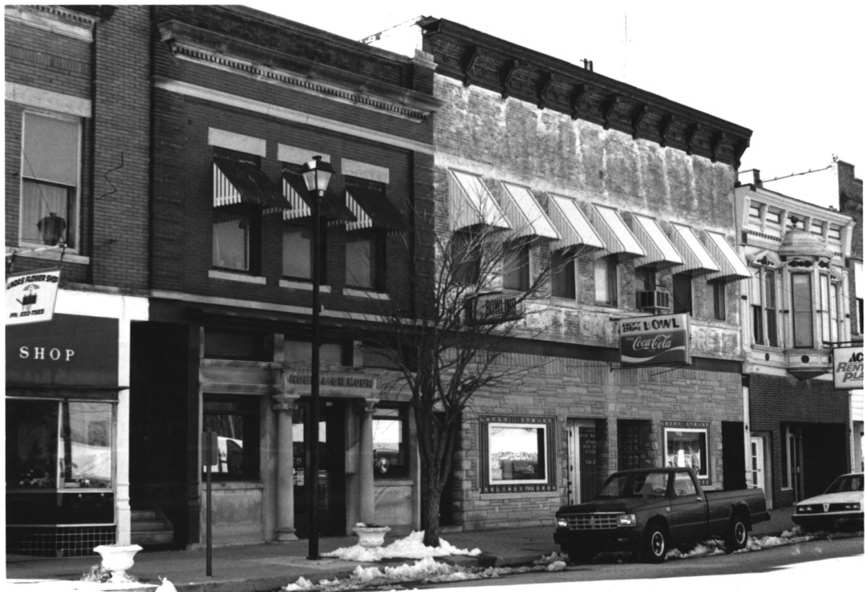
145-139 So. MAIN ST., CLINTON DOWNTOWN HIST. DIST., VERMILION CO., IN., PHOTO NO. 5
