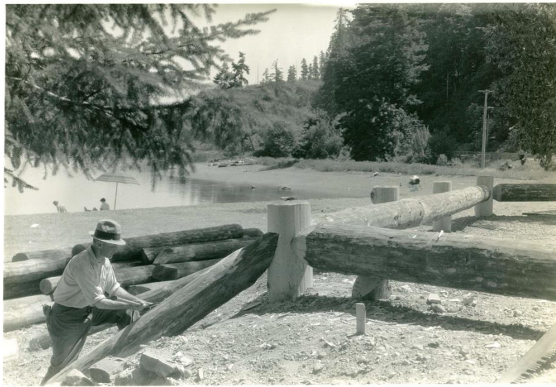
TSP14: Enrollee working on guard rails. Dan Sheehan, photographer. July, 1936
