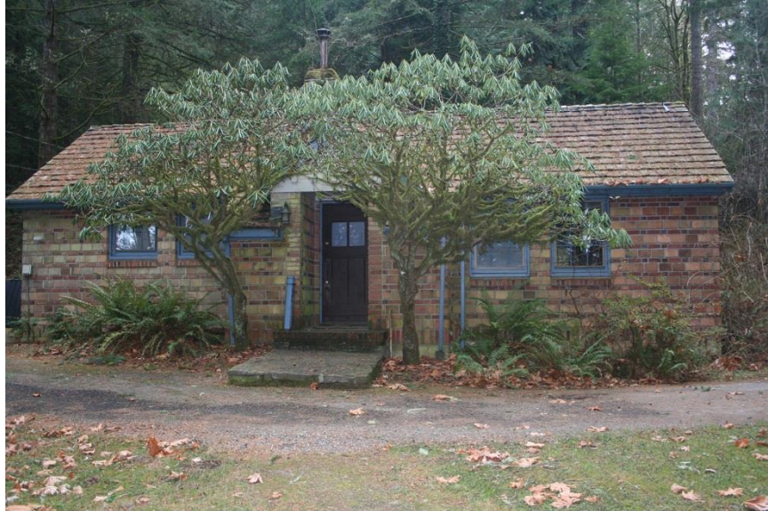
0037: Building 1 (superintendent's house), north (front) elevation, looking south.
