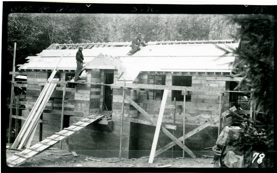
TSP19: Superintendent's house, under construction. Unknown photographer. Ca. 1936
