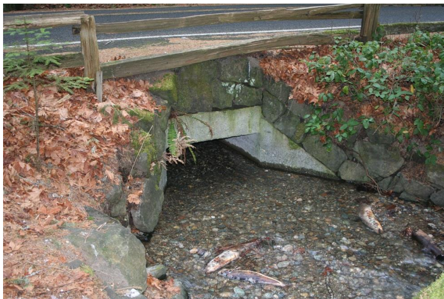
0028: Highway culvert, north elevation, looking southwest.
