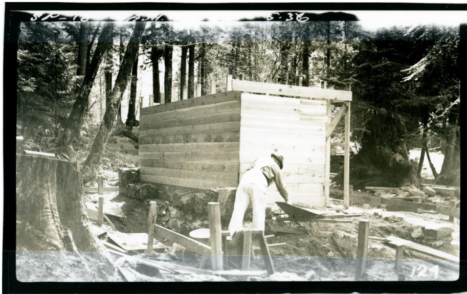
TSP6: Comfort station stone wall construction. Unknown photographer. Ca. 1936
