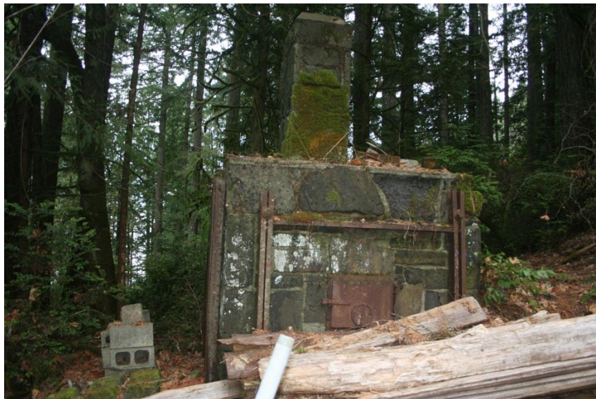
0044: Incinerator, west elevation, looking east.
