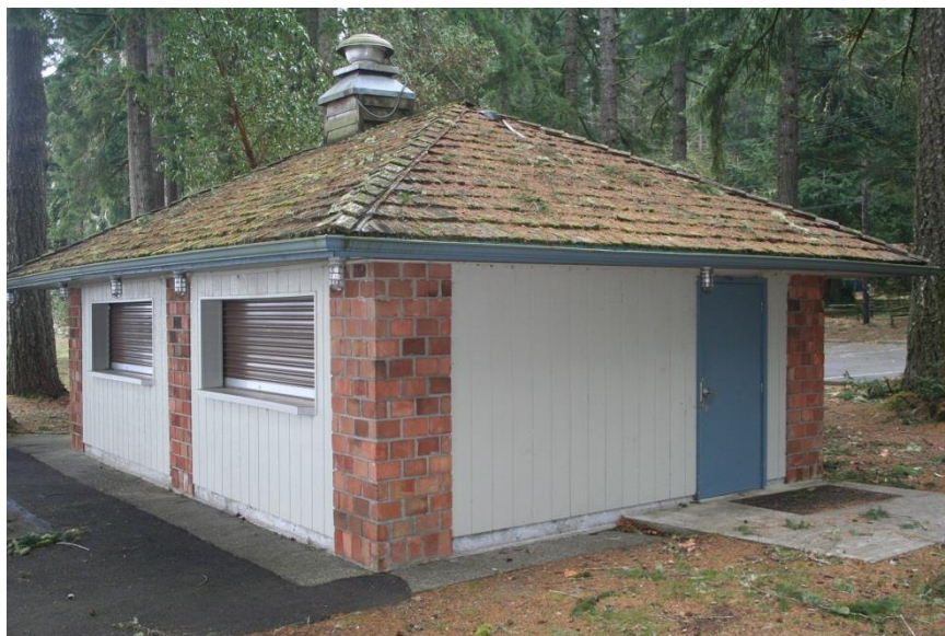
0020: Building 16 (concession), north and west elevations, looking southeast.
