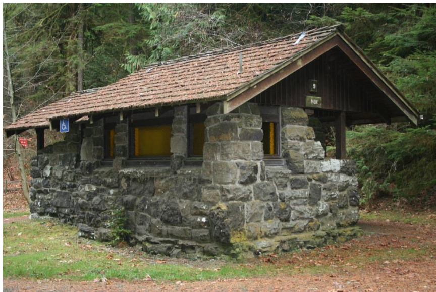
0030: Building 9 (comfort station #4), west and south elevations, looking northeast.
