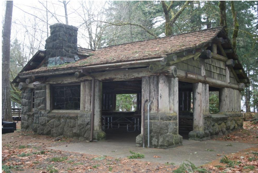
0007: Building 11 (shelter kitchen), southwest and southeast elevations, looking north.
