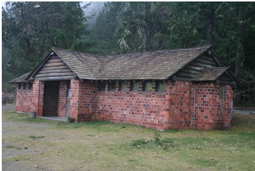
0024: Building 4 (bathhouse #1), north and west elevations, looking southeast.
