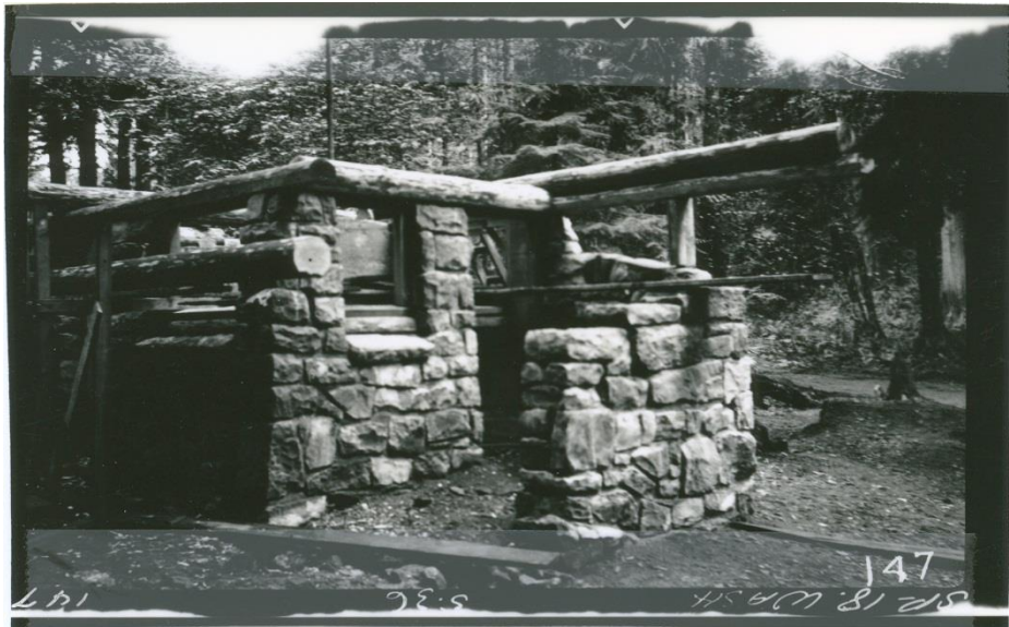
TSP10: Building 9 (comfort station #4) under construction. Unknown photographer. May, 1936
