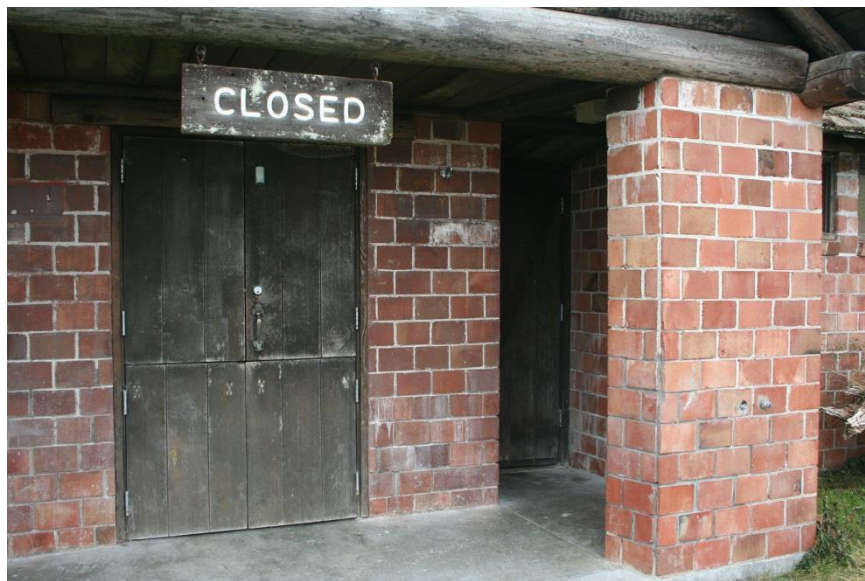
0022: Building 5 (bathhouse #2), entry detail, looking southwest.
