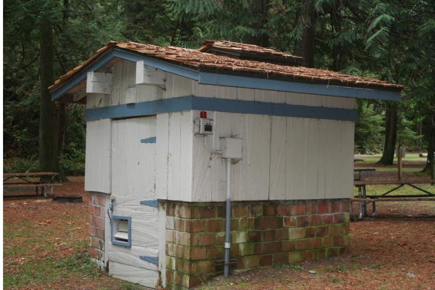
0029: Upper campground pump house, north and west elevations, looking southeast.
