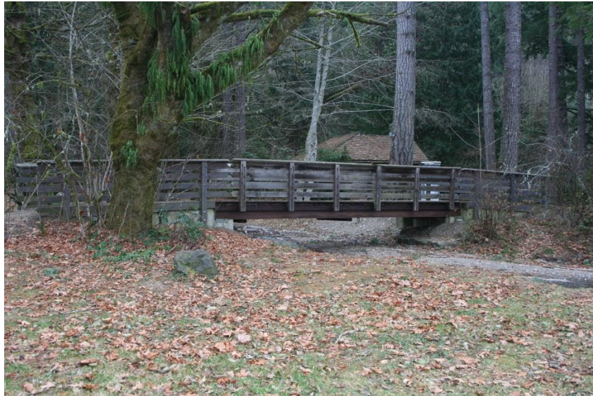
0005: Lower footbridge, north elevation, looking southwest.
