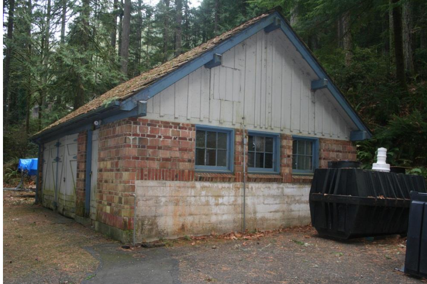
0041: Building 3 (garage/shop), west and north elevations, looking southeast.
