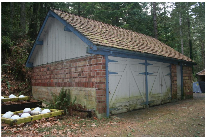
0042: Building 3 (garage/shop), north and east elevations, looking southwest.
