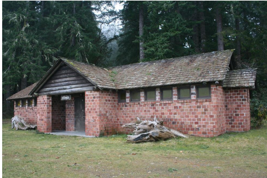
0021: Building 5 (bathhouse #2), north and west elevations, looking southeast.
