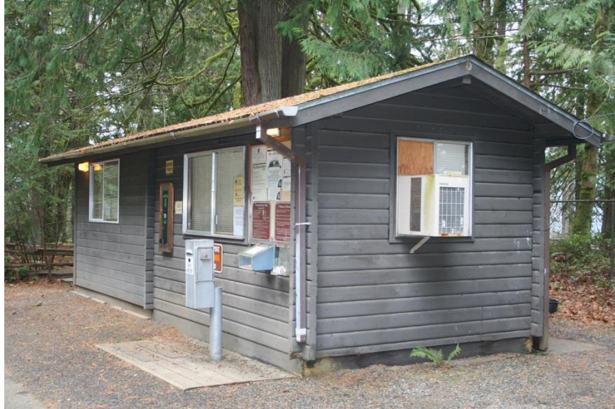
0027: Ranger's office, south and east elevations, looking northwest.
