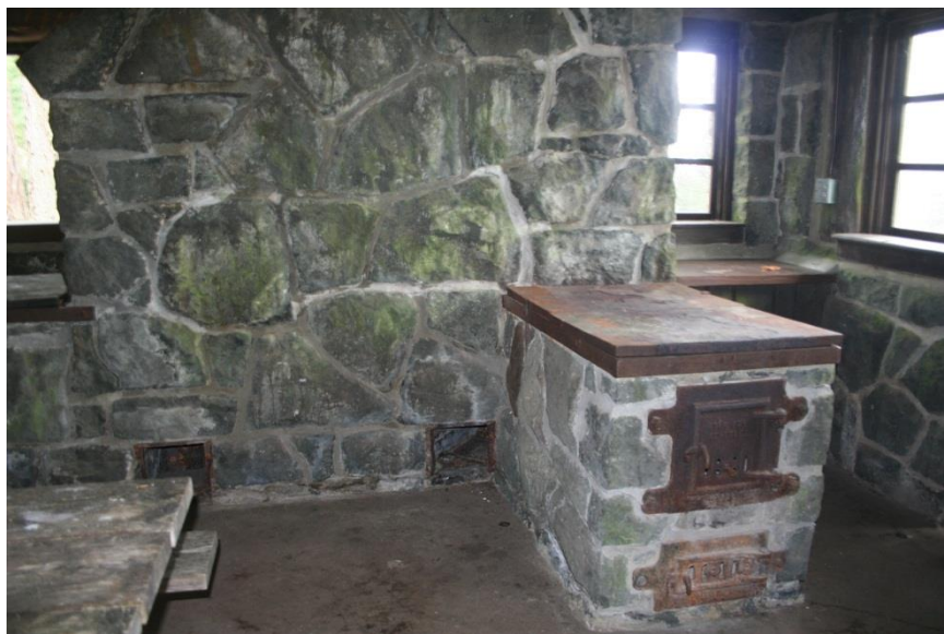
0008: Building 11 (shelter kitchen), interior, stove, looking north.
