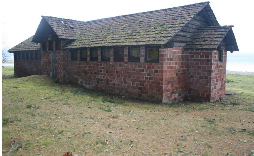
0023: Building 5 (bathhouse #2), south and east elevations, looking northwest.
