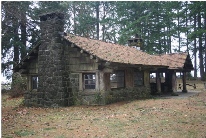
0012: Building 10 (community kitchen), south and west elevations, looking northeast.
