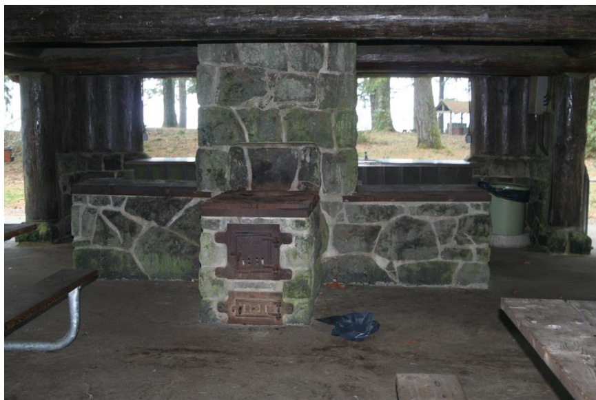
0014: Building 10 (community kitchen), interior, stoves, looking east.
