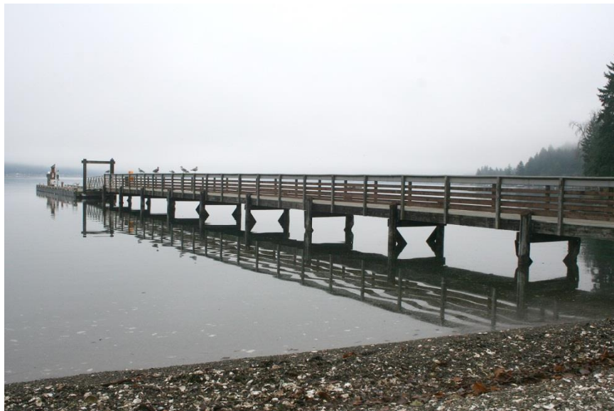
0026: Pier and dock, west elevation, looking northeast.
