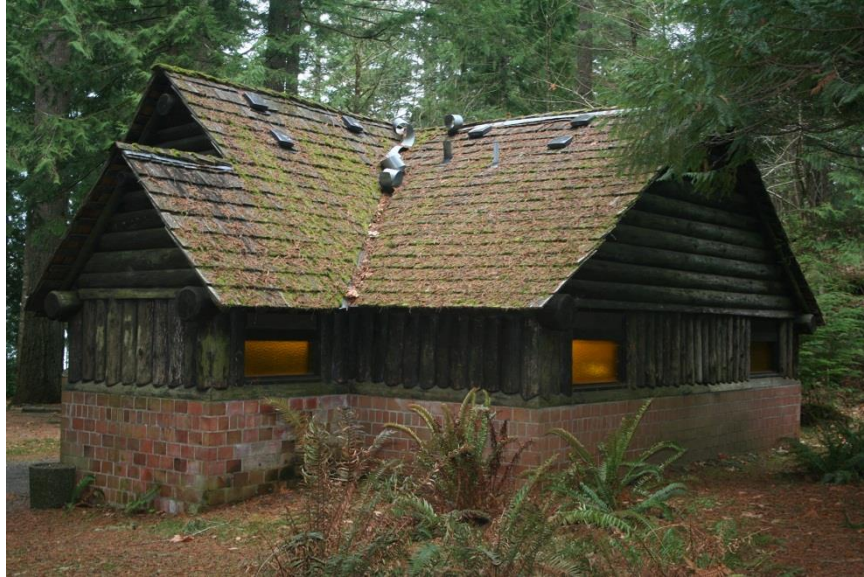
0035: Building 8 (comfort station #3), south and east elevations, looking northwest.
