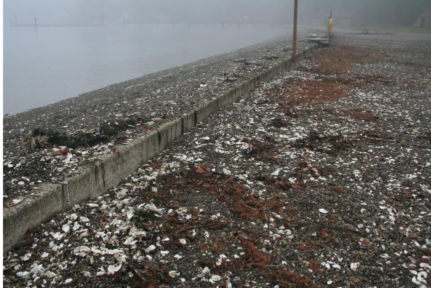
0017: Seawall, looking east.
