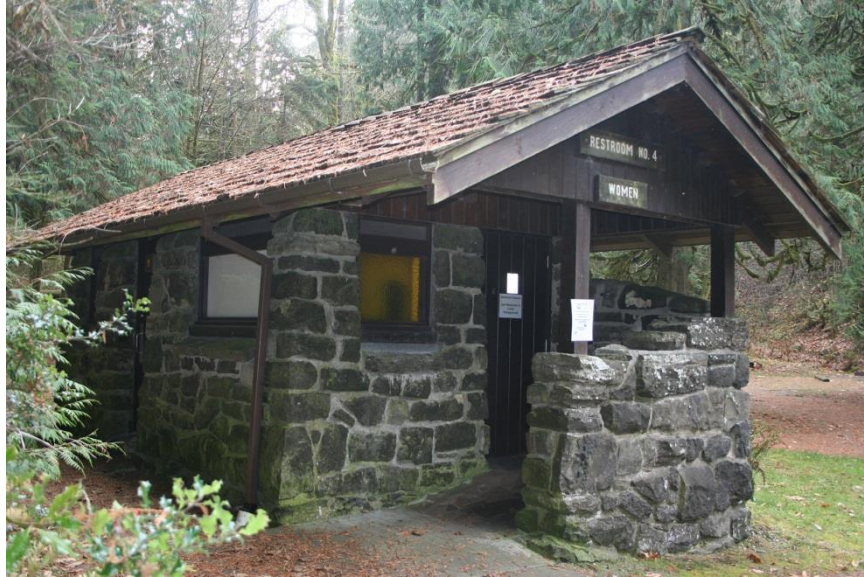
0031: Building 9 (comfort station #4), east and north elevations, looking southwest.
