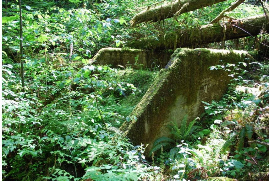
0033: Settling tank remnant, looking southeast.
