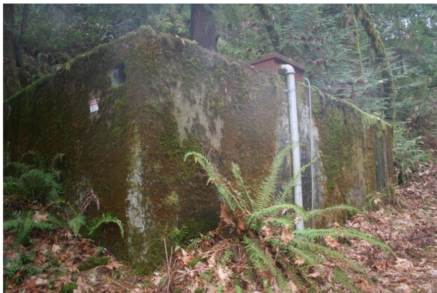
0032: Water storage reservoir, north and west elevations, looking southeast.
