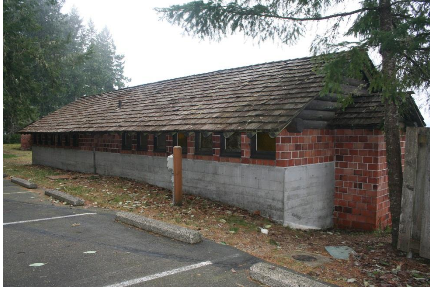
0025: Building 4 (bathhouse #1), south and east elevations, looking northwest.
