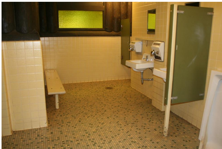
0036: Building 8 interior, looking southwest
