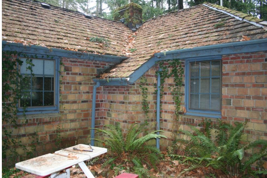
0039: Building 1 (superintendent's house), south and west elevations, looking northeast
