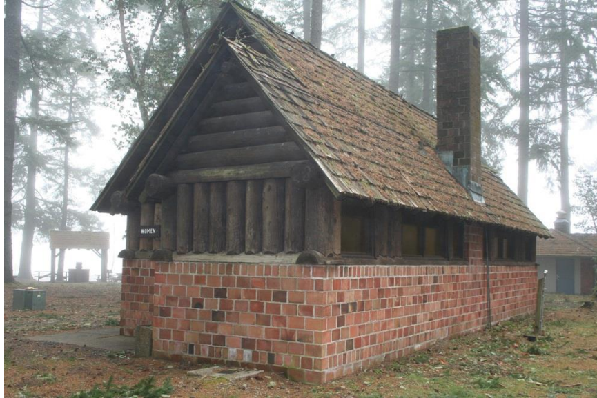
0015: Building 6 (comfort station #1), south and west elevations, looking northeast.
