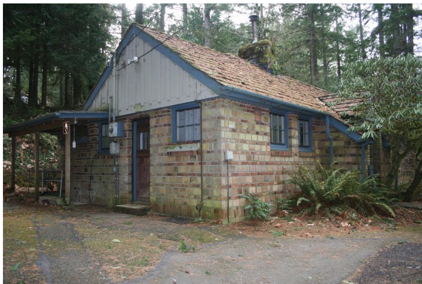
0038: Building 1 (superintendent's house), north and east elevations, looking southwest.
