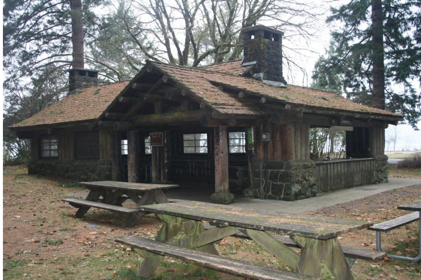
0011: Building 10 (community kitchen), south and east elevations, looking northwest.
