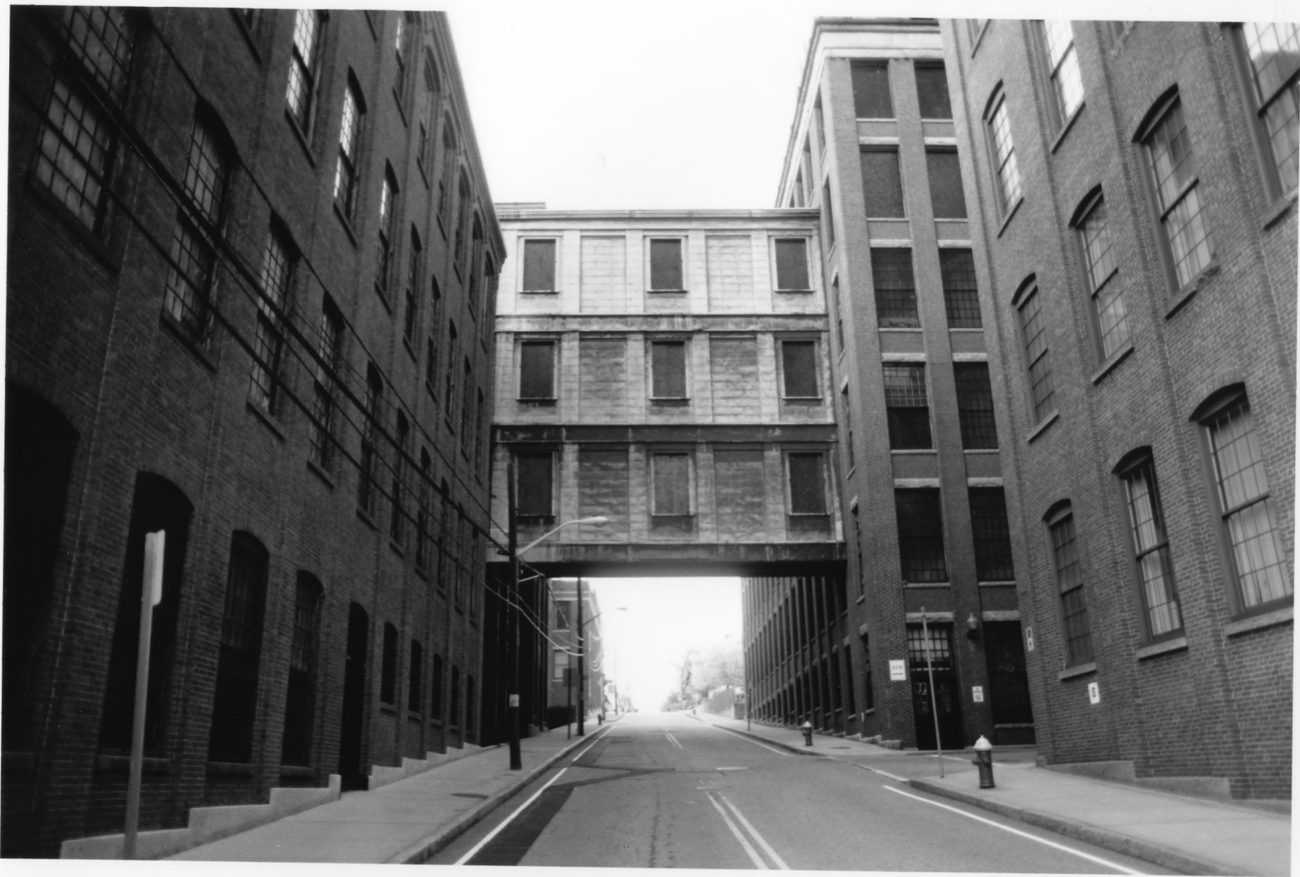
Brown & Sharpe Mfg. Co. Complex Providence County, Providence, RI photo # 5 of 16
