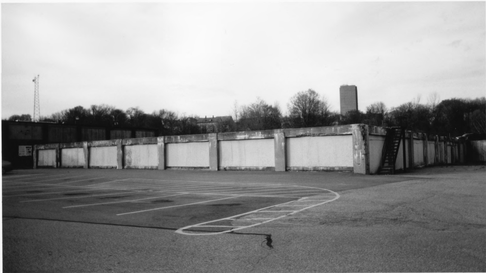
Brown + Sharpe mfg. Co. Complex Providence County, Providence, RI Photo # 8 of 16
