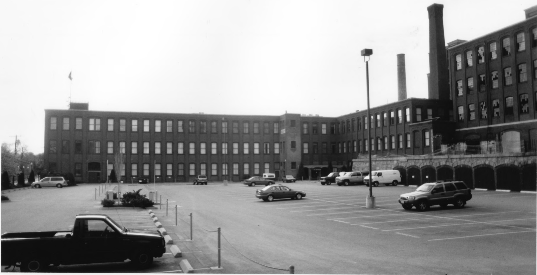
Brown & Sharpe Mfg. Co. Complex Providence County, Providence, RI Photo # 6 of 16
