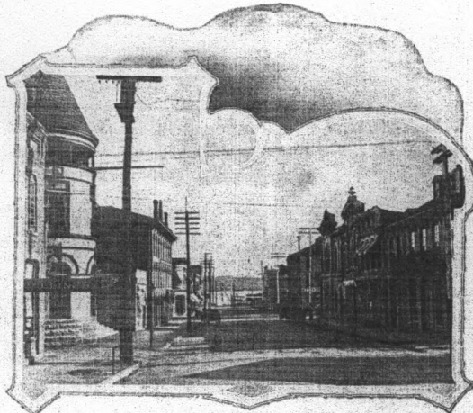
Pine Street, looking toward the Mississippi River
