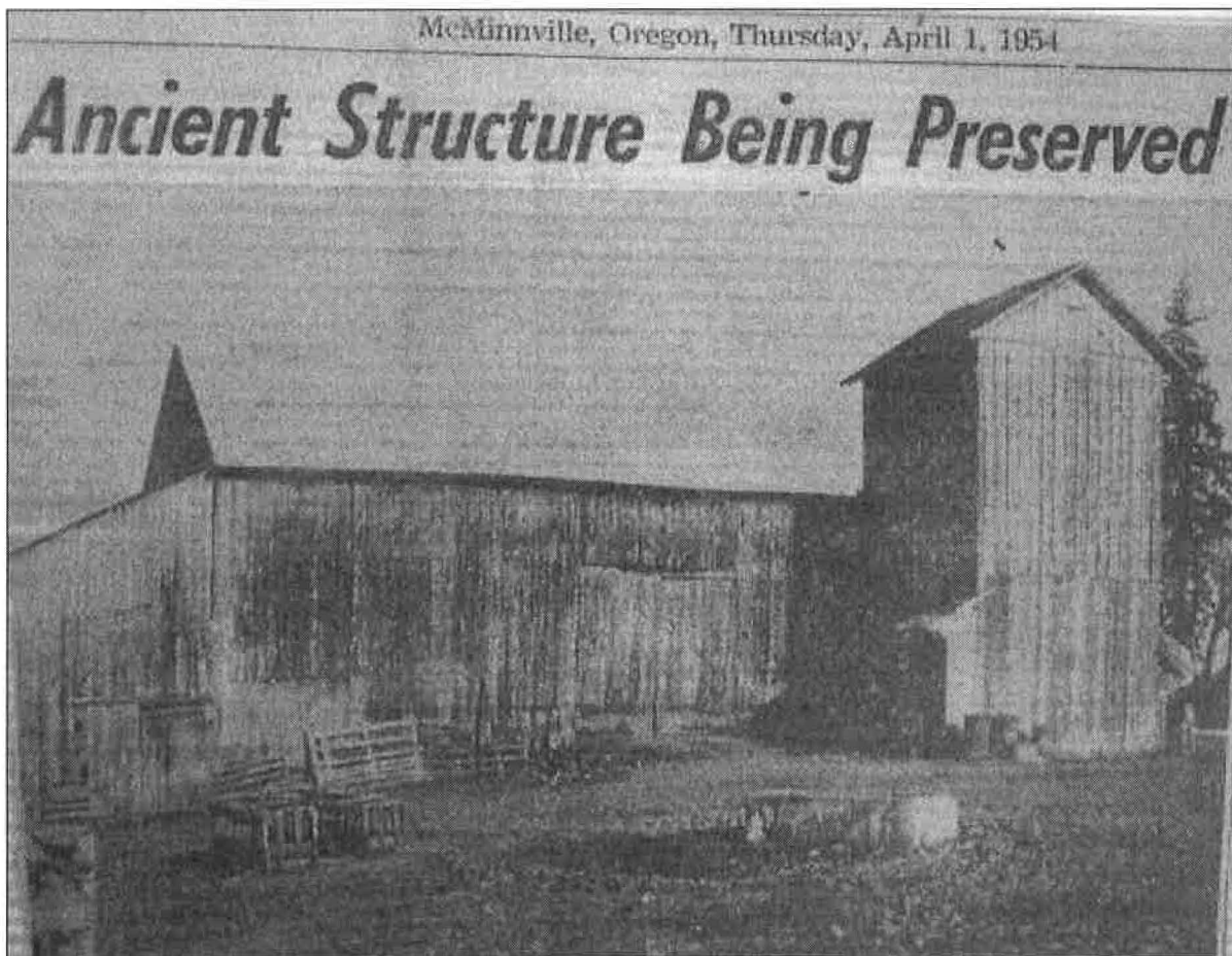
Figure 18: Barn and silo as pictured in 1954 McMinnville News article. Note house over silo (right) and north shed on barn (at left of picture). Courtesy Willamina Historical Museum.
