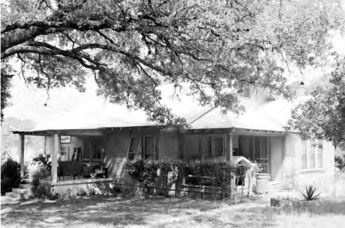
Figure 10 – Texas Historical Commission survey photo (c. 1975) of the 1930 bungalow residence/office. Courtesy Portal to Texas History, University of North Texas, THC Historic Resources Survey Collection.
