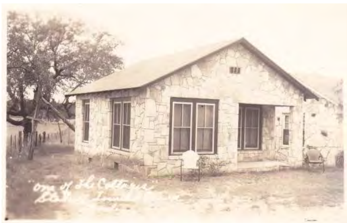
Figure 15 – Historic post card of Cabin #6 at River Oaks Courts. Courtesy Ople Stokes Boyle.
