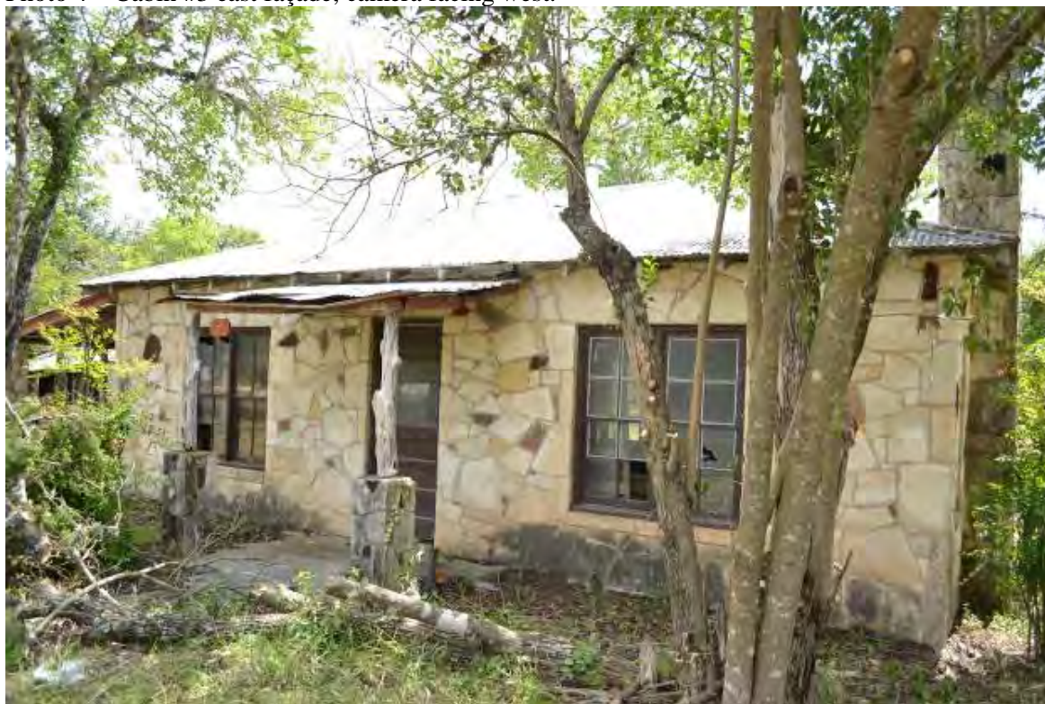
Photo 4 – Cabin #3 east façade, camera facing west.
