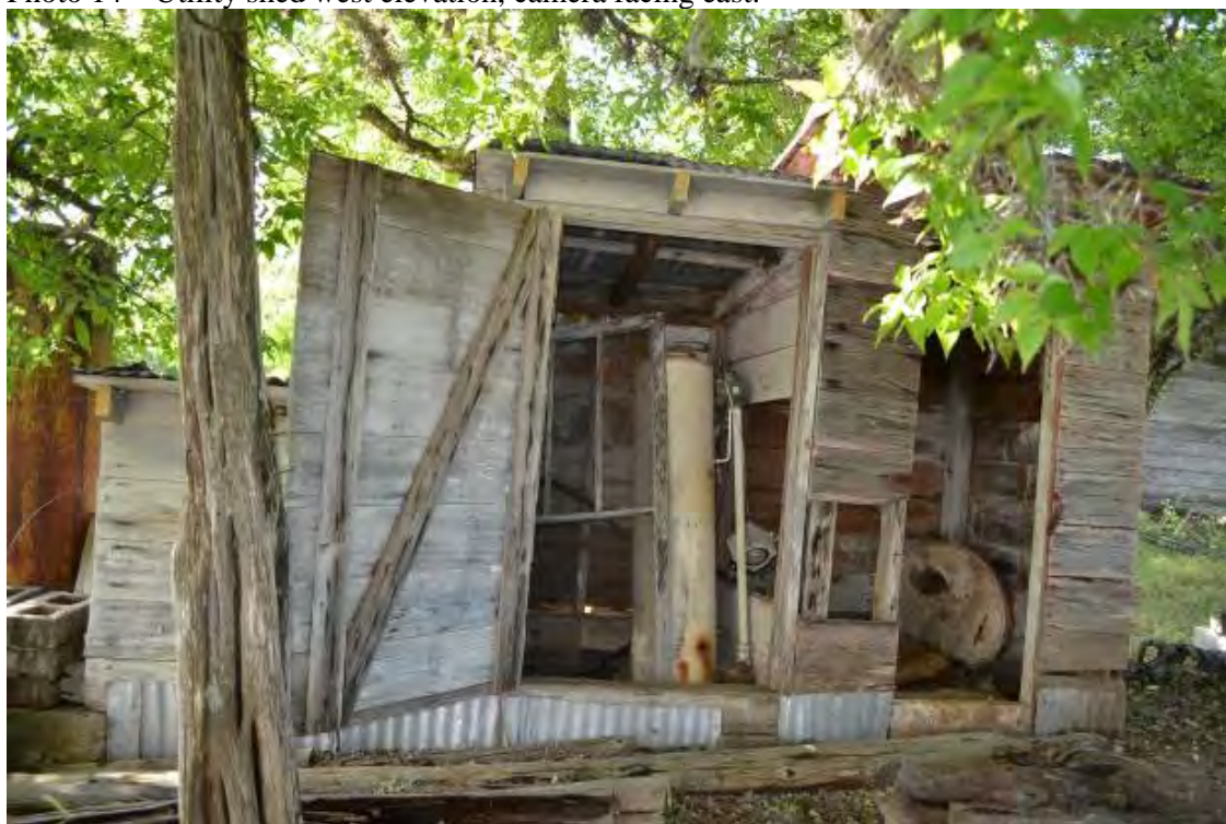
Photo 14 – Utility shed west elevation, camera facing east.
