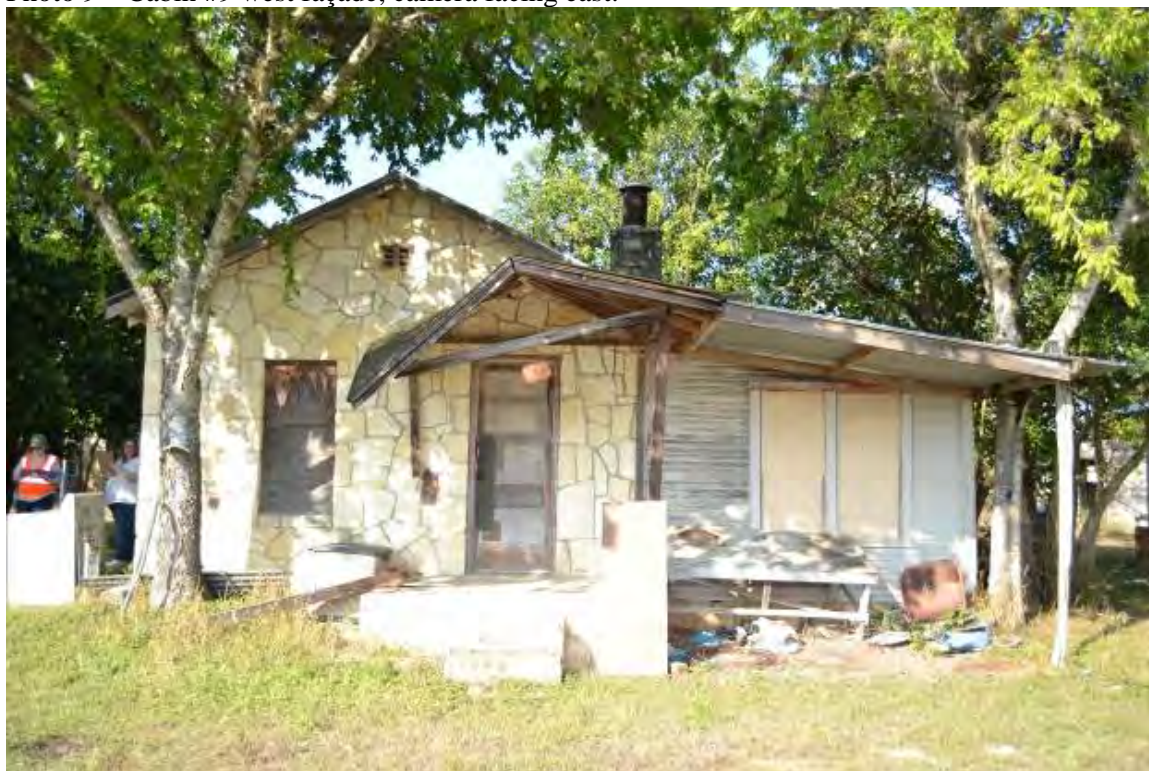
Photo 9 – Cabin #9 west façade, camera facing east.
