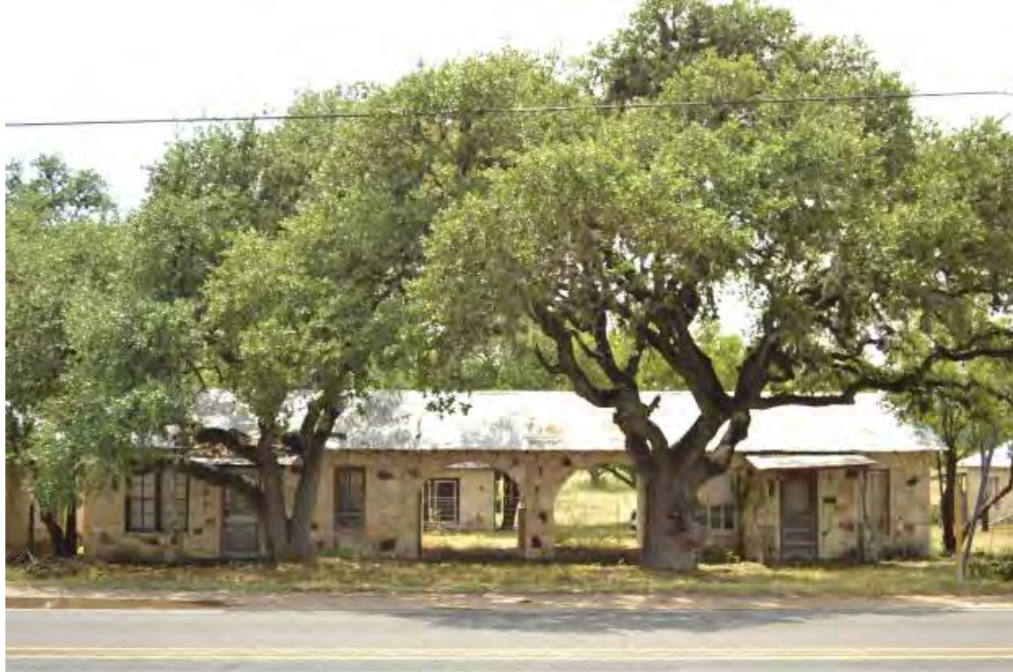
Photo 5 – Cabins #4 and #5 east façades with arched carports, camera facing west.
