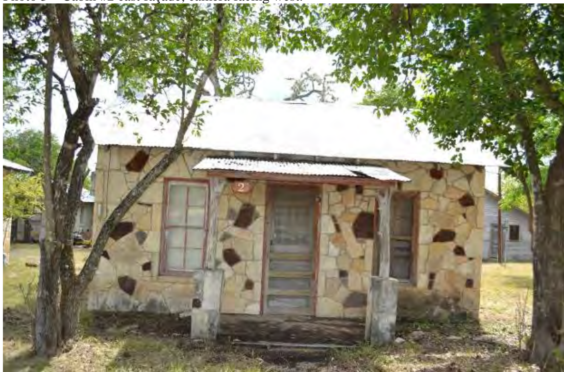
Photo 3 – Cabin #2 east façade, camera facing west.
