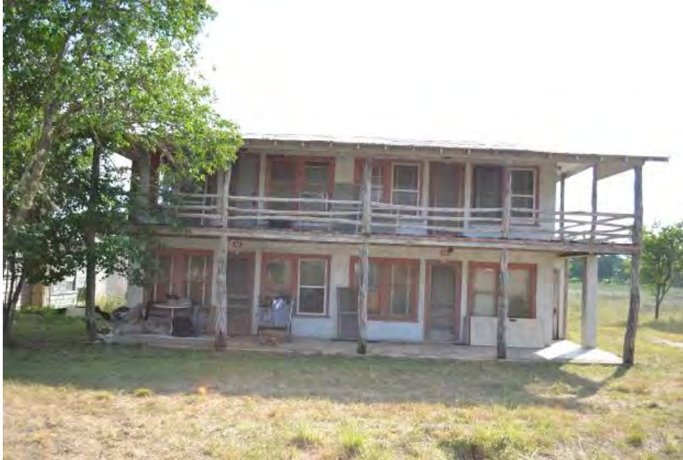
Photo 11 – 1945 Fourplex (units #11-14) east façade, camera facing west.
