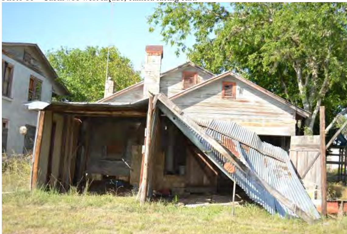
Photo 10 – Cabin #10 west façade, camera facing east.
