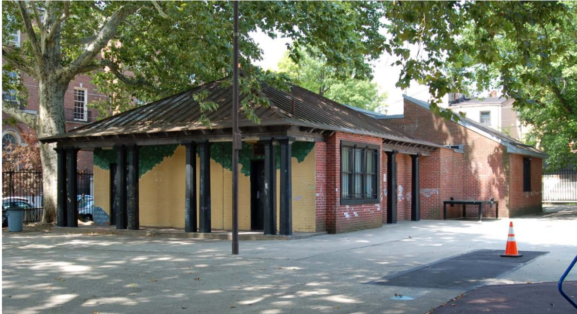
Current Photo 3: The Recreation Building, facing Southwest, which was constructed over the burial ground. The 1924 building includes a late 1970s addition on the west side. The patch of dark pavement with the orange cone in the right side of the image is the location of one of the 2013 trenches investigated to establish the location of the original burial ground wall. See Figure 25.
