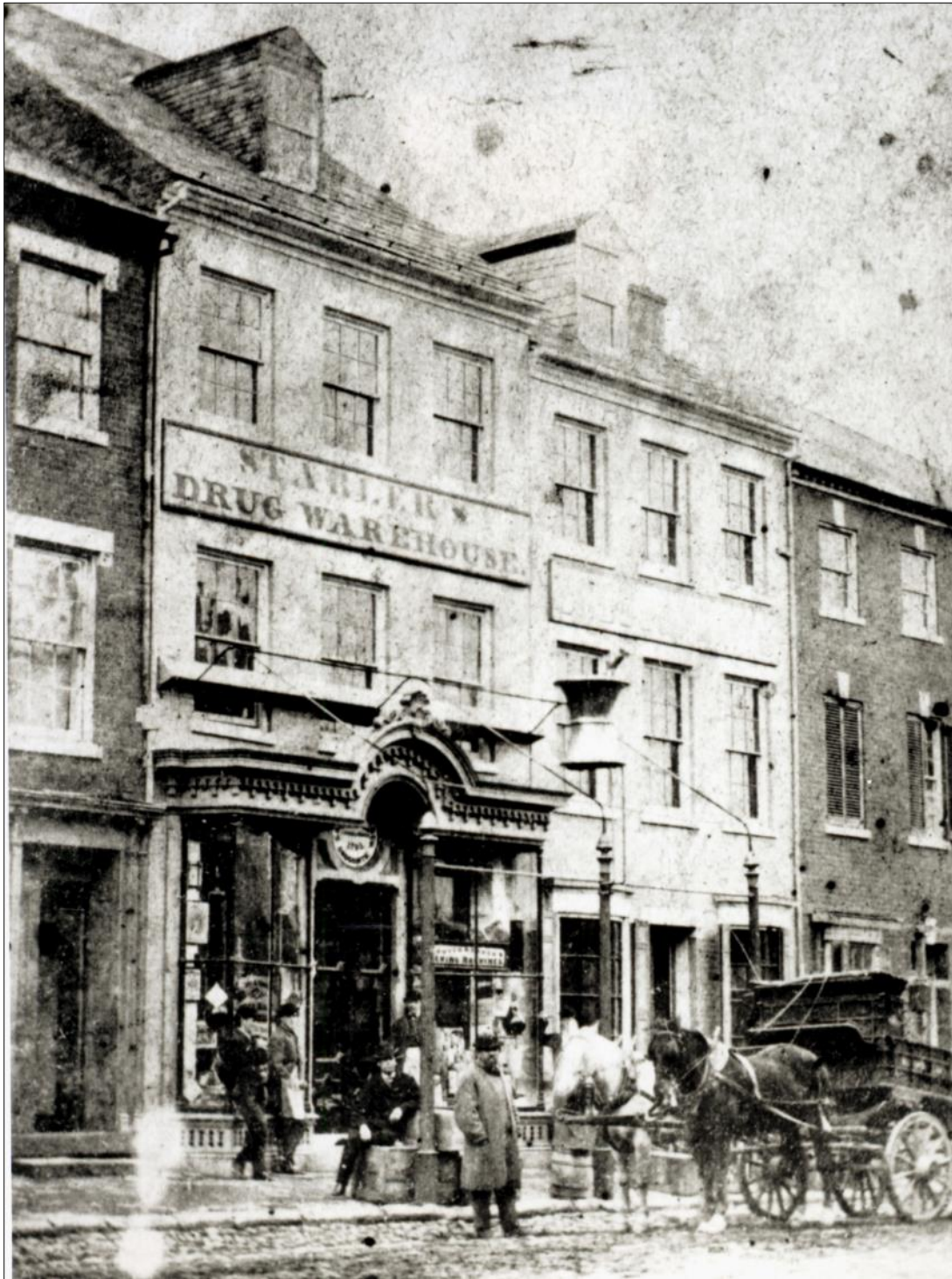
Figure 1. STABLER-LEADBEATER APOTHECARY SHOP, Alexandria, Virginia Italianate storefront on 107 S. Fairfax Street (left) and Federal storefront on 105 S. Fairfax Street (right). circa 1870
