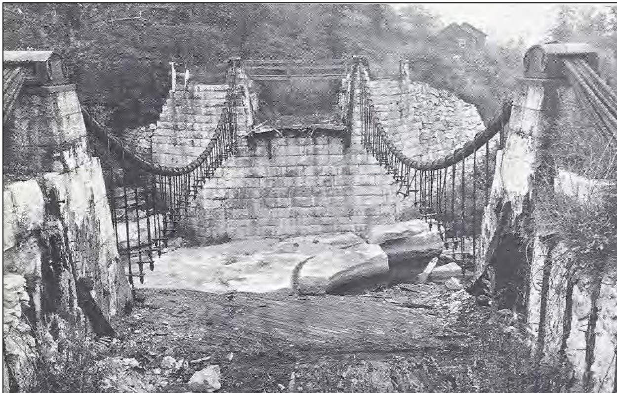
Fig.9: Historic view of suspension structure of the aqueduct that crossed the Rondout Creek in High Falls after a fire burned the wood trough. Although shorter, the Peterskill aqueduct in Alligerville would have been constructed in the same manner. Both were designed by John A. Roebling along with two others on the canal's route. From Wakefield, Coal Boats to Tidewater , 212.
