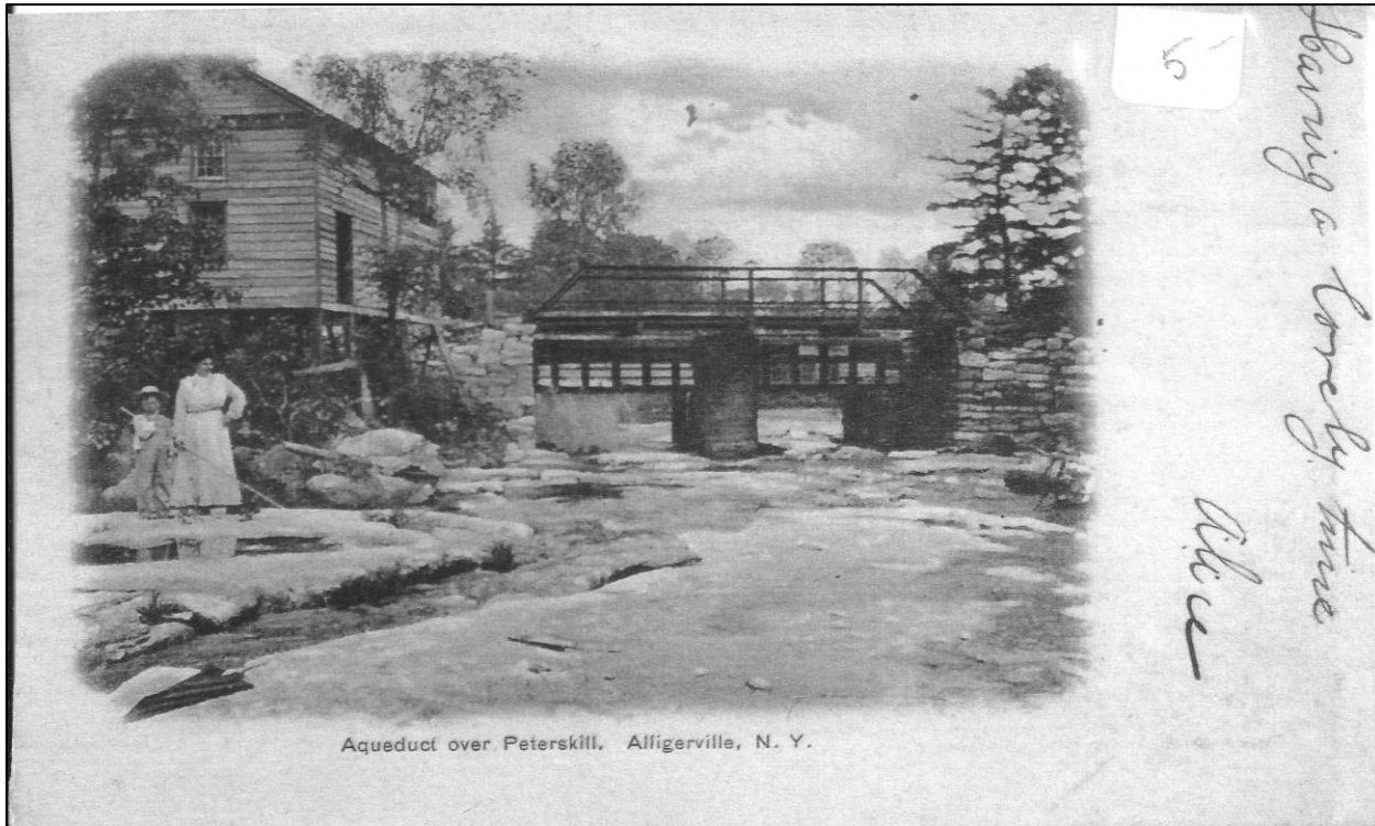
Fig.8: Post card view of Peterskill aqueduct and Peter B. Davis's mill, ca. 1910. Note that the wood trough carrying the canal still existed under the metal truss bridge built for Tow Path Rd. when the canal ceased operation. Collection of Delaware & Hudson Canal Historical Society, High Falls, NY.
