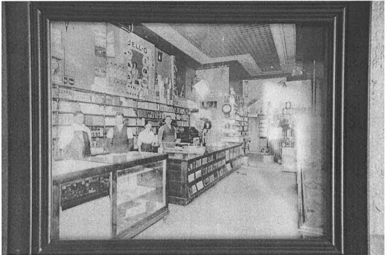
Figure #2: Interior View, date unknown
