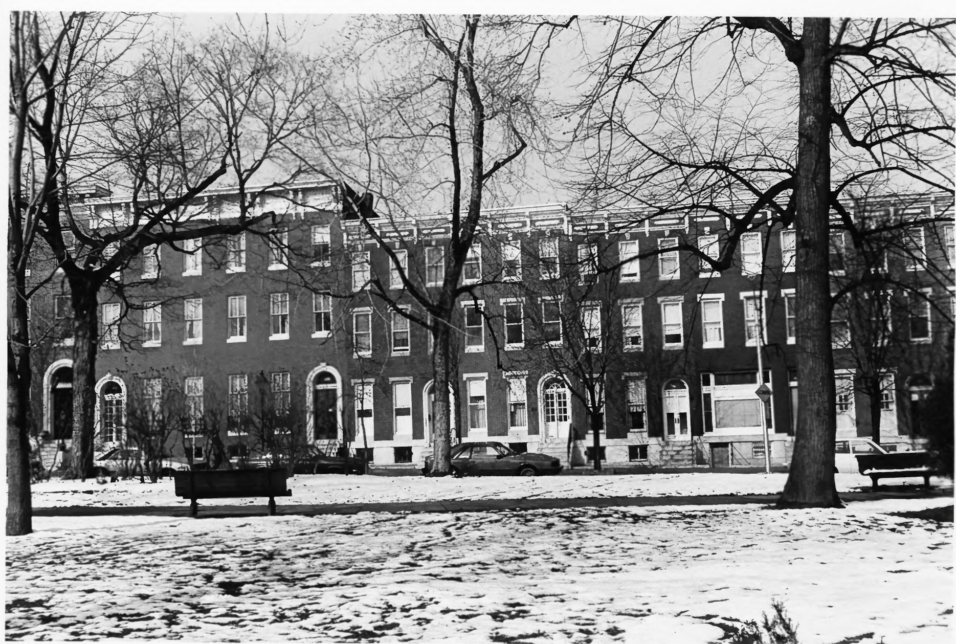
4/20 View of 1500 block of Hollins Street from Union Square with Mencken House in center of photograph
