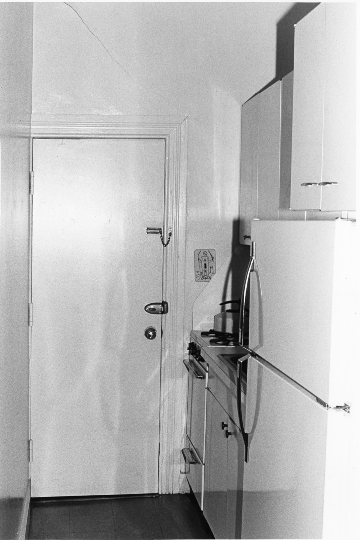
16/20 Interior, third floor, view of kitchen installed in el of front room, doorway leads into stair hall, partition on left was added when the kitchen was installed
