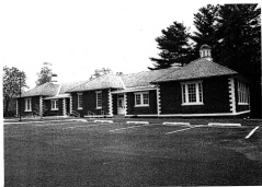
Court Street School, Freehold (1921)
