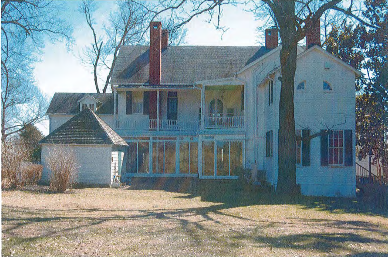
MD_FrederickCounty_Oakland_0002.tif Rear of house, camera facing south
